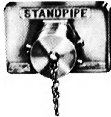
standpipe connection
