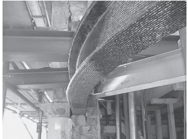
Fig. 43.8 The upgrading of a curved steel structural beam by the carbon fibre/epoxy composite low-temperature mould prepreg (Courtesy of Taylor Woodrow, UK, and ACG Derbyshire, UK).
