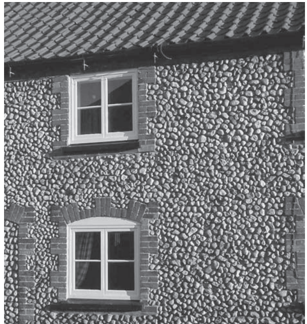
Fig. 37.7 Well-conserved flint-work masonry in Norfolk.
