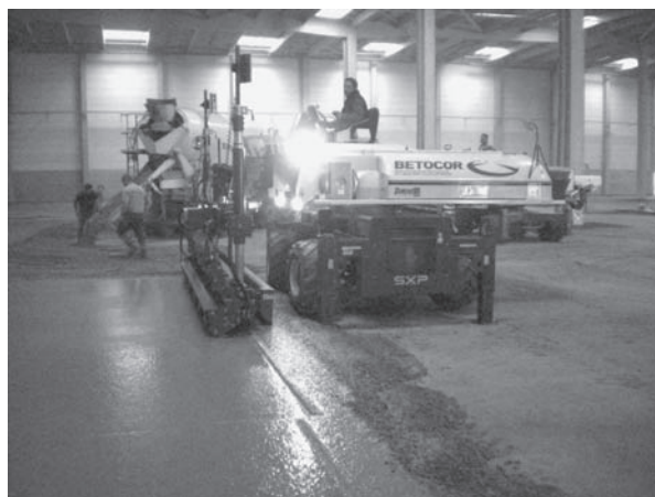
Fig. 50.4 Steel–FRC floor installation. (Supplied by J. Greenhalgh, Bekaert Ltd, UK ( www.bekaert.com )).
