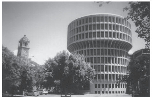
Fig. 50.1 Newcastle Council Chambers, Newcastle, Australia. (Photo by Kate Farquharson, Australia (2008), reproduced from flickr.com/photos/zigwamp under Attribution-No Derivative Works 2.0 Generic License (see creativecommons.org for license details).)
