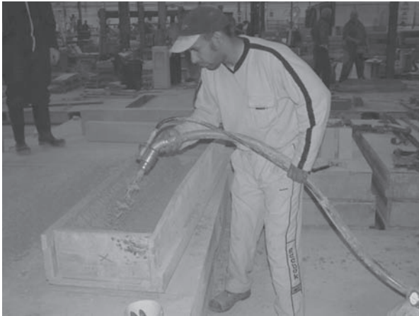
Fig. 49.2 Spraying of premix glass-FRC. (Supplied by Iain D. Peter, Powersprays Ltd., UK ( www.power-sprays.co.uk ).)
