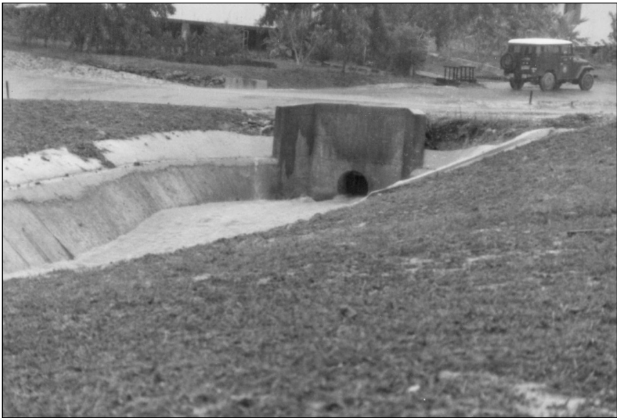
Figure A.2 Water canal–drainage system outlet under roadway.
