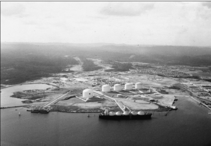
Figure A.1 Aerial view of a liquefied natural gas plant.
