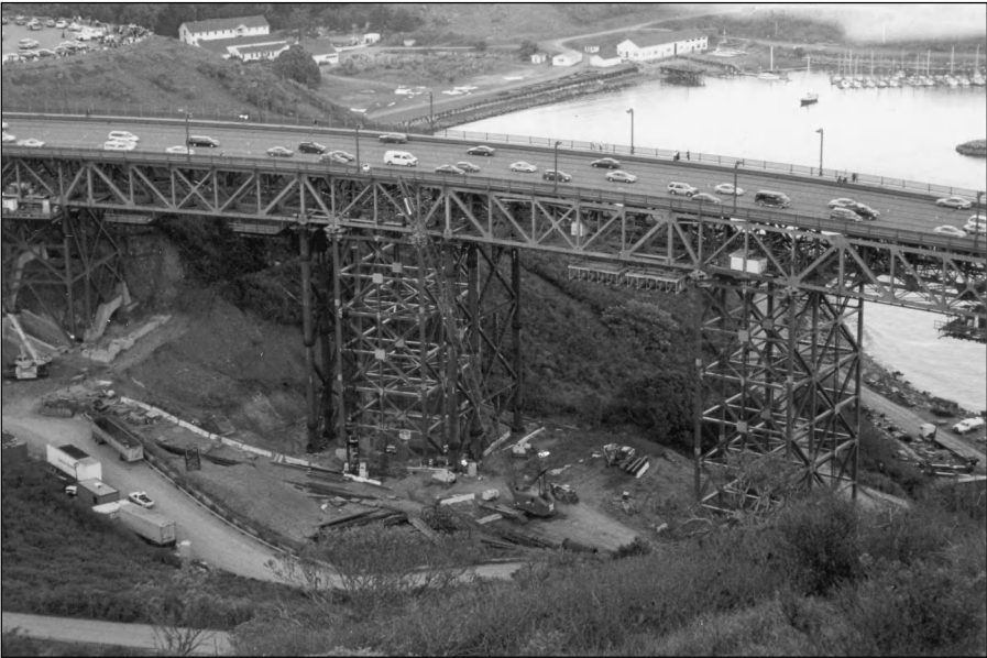
Figure 1.6 Golden Gate Bridge retrofit project, San Francisco, California.
