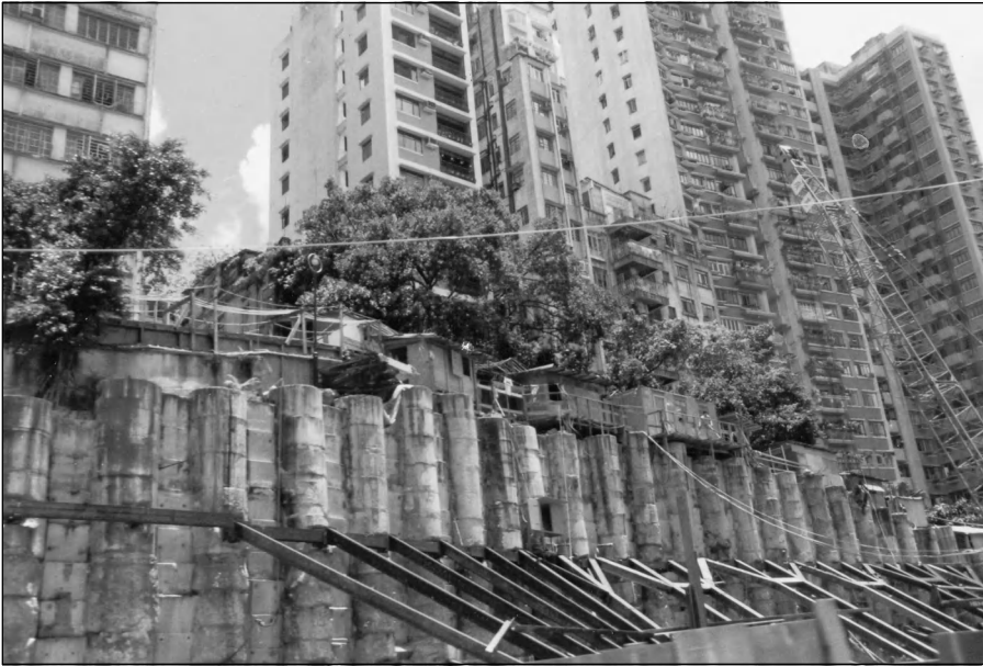
Figure 1.3 Construction of a retaining wall, Hong Kong.
