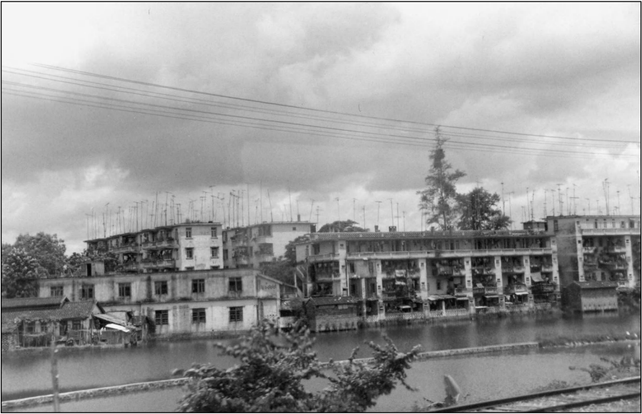
Figure 13.1 Antennas for television reception, China.
