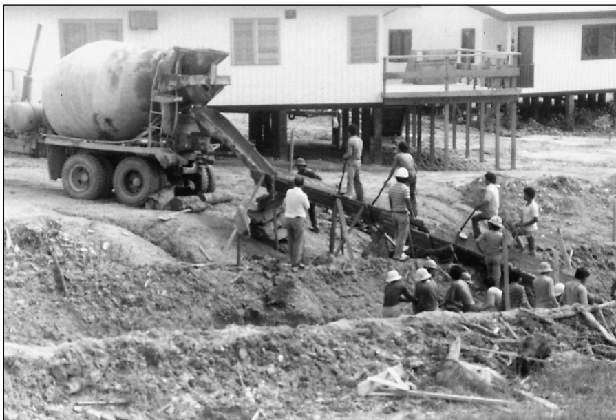
Figure A.4 Concrete pumping operation (chute supported by rocks and lumber).
