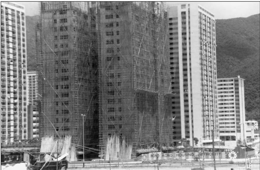
Figure 3.6 Bamboo scaffolding, China.
