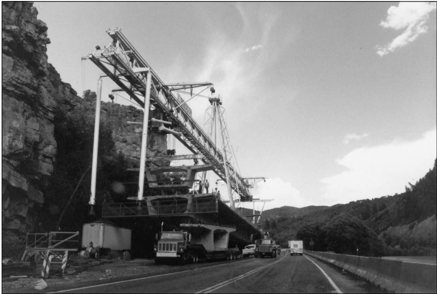
Figure 1.7 Gantry lifting a roadway section, Bear Creek, Colorado.
