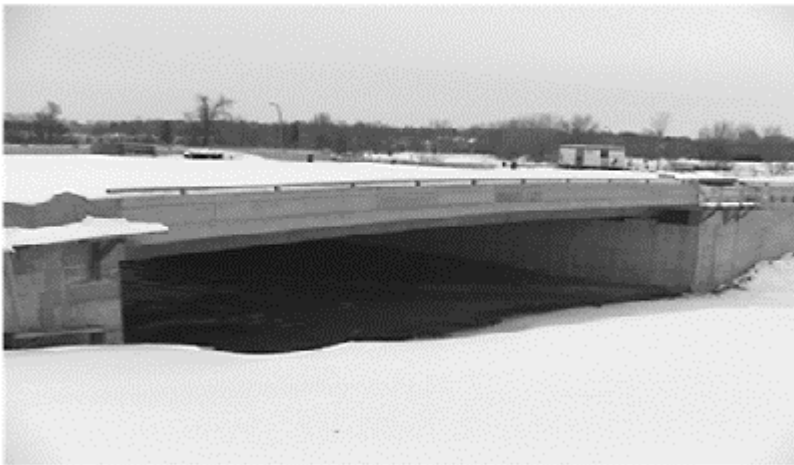
Figure 9. King Edward overpass.
