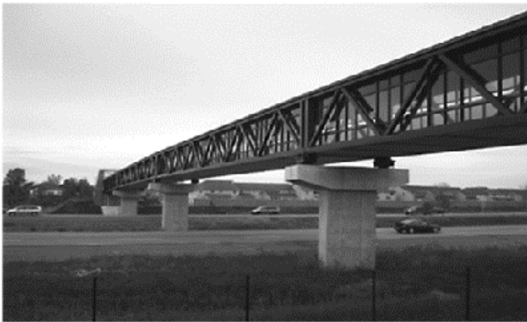
Figure 7. Pedestrian bridge over highway 417.
