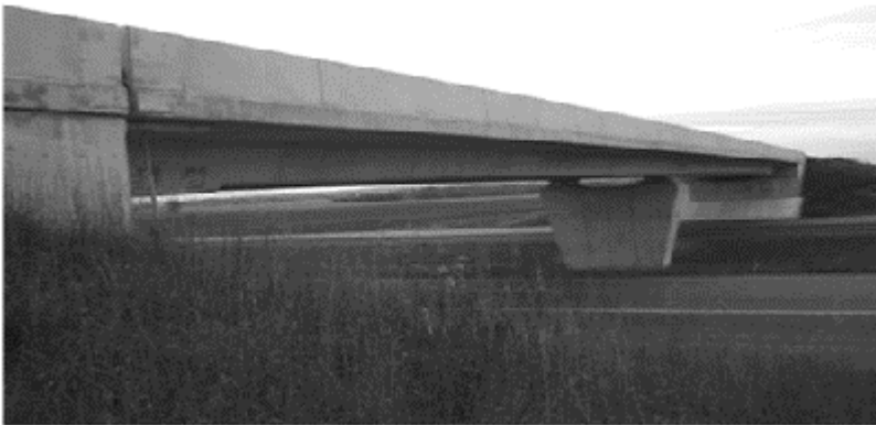
Figure 5. RR 22 over highway 417.
