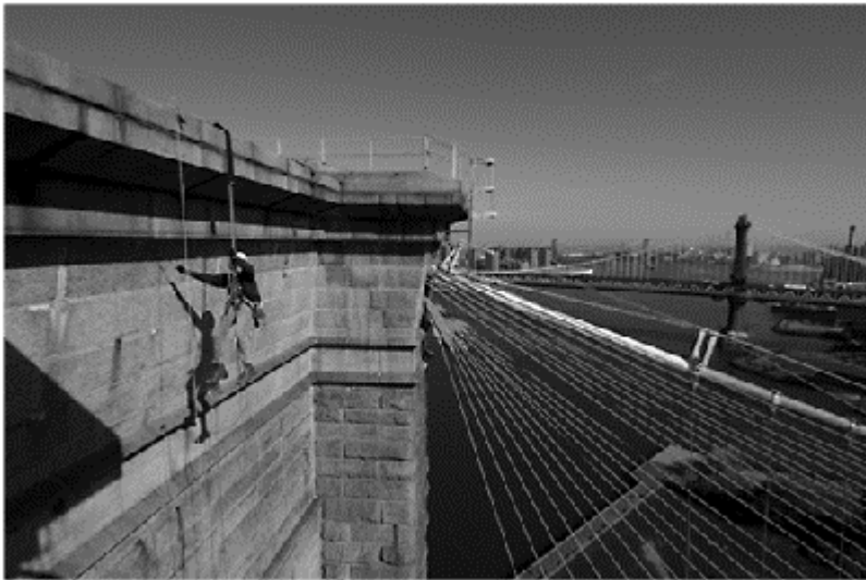
Figure 7. Inspector sounding mortar on Brooklyn Tower.
