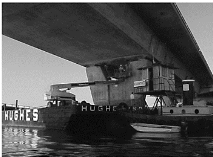
Figure 7. Barge and manlift operation.
