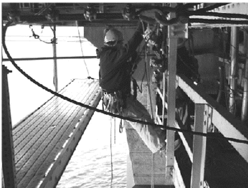
Figure 6. Access beneath deck through rope transfer.
