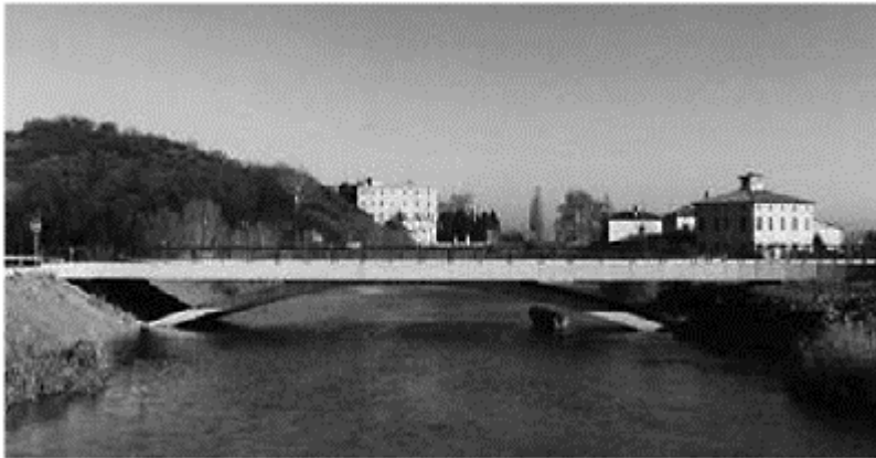
Figure 7. Bridge over river Battaglia in Battaglia Terme, Padua.
