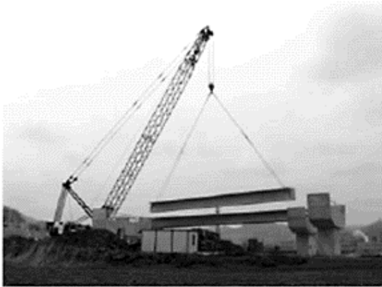
Figure 13. Erection of girders.
