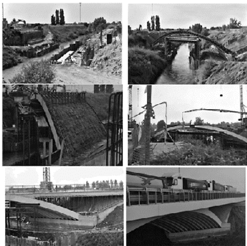
Figure 22. Stages of realization of the bridge.
