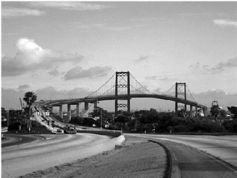
Figure 1. The Vincent Thomas Bridge located in San Pedro, CA.
