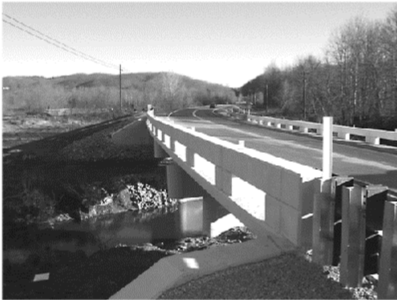
Figure 4. Above bridge after rehabilitation.
