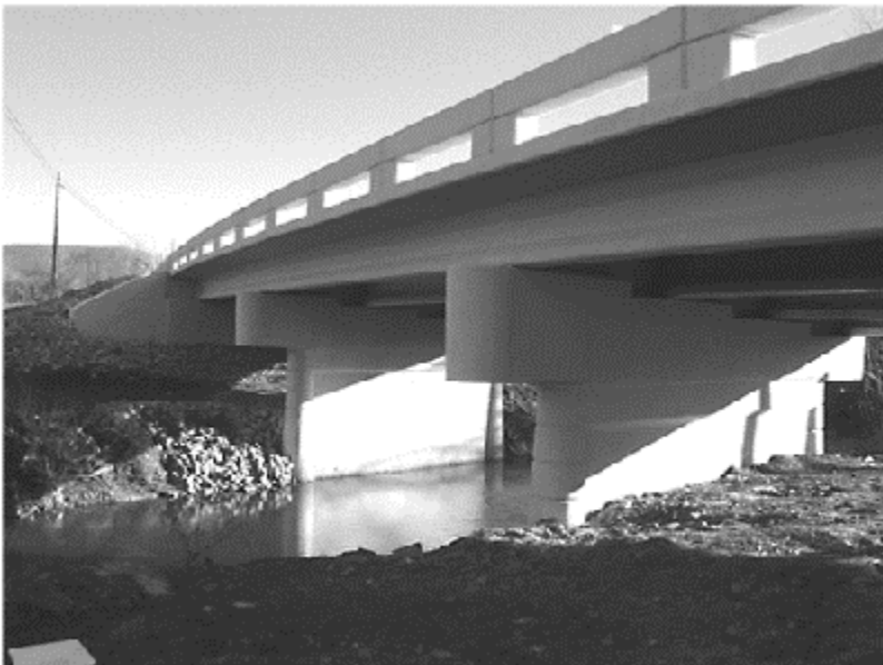
Figure 5. Below bridge after rehabilitation.
