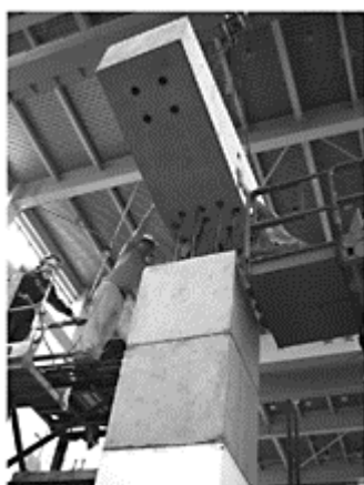
Figure 3. Assembling of pier cap.
