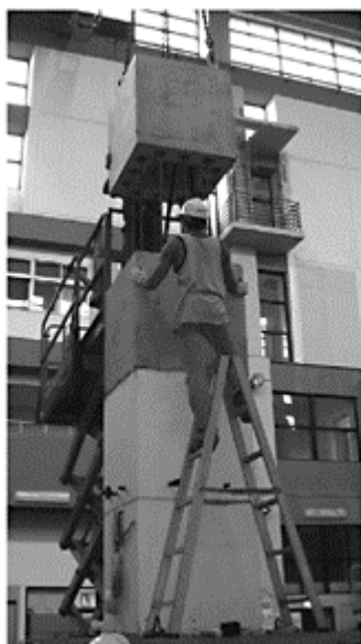
Figure 2. Assembling of column segments.
