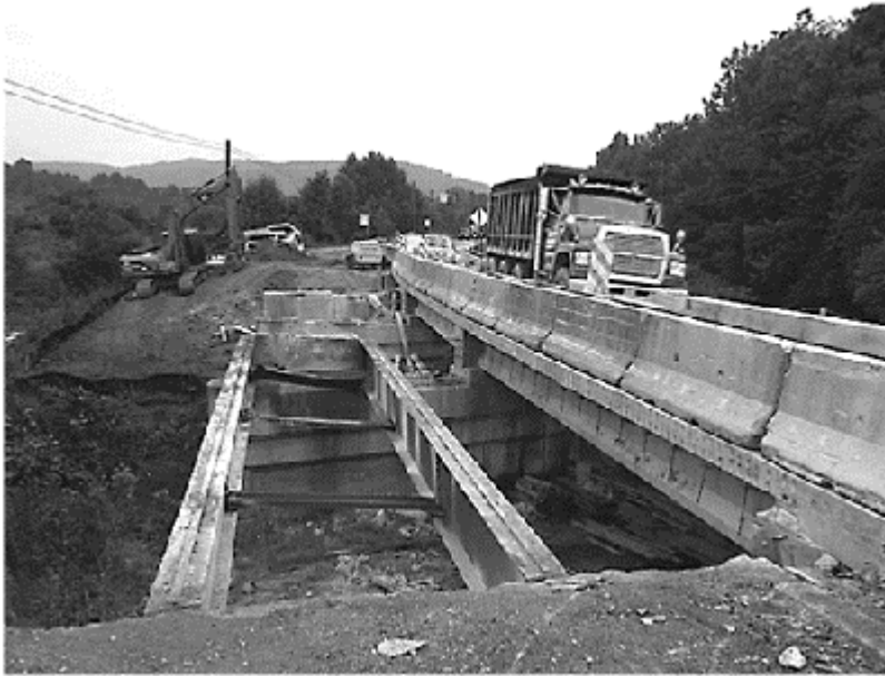
Figure 6. Phased construction and traffic control.
