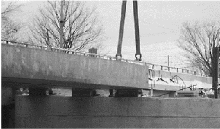
Figure 2. Precast girder being lowered onto SIB.
