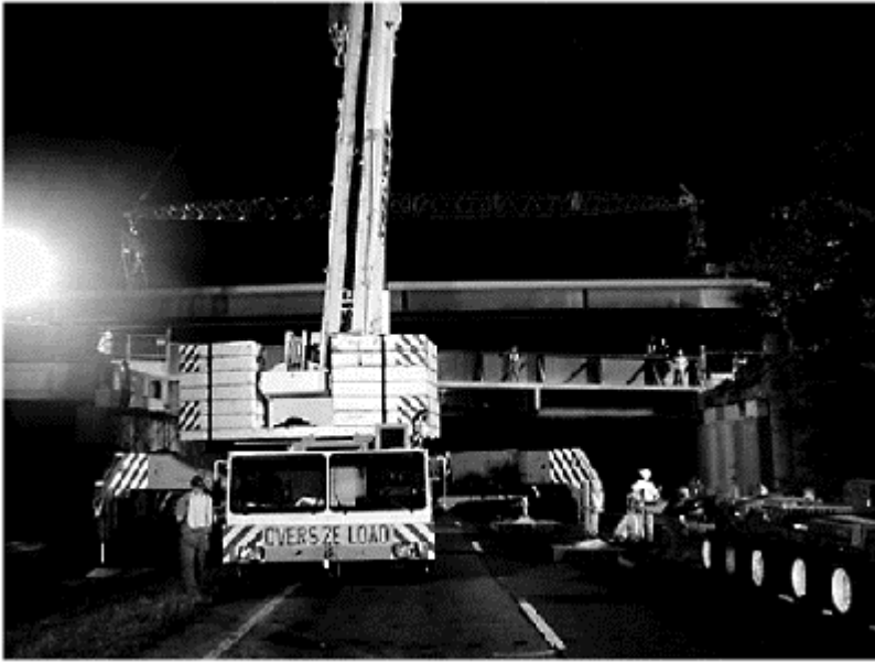
Figure 2. Night time erection of deck panels over I-295.
