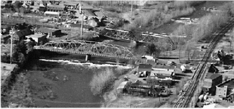
Figure 1. Aerial view of Great River Bridge.
