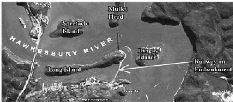
Figure 1. Aerial view of Hawkesbury River Bridge area. (Copyright 2007 – Digital globe).
