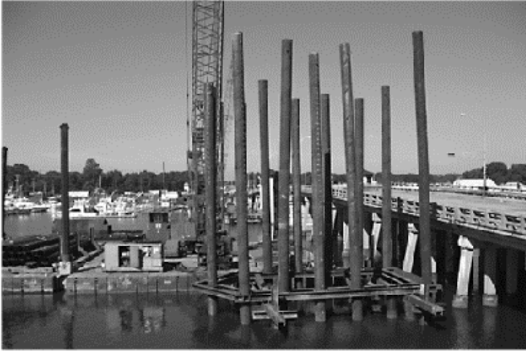
Figure 2. Perimeter piles driven with a template.
