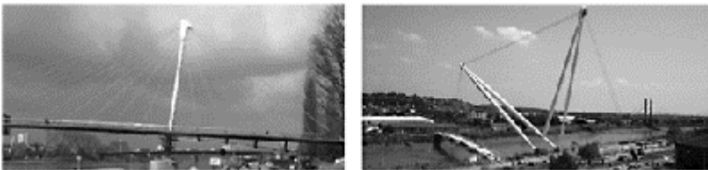
Figure 8. Pedestrian Bridge Strasbourg/Kehl (France/Germany, 2003) and River Usk Bridge (UK, 2006).
