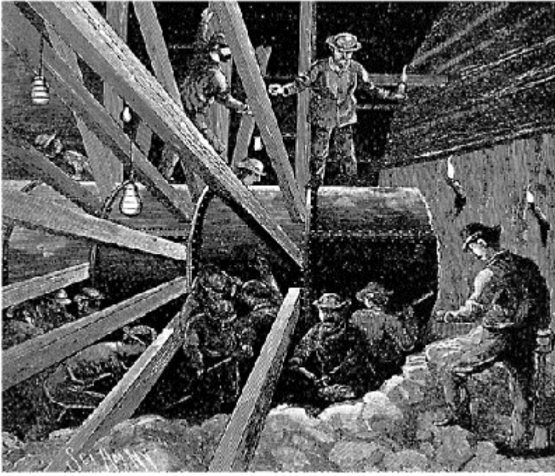
Figure 17. Use of pilot tube for the excavation of Hudson River Tunnel (Scientific American, 1889).
