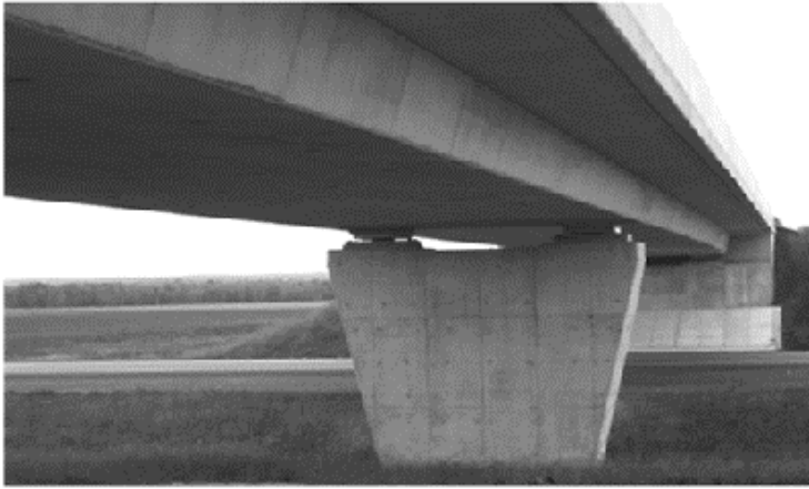
Figure 6. RR 22 pier SIB.
