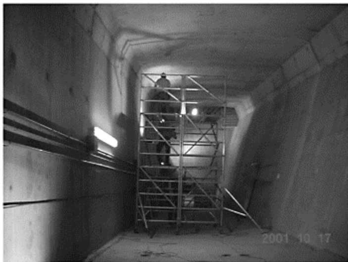
Figure 8. Interior inspection utilizing 30-foot scaffolding (Not shown to full height).
