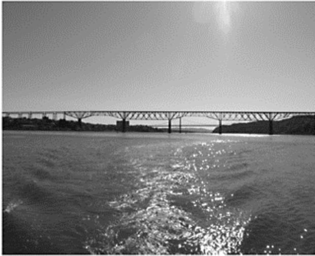
Figure 12. Overall view of the river spans of the bridge, looking north.
