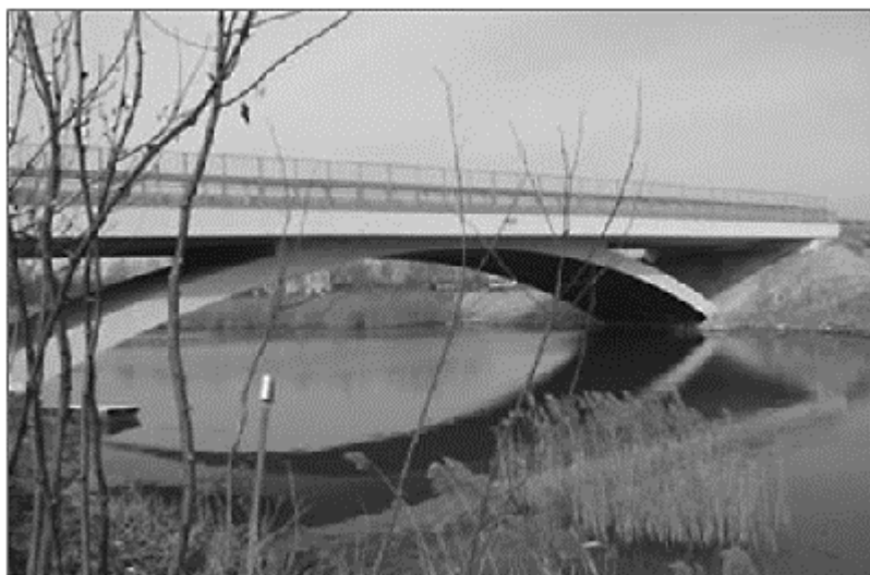
Figure 17. Final aspect of the bridge.
