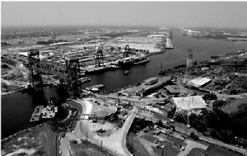
Figure 1. Current view of main span project site.
