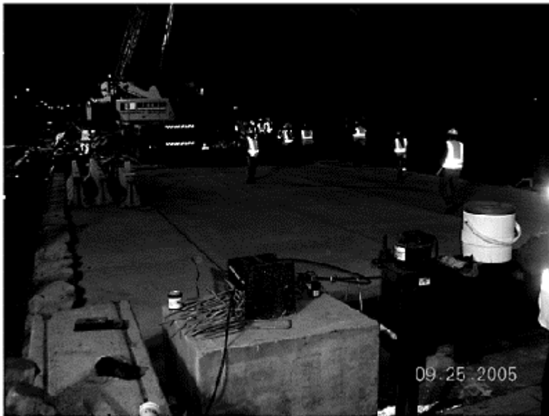
Figure 6. Erection of final deck panel of Route 1 Southbound Bridge over Mulberry Street.
