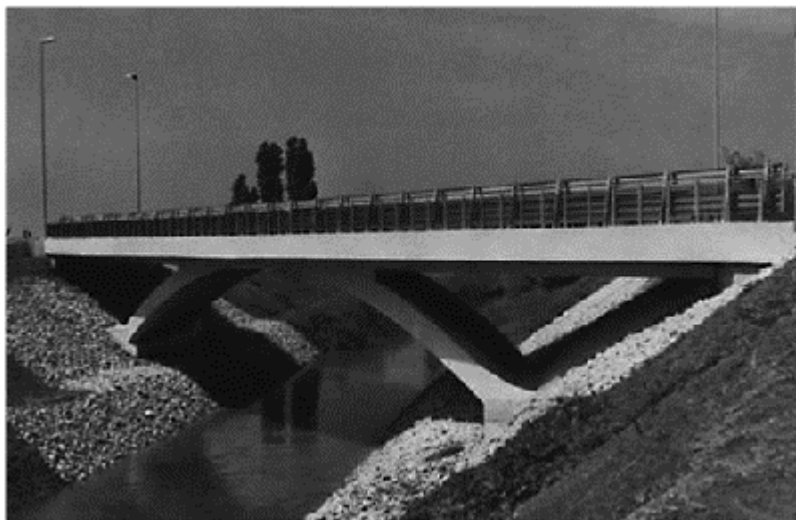
Figure 23. Aspect of the bridge.
