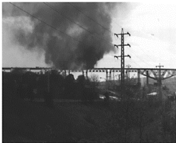
Figure 9. 1974 fire on east approach.
