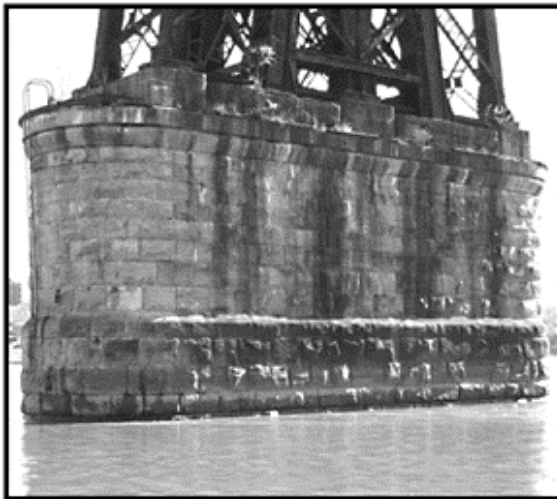
Figure 13. Pier 2 west and north elevation.
