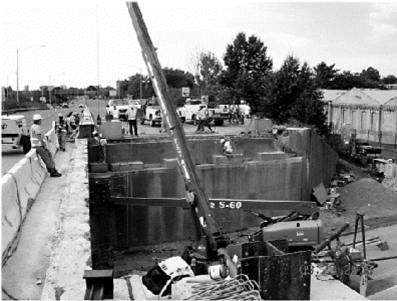
Figure 5. Initiation of erection of Route 1 Southbound Bridge over Mulberry Street.
