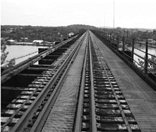
Figure 3. A current view of bridge surface looking east.
