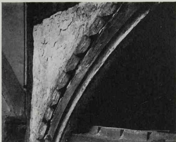
31. The arched brace of a twelfth-century Western roof. The Bishop's Palace, Hereford
