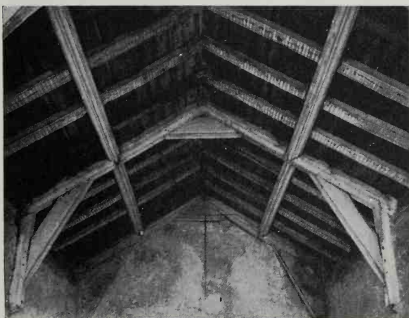
32. A primitive example of a framed 'principal'. Sedgeford church, Norfolk
