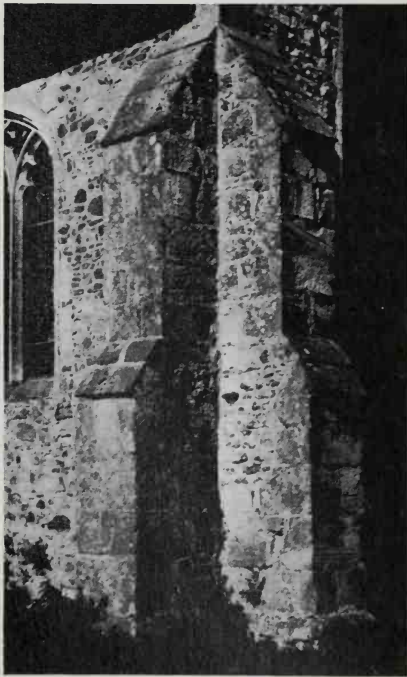
48. A buttressed angle of the Early Gothic period
