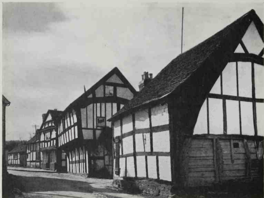
7. The nearest of these sixteenth-century houses at Weobley in Herefordshire is built on 'crucks'
