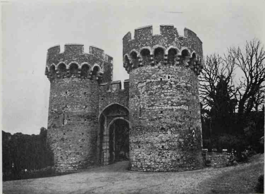
57. A gatehouse with its tower-tops 'machicolated' at Cooling Castle in Kent
