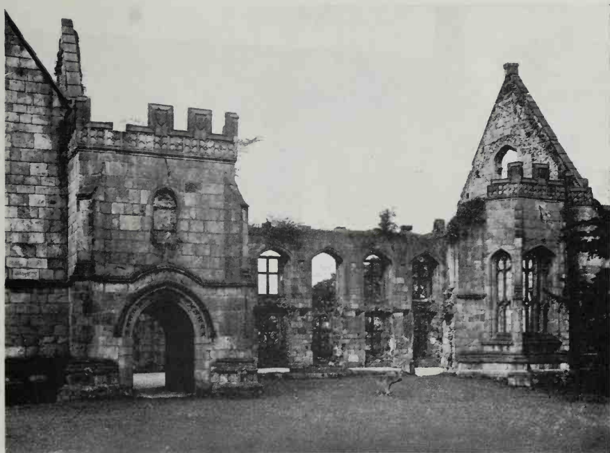
113. The hall porch and bay window of a late mediaeval great house at South Wingfield, Derbyshire
