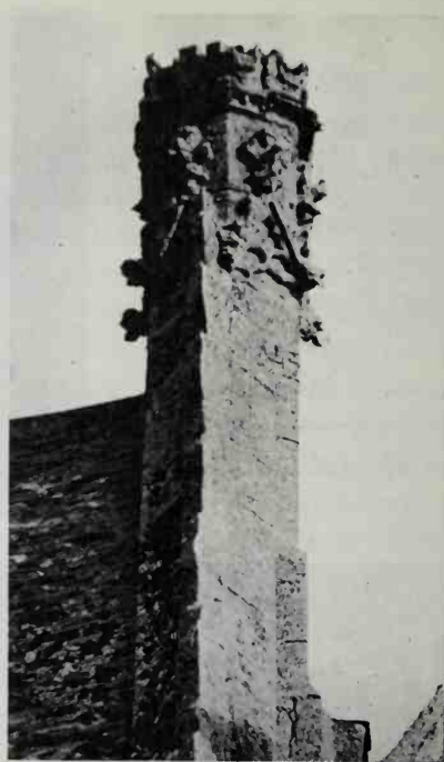
182. Late mediaeval chimney
