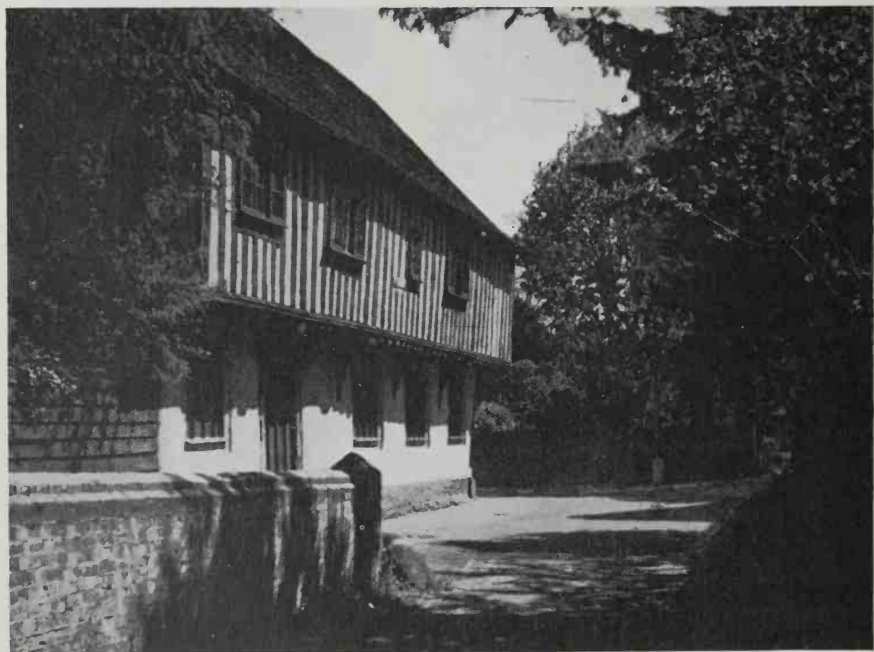
8. Fifteenth-century timber-framed house at Lavenham in Suffolk having the upper storey 'jettied out'
