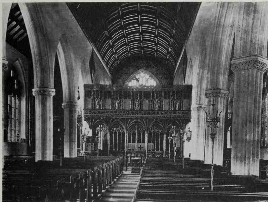
87. A Devon 'hall church' with its cradle roof and elaborate rood-screen. Kenton church
