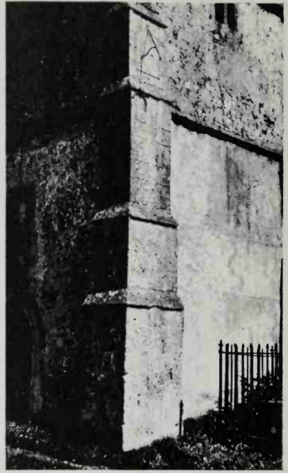
47. Thickened-out angle typical of the twelfth century
