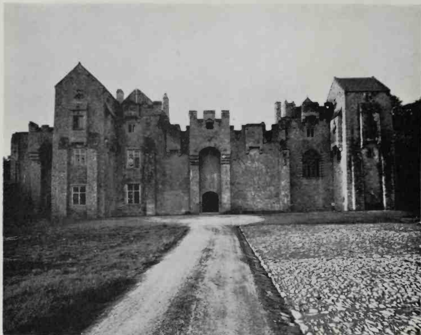
56. A late mediaeval manor house fortified with 'drop-boxes'. Compton Castle, Devon
