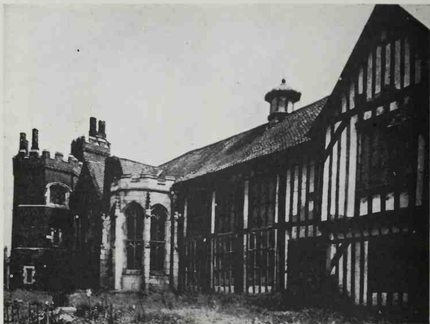
167. A stone bay window has been added to this fifteenth century hall of Gainsborough Old Hall, Lincolnshire
