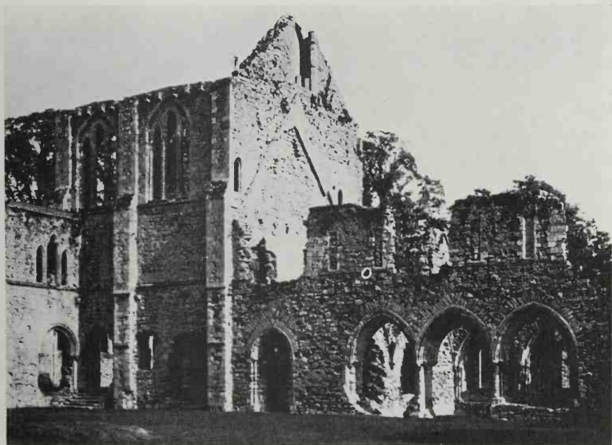
126. The ruins of the monks' house attached to the south transept of Netley Abbey, showing the entrance to the chapter house
