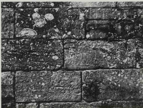
16. Late mediaeval masonry
