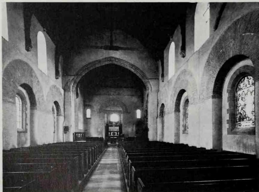
82. Eleventh-century nave arcades with arches turned in Roman brick. Brixworth church, Northamptonshire
