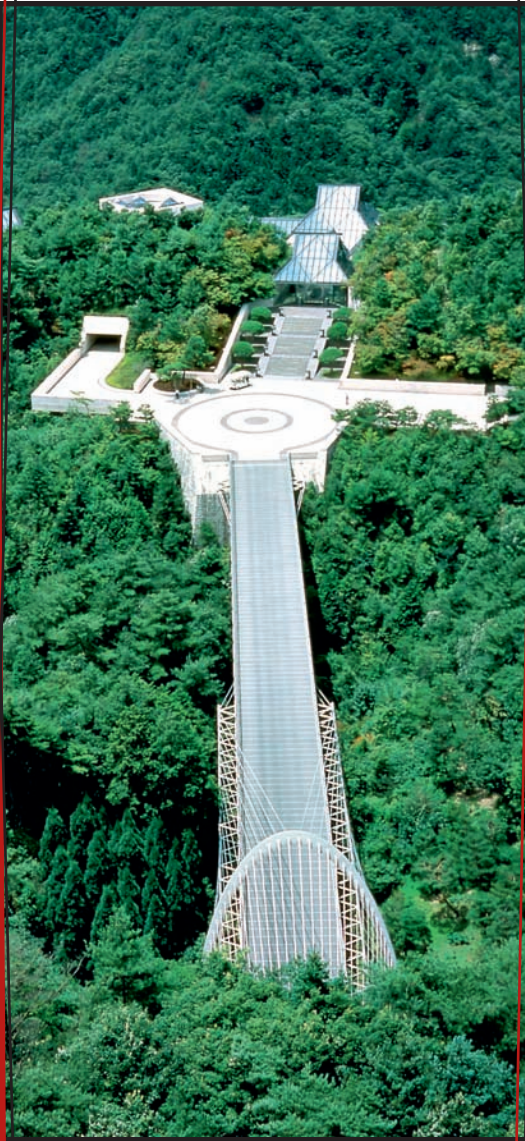
THE GRACEFUL SUSPENSION BRIDGE OVER THE GORGE LEADS TO THE ENTRANCE OF THE MIHO MUSEUM. EIGHTY-FIVE PERCENT OF THE MUSEUM LIES UNDERGROUND. THE CONTOUR OF THE ORIGINAL MOUNTAIN REMAINS UNCHANGED.
