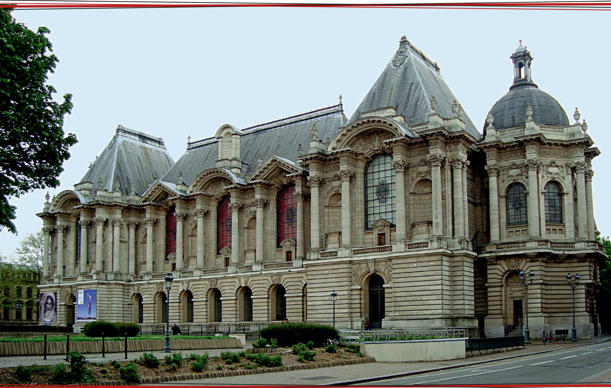
CLASSIC ELEMENTS IN PERFECT SYMMETRY ARE TYPICAL OF THE BEAUX-ARTS STYLE PRESENT IN THE COLUMNS, BALUSTRADES, ARCHED WINDOWS, AND DOORWAYS OF THE FRENCH ART MUSEUM PALAIS DES BEAUX-ARTS DE LILLE.
