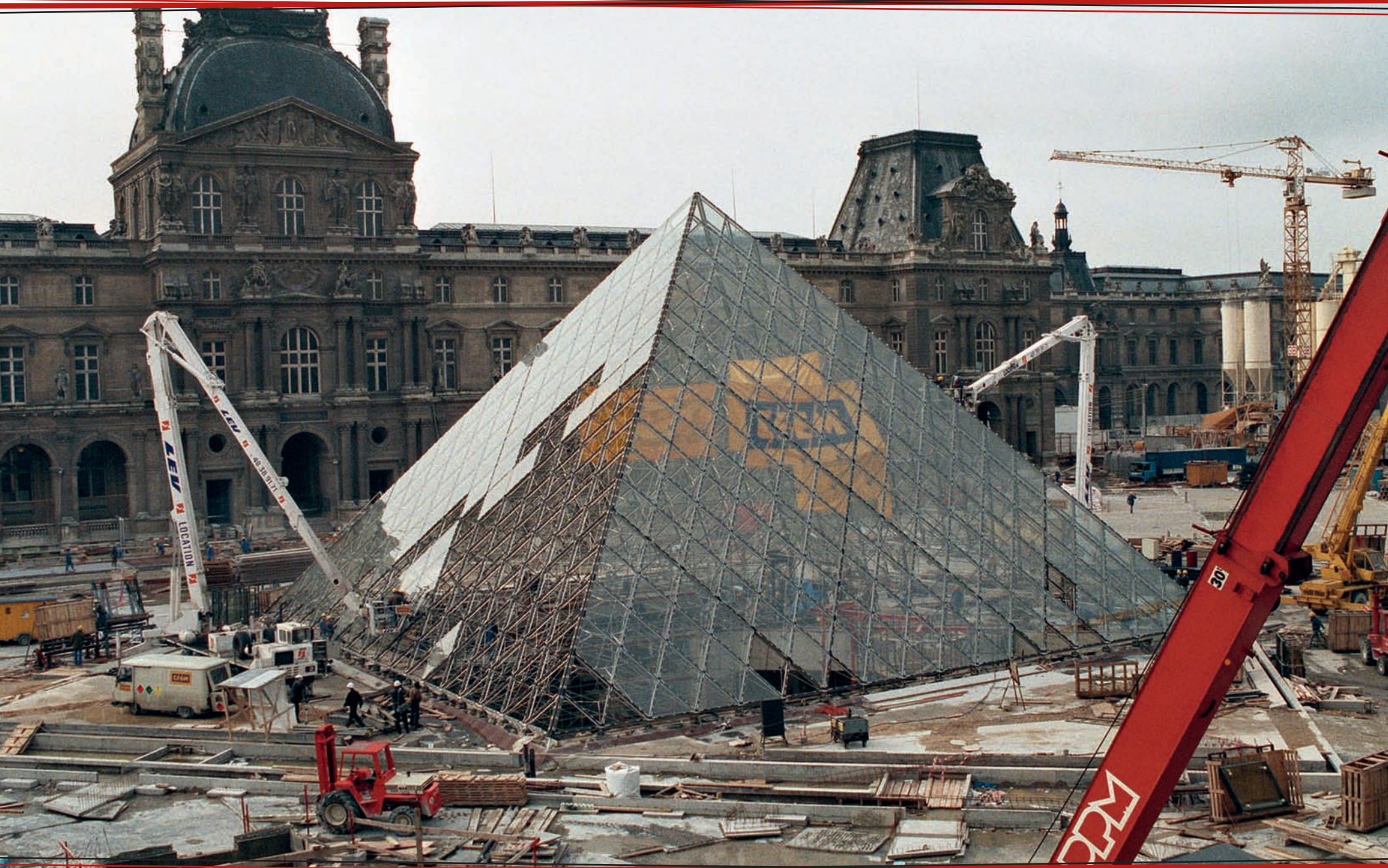
UNDER CONSTRUCTION, THE PYRAMID RISES IN THE CENTER OF NAPOLEON'S COURTYARD.
