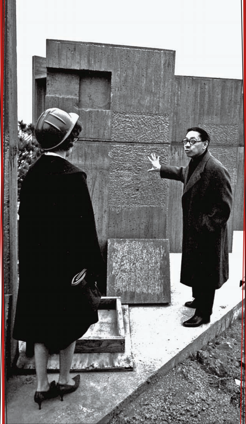
PEI INSPECTS THE COLOR OF TEST SLABS MADE OF CONCRETE AND STONE FOR THE NCAR BUILDING. HIS SELECTIONS BLEND INTO THE LANDSCAPE, THE SAME WAY AS THE PUEBLO DWELLINGS.
