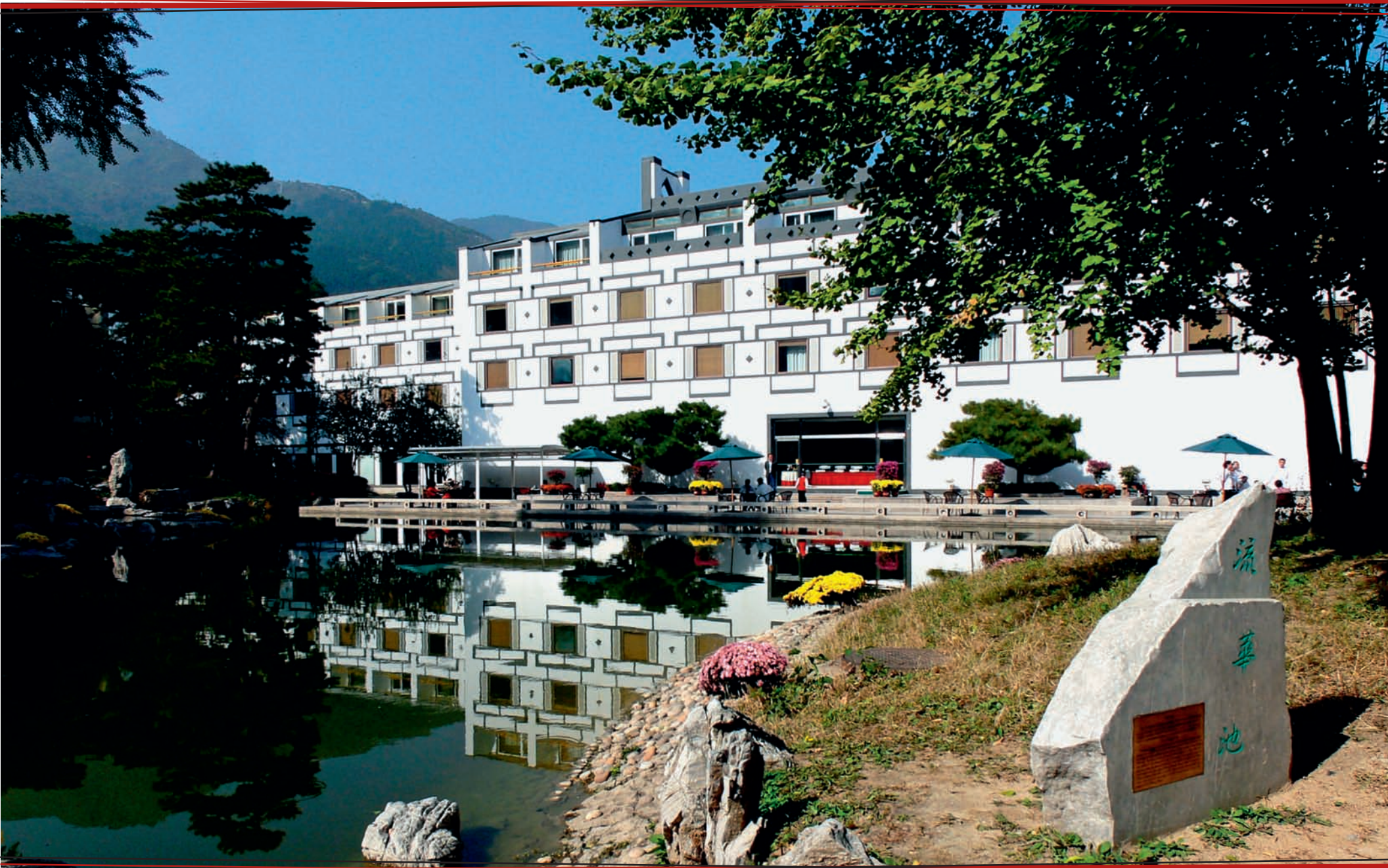
FRAGRANT HILL HOTEL'S STRONG, GEOMETRIC DESIGN IS MODERN WHILE RESPECTING CHINA'S ARCHITECTURAL PAST.
