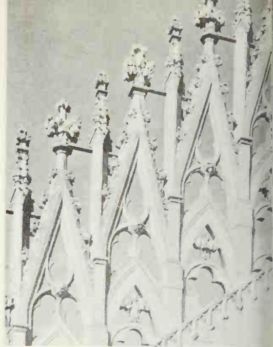
8. Milan Cathedral. Tracery work; left: old pinnacles, right: pinnacles of 1927.
