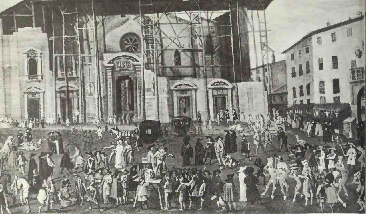
18. Milan Cathedral. State of the façade in 1683. Anonymous painting, showing old S. Maria Maggiore inside the new structure.
