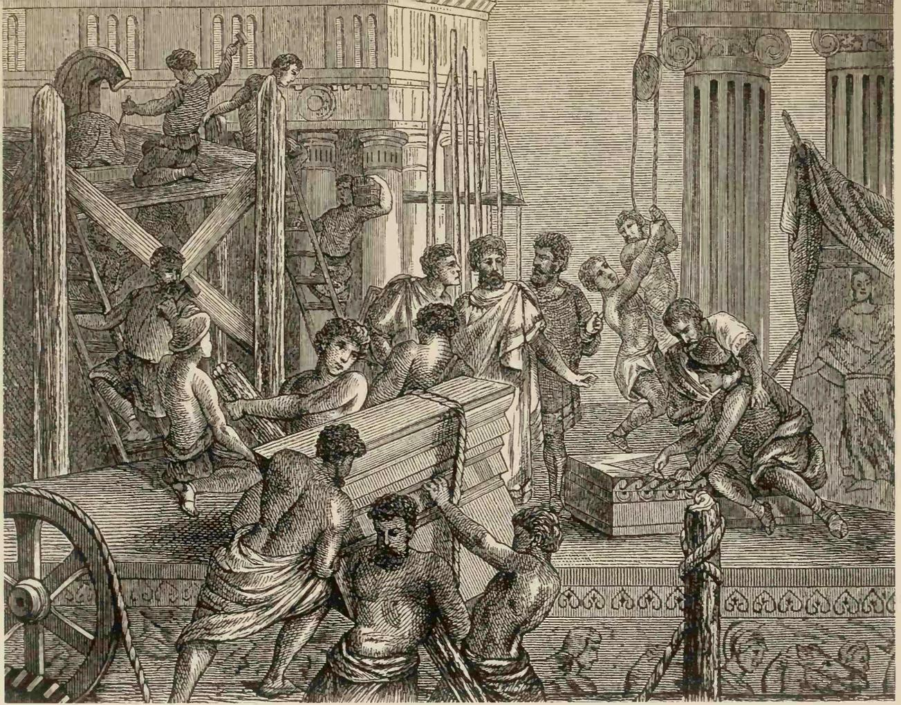
chunks of stone called **drums** to make the columns. Each of the Parthenon's columns consisted of about eleven drums stacked on top of one another, with a Doric capital at the top. A single drum weighed from five to ten tons. Lifting the upper drums into place was a daunting task.
