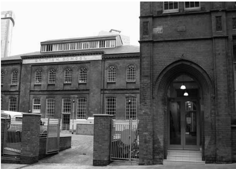
'Schools into homes 2006-7'. This development in Birmingham, England uses the 'shell' of the former Severn Street School, the city's first Nonconformist school, started in 1809. The First Day School was opened on this site in 1845 and was founded by the Quaker merchant, anti-slavery and peace campaigner Joseph Sturge to teach adults and poor children.
