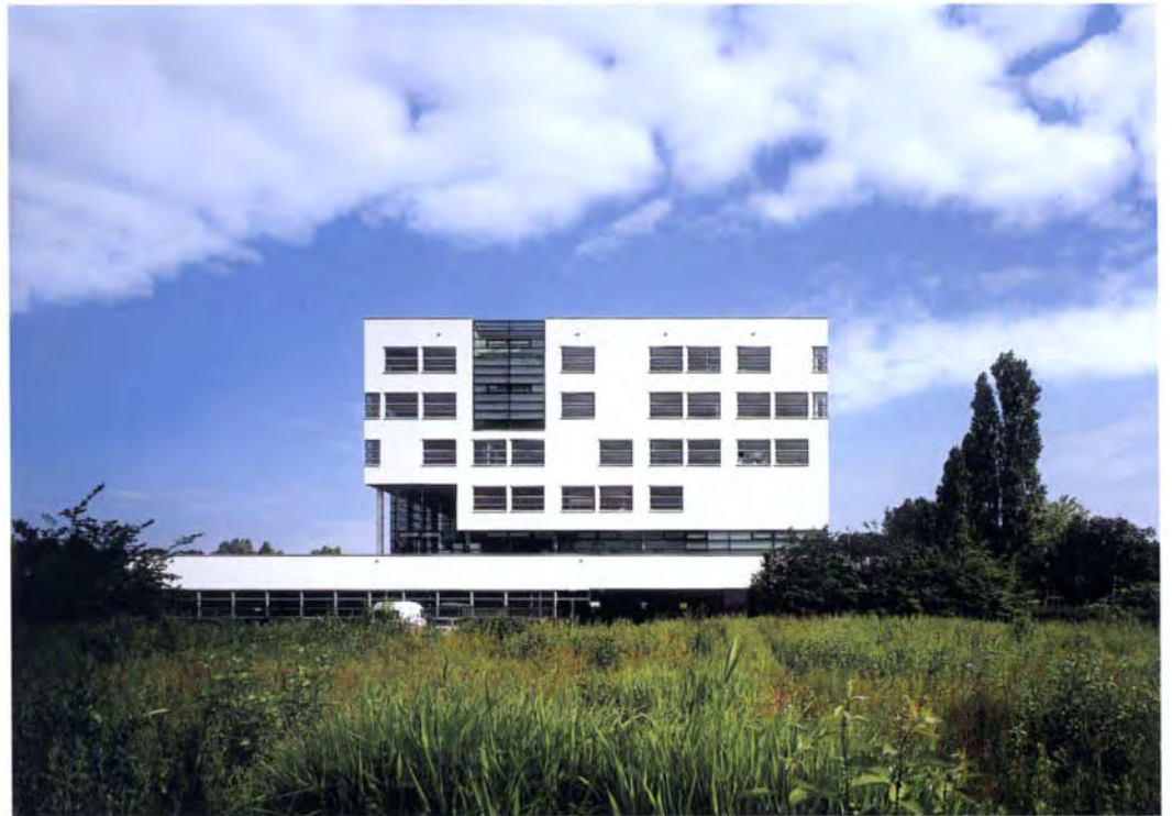
Entrance staircase | Lateral façade with technical classrooms in the 'base level' | View of central void | Grand staircase | Study area outside the classroom
