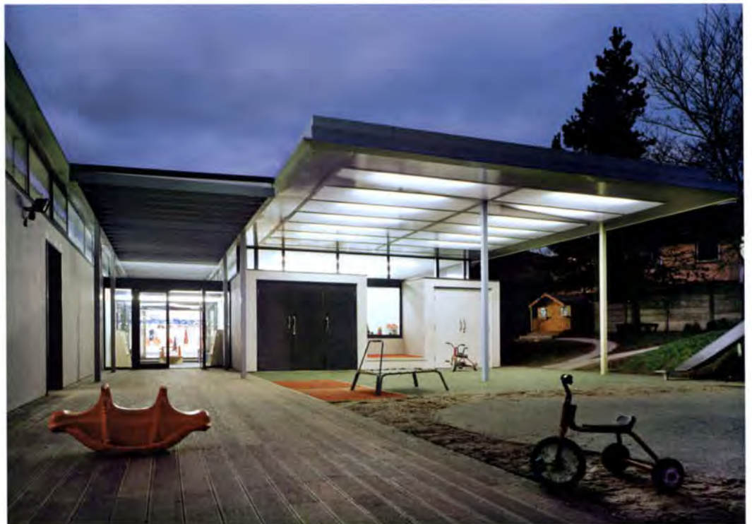
View of the stone wall and horizontal roof plain from the street | View from the courtyard looking towards the covered outside play area and storage cupboards | Views into the main activity area showing the even colorless clearstory lighting
