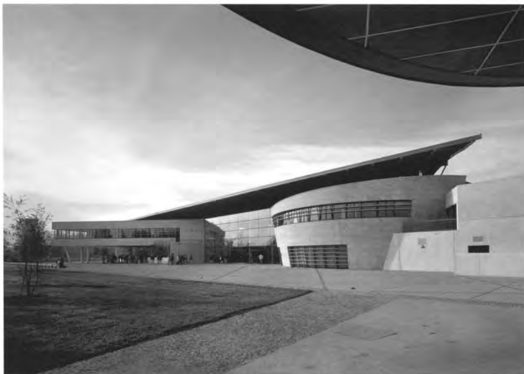
A bridge link across the courtyard gardens connects the teaching blocks | The main communal building with learning resources and social areas projecting out into the landscape | The entrance lobby with mezzanine bridge link | Typical internal corridor within the teaching blocks
