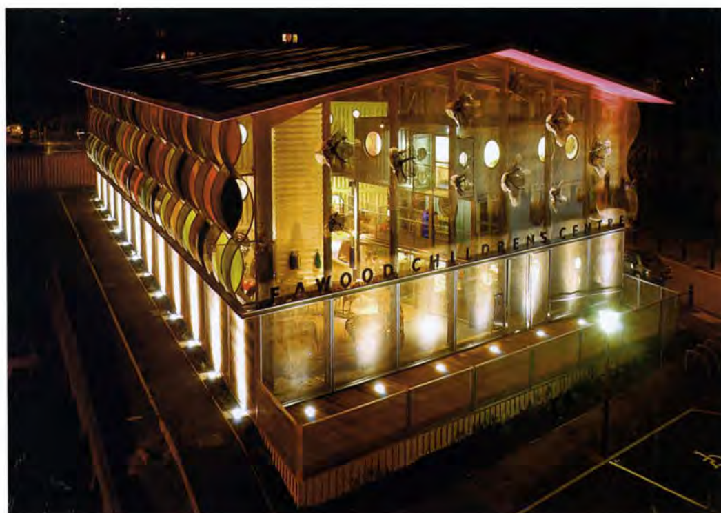
Site plan | Mesh cladding to the lower part of the façade will eventually be covered with climbing plants | Detail of pendant walls | Interior view showing the stacked containers behind which is the stage willow eave around the play piazza
