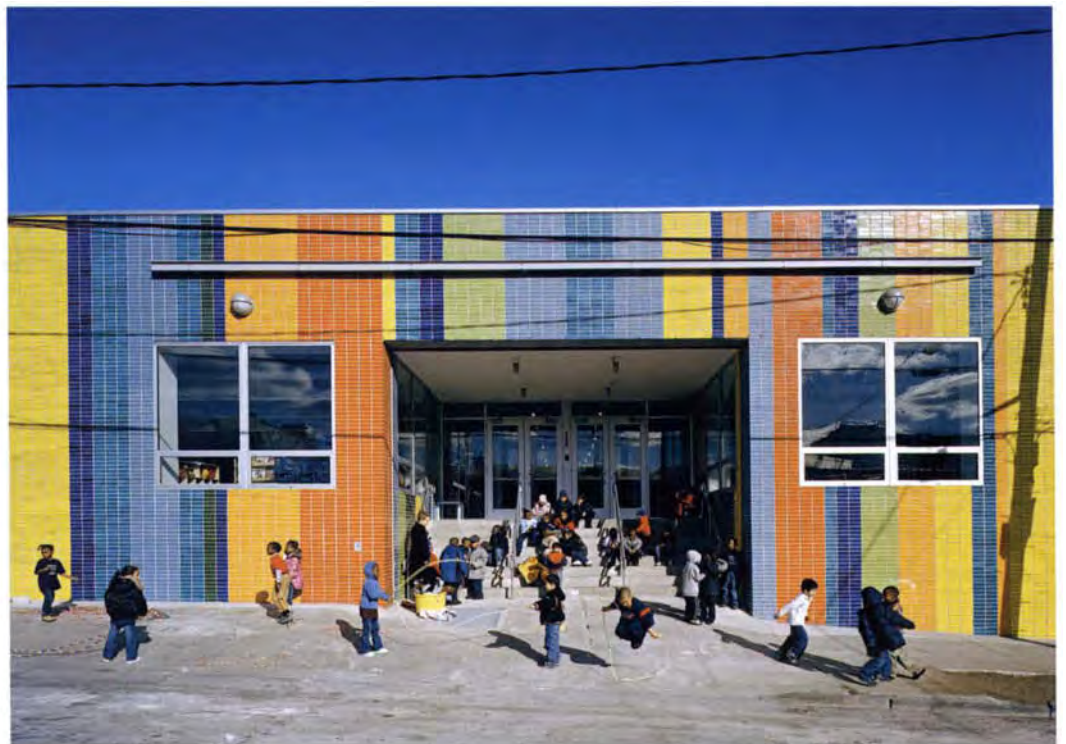
Coloured tiles on the street façade counter the drab post industrial context | Conceptual façade with the suggestion of the use of the dead-end street as a playground during school hours
