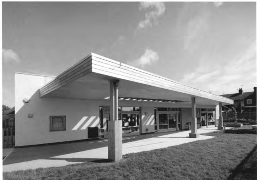
The building block composition around the main entrance | Rear façade | Main children's activity area showing sliding folding wall panels | Circulation area
