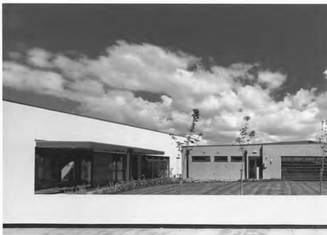
End façade at the highest point of the building with child height coloured optic windows | The entrance court with the coloured 'Sure Start' building detached from the main nursery | View from the courtyard looking towards the children's cloakroom area | Activity area | Courtyard with picket fence
