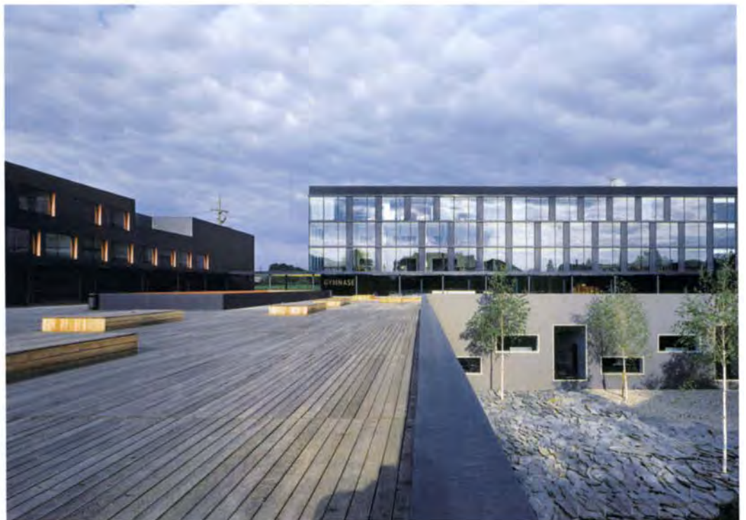
Rear façade of vocational school building | View towards the grammar school across the upper deck with the lower courtyard | View of lower courtyard | Link bridge across one corner of the lower courtyard
