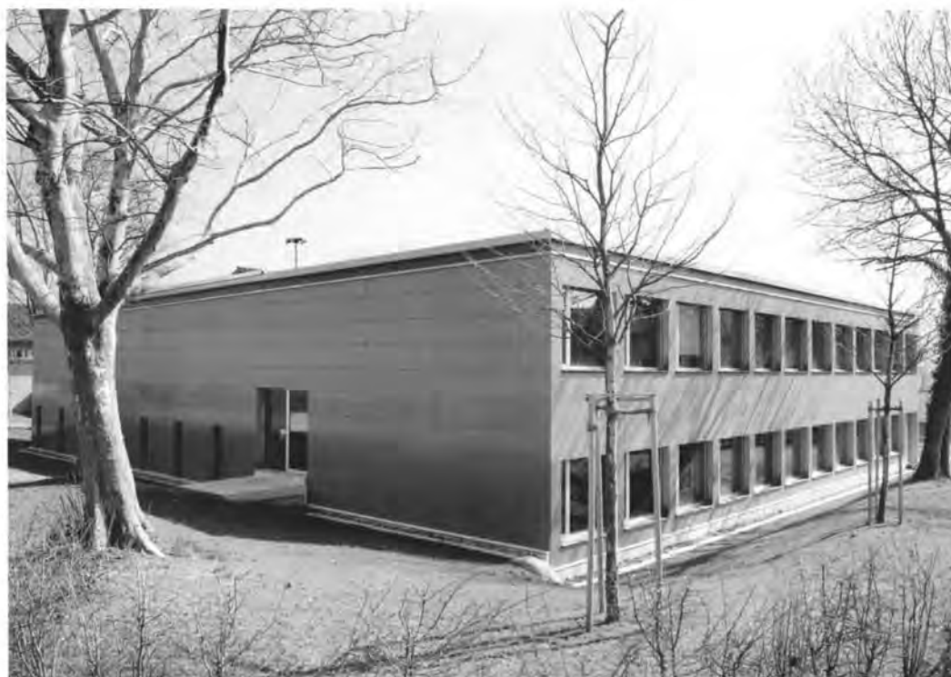
Terrace with new extension connected elegantly onto the existing building | View from northeast | Renovated classroom with coordinated furniture and timber wall paneling | Old building with new corridor façade with integrated storage and pupil lockers
