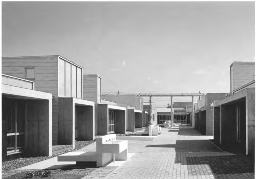
Site with roof plan | View down courtyard street | Circulation space | Typical open classroom with English class underway
