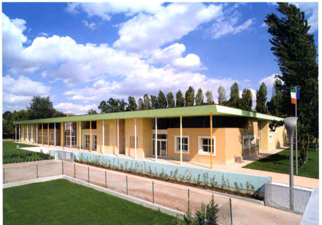
Views of covered colonnade providing a natural extension to the interior space out into the gardens | Night view | The central square with views to the courtyard garden, a little bit of outside space captured within the building
