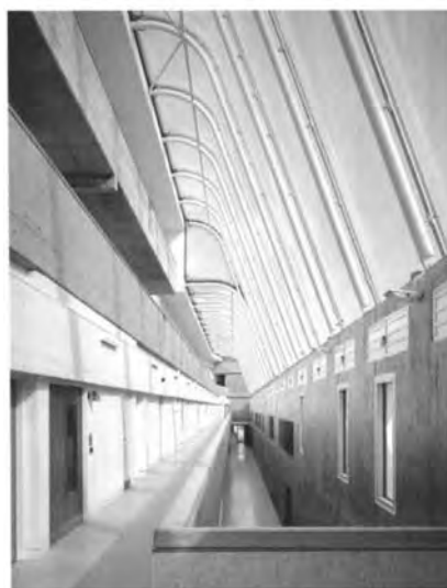
Internal views of ETFE atrium. Academy of St. Francis of Assisi, Liverpool
