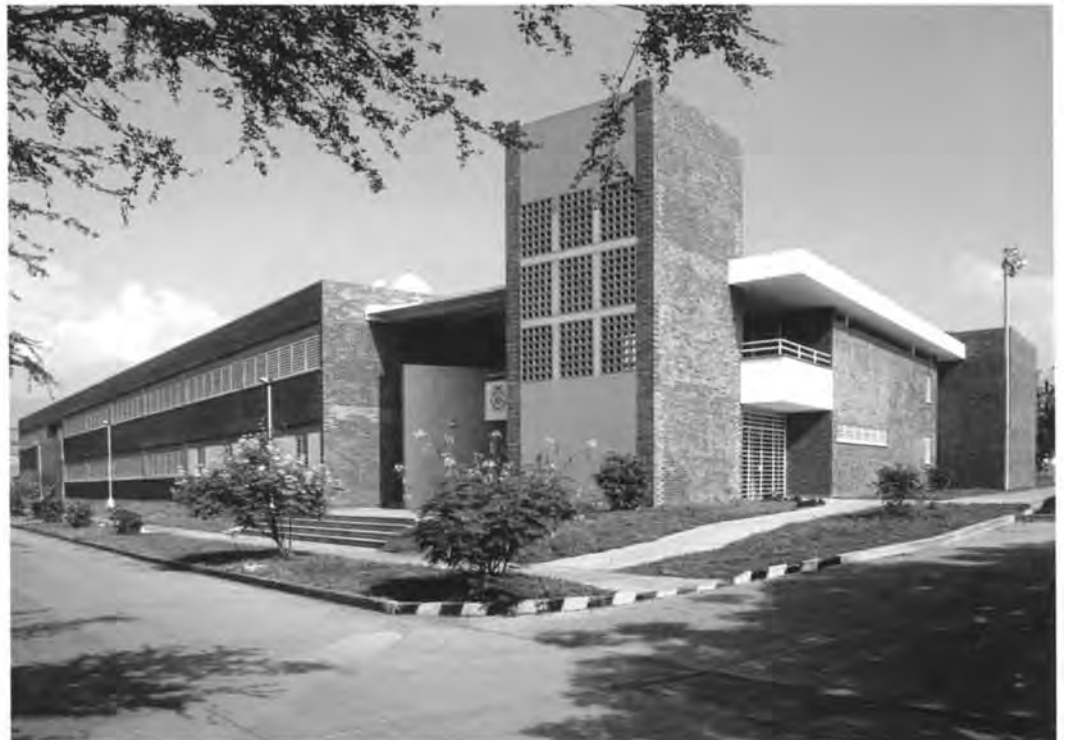
The colonnade provides shade for the classrooms | Entrance corner with stair tower for cooling and ventilation | Views of internal courtyard showing restrained use of colour
