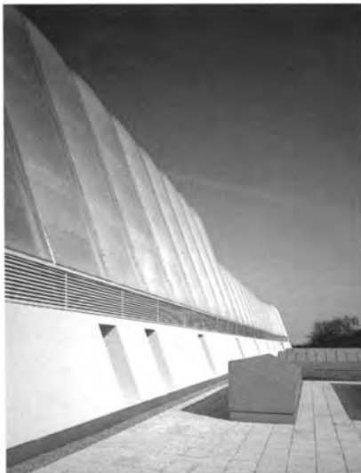
South-facing passive solar ETFE atrium. Academy of St. Francis of Assisi, Liverpool, Buro Happold
