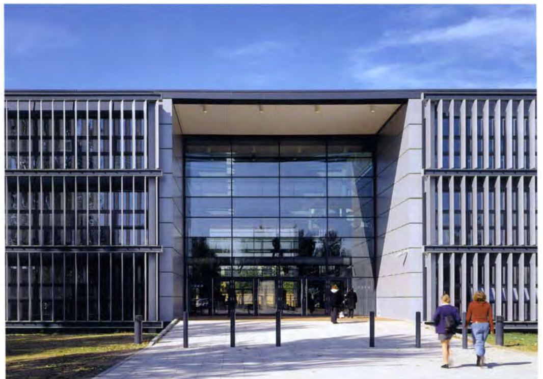
View of teaching spaces from across the art courtyard | Main entrance | Interior view of technology courtyard | View of business courtyard with restaurant beneath mural showing all new pupils | A lesson takes place in the courtyard
