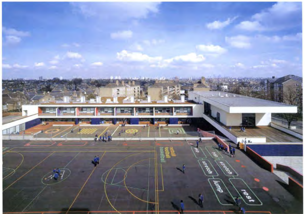
Hall with cantilevered roof | Distant view from the south with the main hall and social deck on the left | Main entrance | Nursery entrance | Two-storey classroom block
