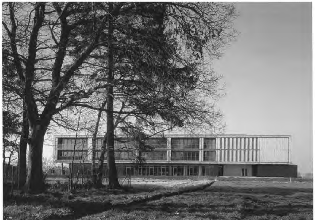
View towards the main entrance | Elevation from the riverbank | View to internal courtyard with broad steps running up to first floor teaching areas | View of typical classroom, with the use of simple materials and even controlled colour coding
