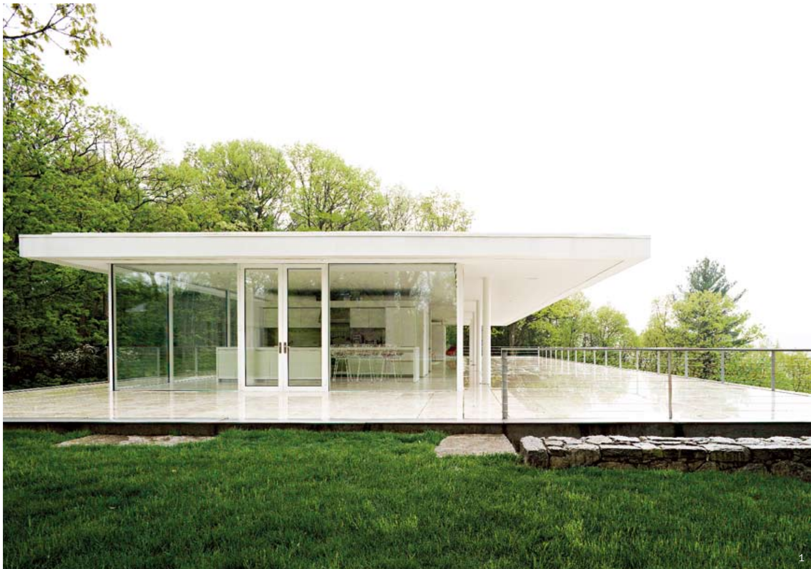
1. The terrace paved with white tiles can receive all the sunshine 2. The light and shadow endows the space with different expressions
