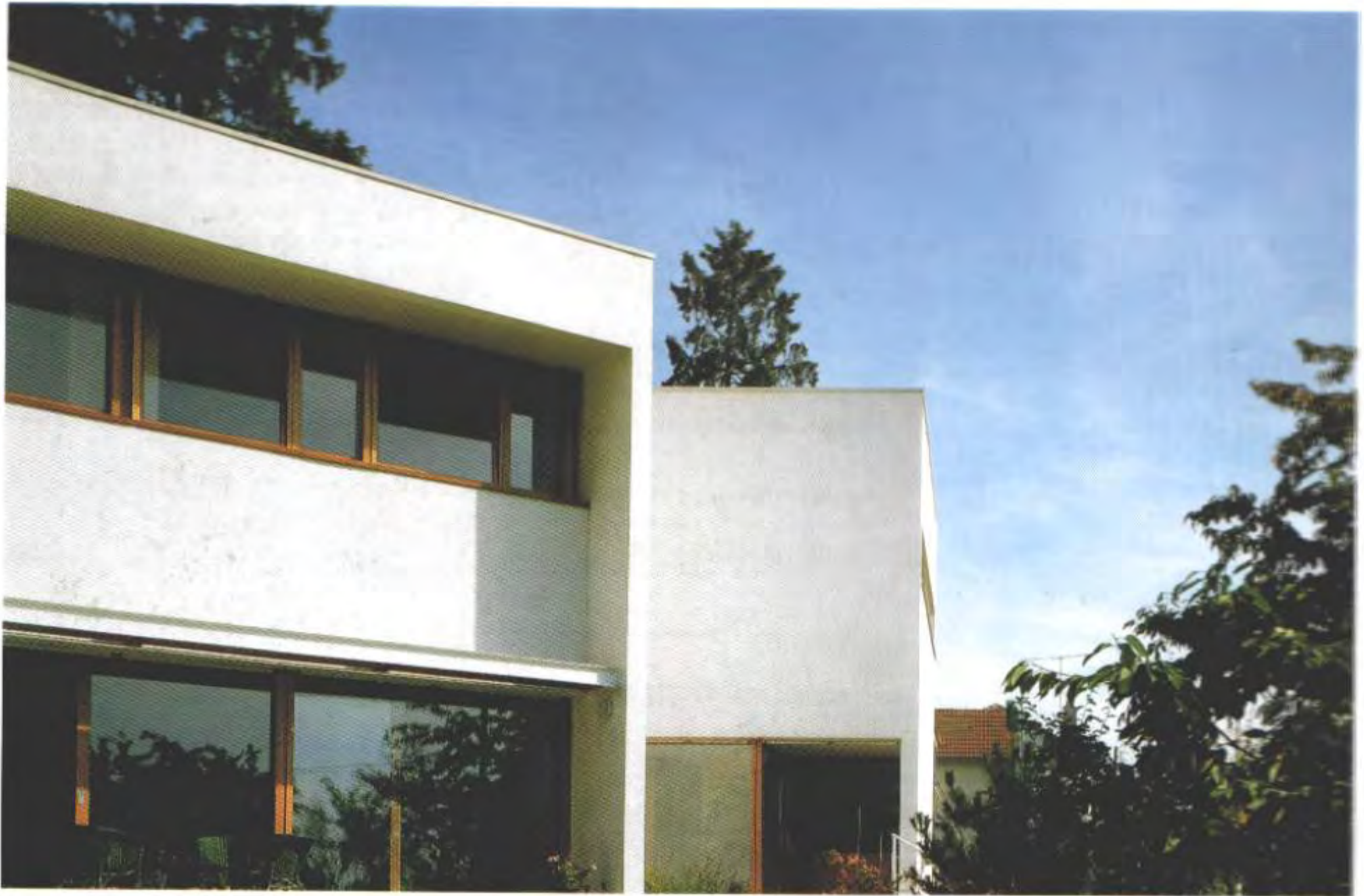
Details of the encounter between the two volumes, the access staircase and the part of the parallelepiped that opens onto the garden.
