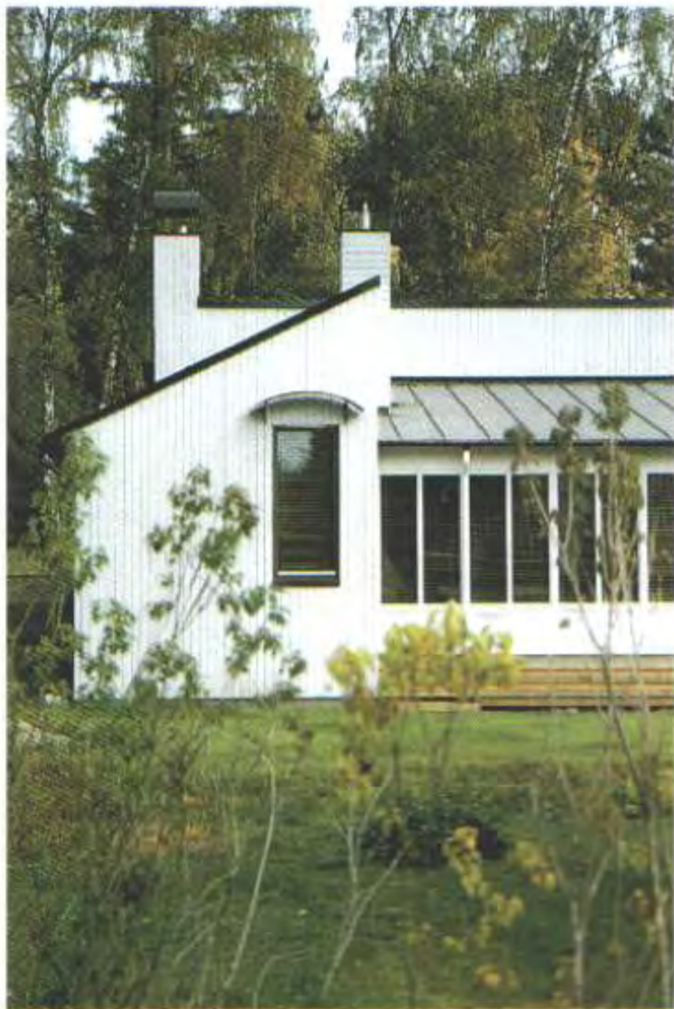
Part of the southwest facade. Parte de la fachada sudoeste.
