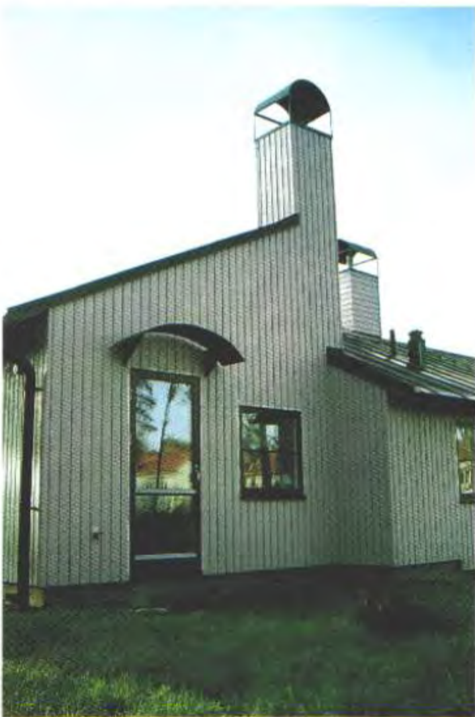
The kitchen entrance, northwest facade. Entrada de la cocina, fachada noroeste.
