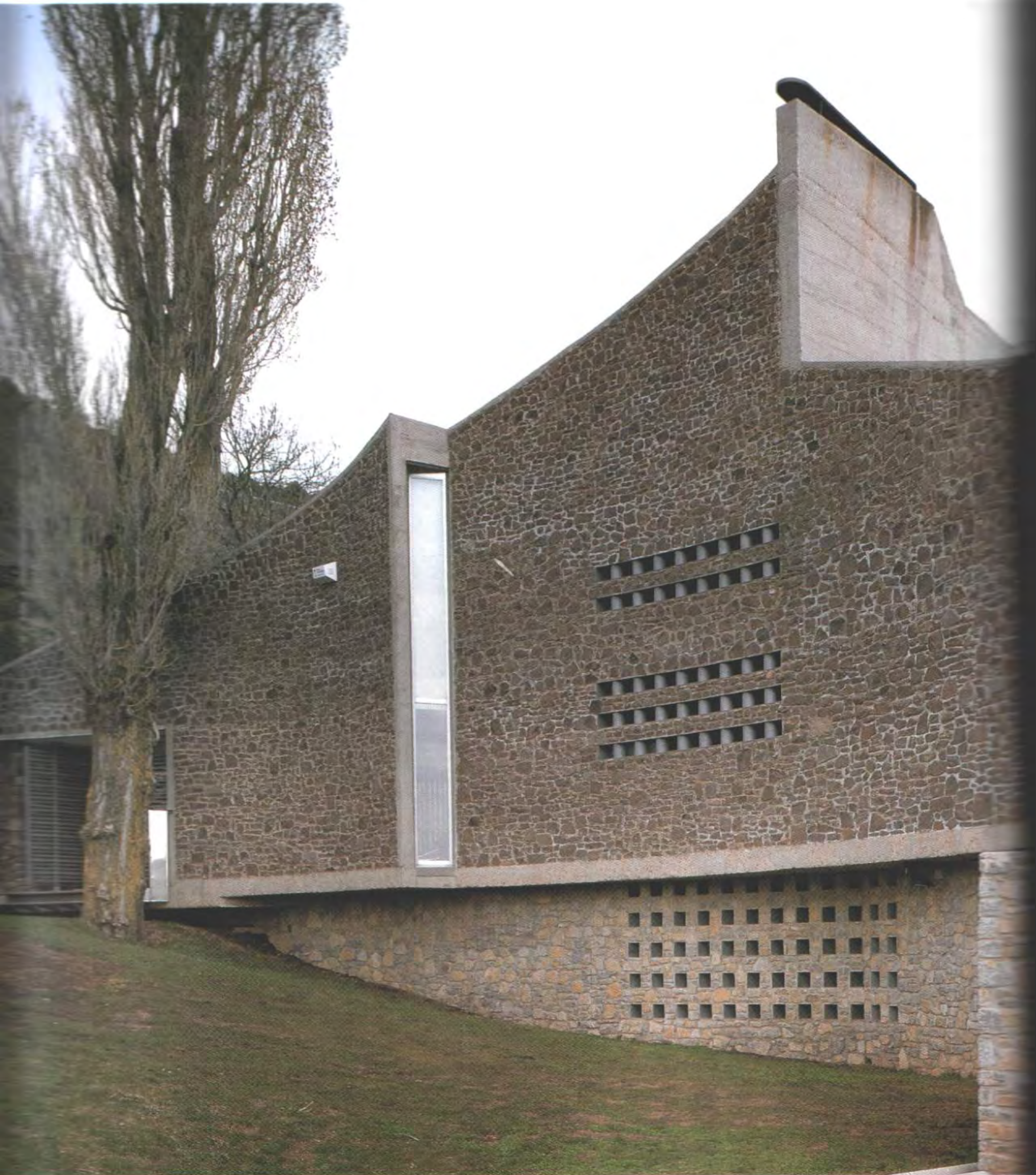
View of the western elevation, with its two grades of local masonry. The dwelling descends, conforming subtly to the topography of the terrain. The upper storey opens onto a terrace which faces the countryside.
