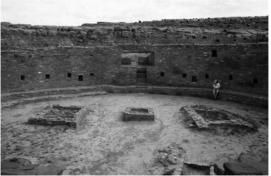
The Anasazi built in stone as well as adobe, or mud brick, specializing in walls without mortar that were constructed so well that they have stood the test of time. Source: Ken Breish
