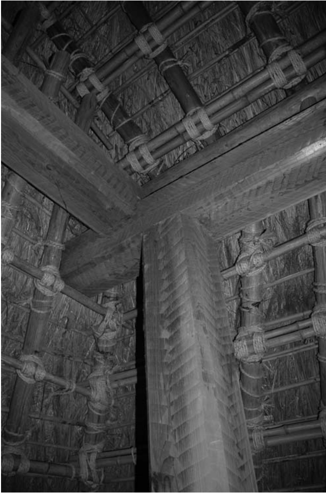
Before the Yayoi culture entered Japan, the indigenous people built houses that were partially dug into the earth, which had heavily thatched roofs like the minka farmhouses today. Source: James Steele
