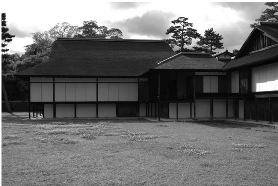
Katsura is the perfect example of a sukiya style traditional Japanese house because of its raised floor, light frame construction, wide overhanging eaves, and shoji , or rice paper, screen components. Source: James Steele
