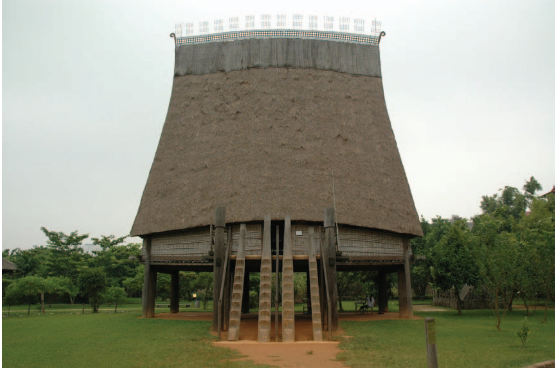
Bahnar The Bahnar house has a distinctive high roof and is raised far above the ground to increase natural ventilation and provide protection. Source: James Steele
