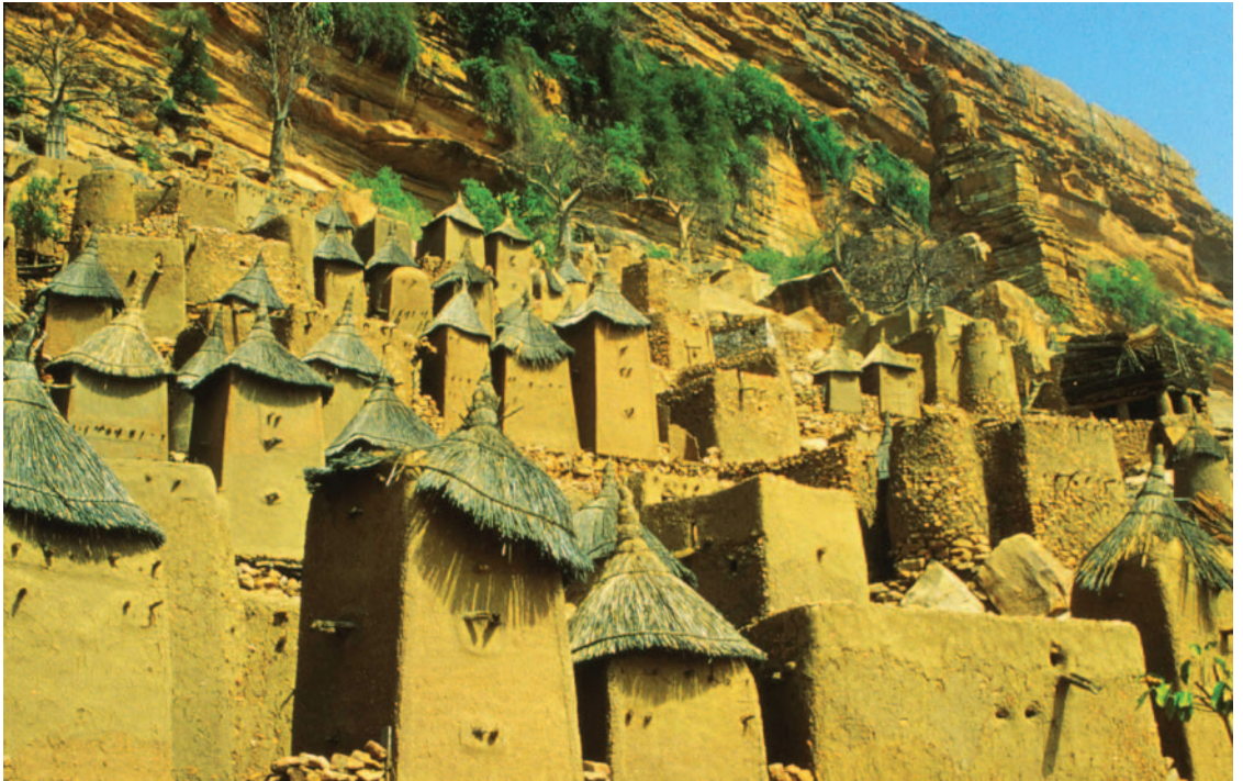
Dogan Houses The Dogon people of Mali build their houses of mud brick and use thatch for the roofs. Because each individual or family has a freestanding house and they are typically clustered close together, their settlements have a distinctly vertical, uniform appearance. Source: James Steele
