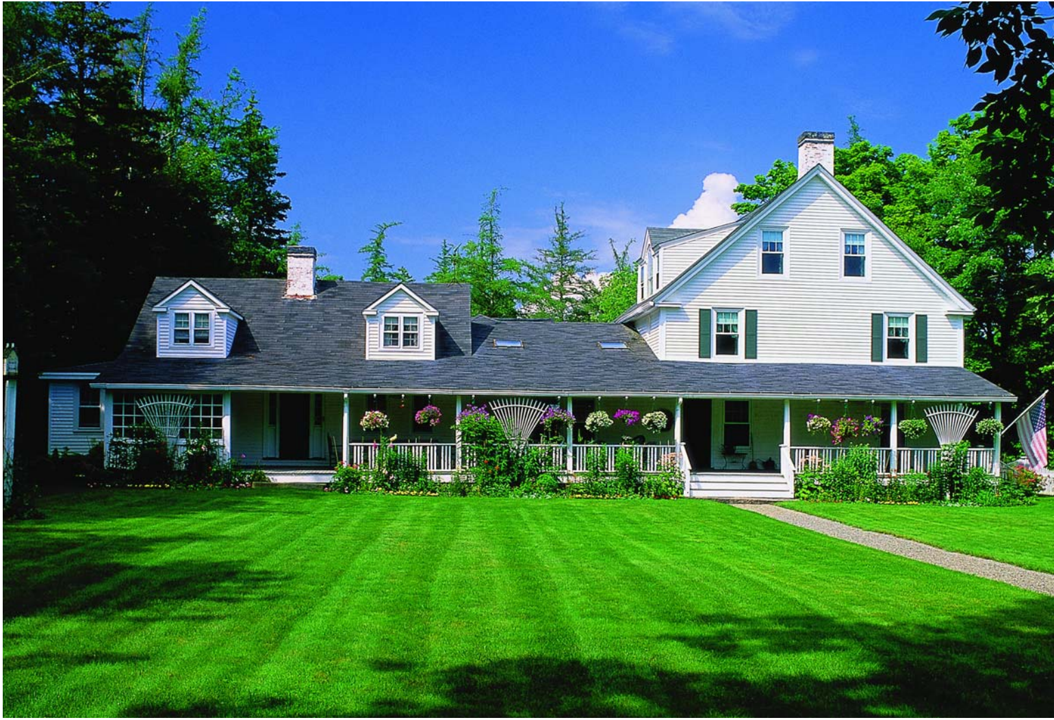
Old Homestead, Northeast Harbor, additions by Fred L. Savage, ca. 1900
