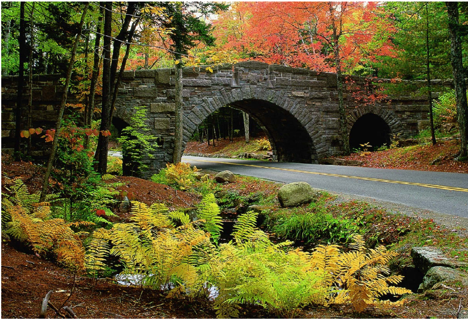
Stanley Brooke Bridge, Acadia National Park
