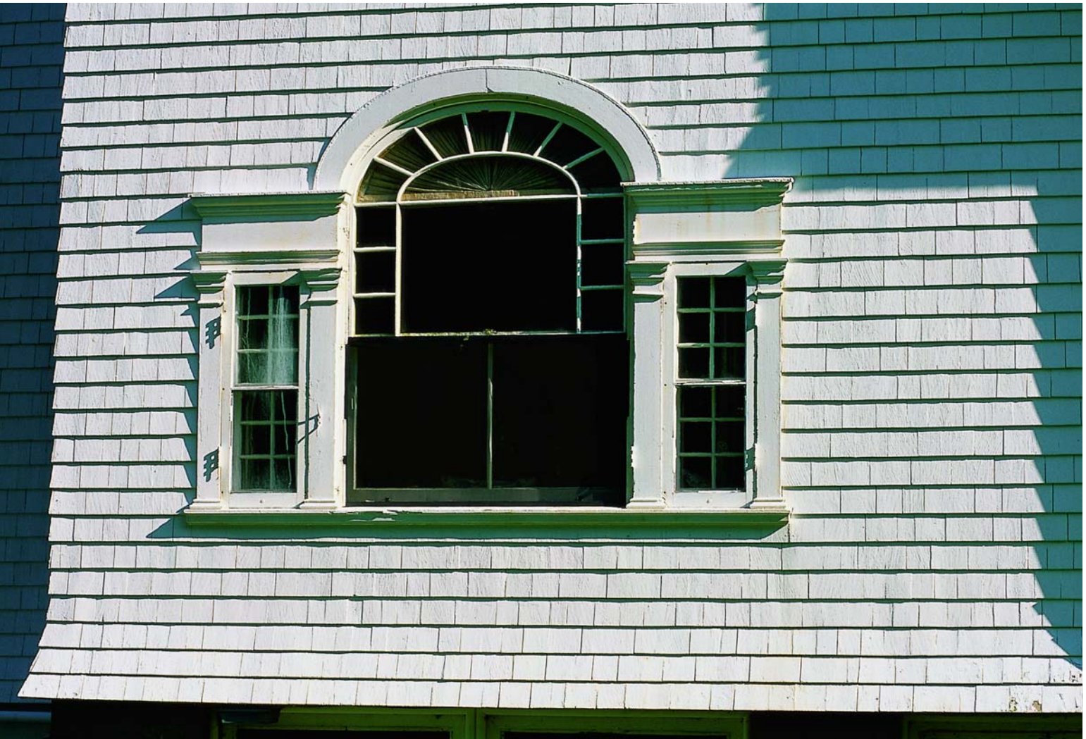
above and opposite: Reverie Cove
