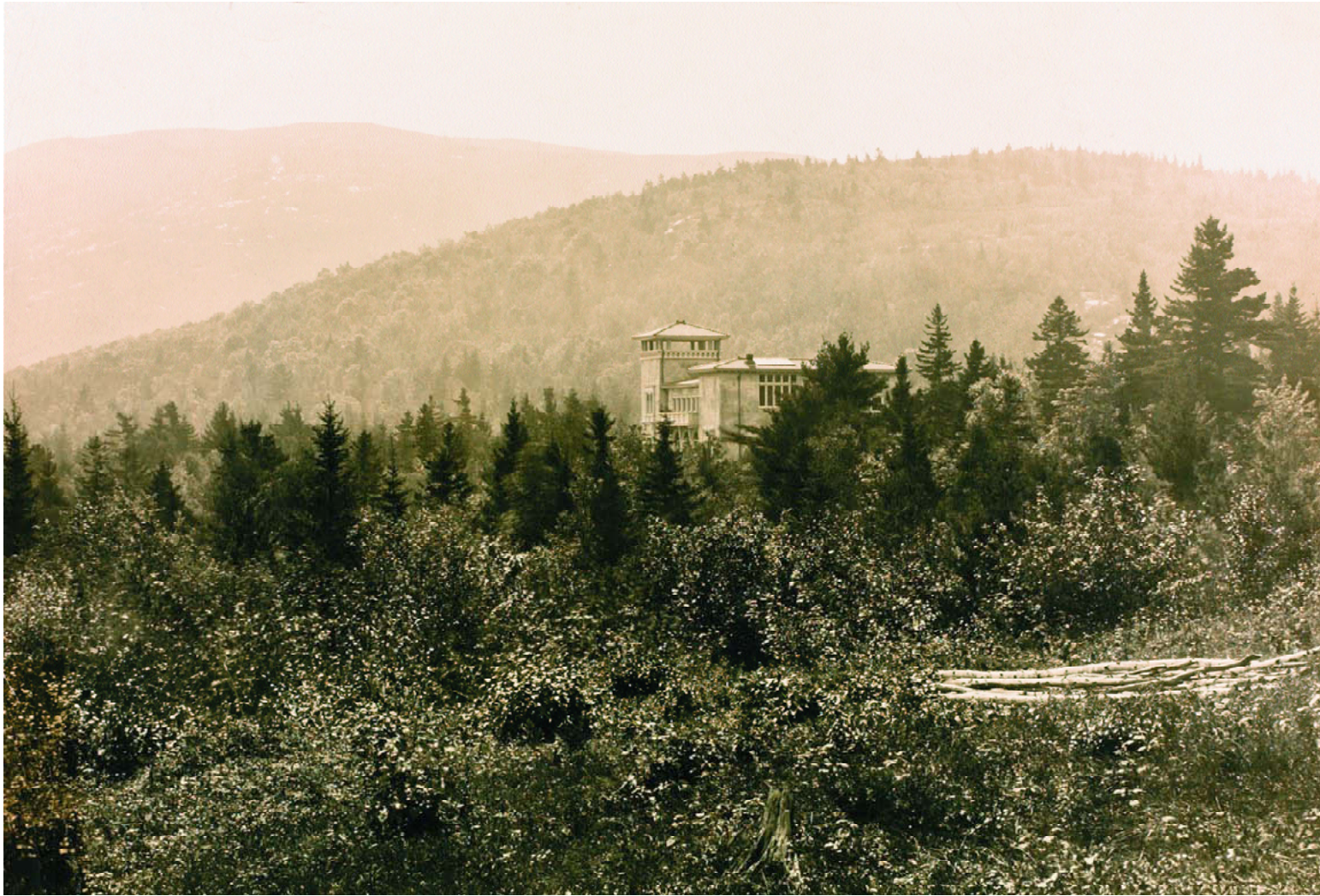
Archbold Cottage, Bar Harbor, Fred L. Savage supervising architect, 1904. Courtesy of the Bar Harbor Historical Society.
