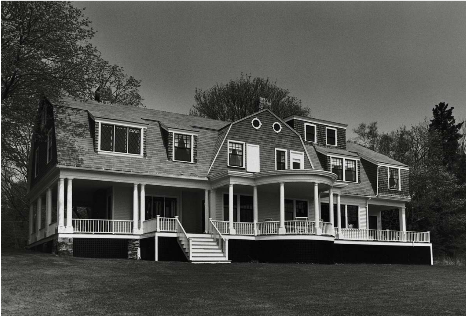
Williamson Cottage, Islesboro, Fred L. Savage, 1895. Photograph © 1989 by Richard Cheek for the Maine Historic Preservation Commission.
