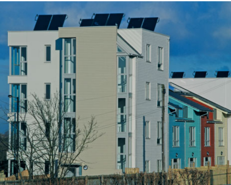
Apartment blocks are typically more muted than the houses, employing olives and khakis. However, many local residents have dubbed the scheme 'Balamory'. The parapet on the right of the image has been artificially raised, as the right-hand block is three storeys high, compared with the four-storey block on the left.
