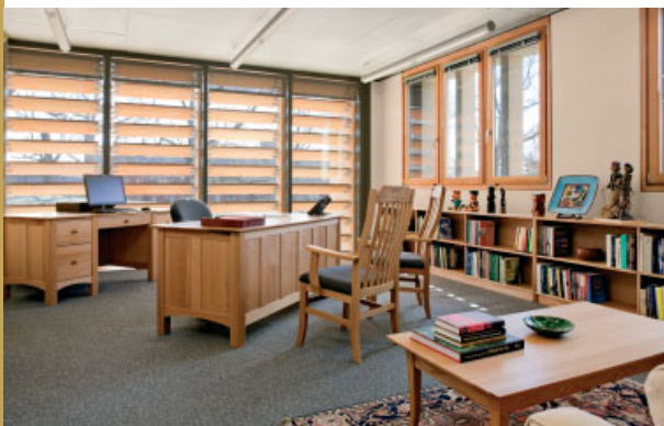
Wooden window frames, louvres and furnishings carry the decorative and symbolic generous use of wood into faculty and staff offices that occupy most of the building. Natural light is provided as well as highly efficiently fluorescent lighting that shuts off when it is not needed or when rooms are vacated.
