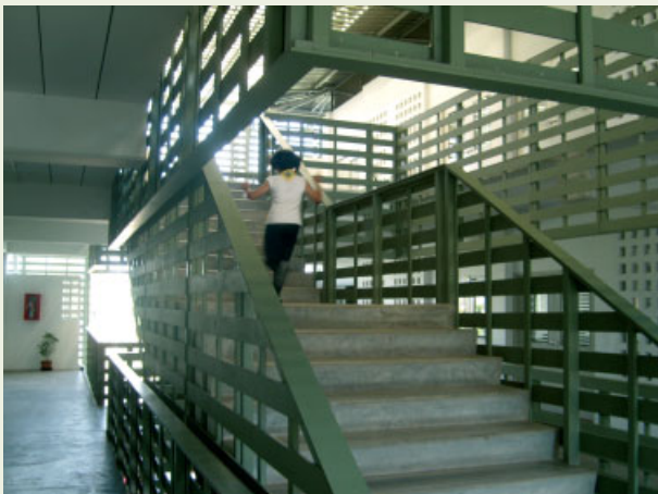
The lattice continues to wrap the interior of the dormitory atrium and becomes handrails for stairways and connecting corridors to the rooms.
