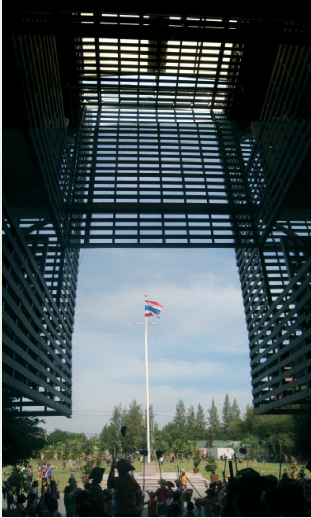
This view from within the open vestibule of the dormitory shows how effectively the lattice screens the strong tropical sun, and frames the parade grounds where the scouts assemble.
