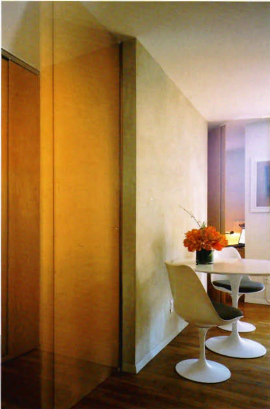
The plan shows the opening in the partition that brings more light into the study, situated in the bedroom. The sliding timber panels close off the space if necessary.
