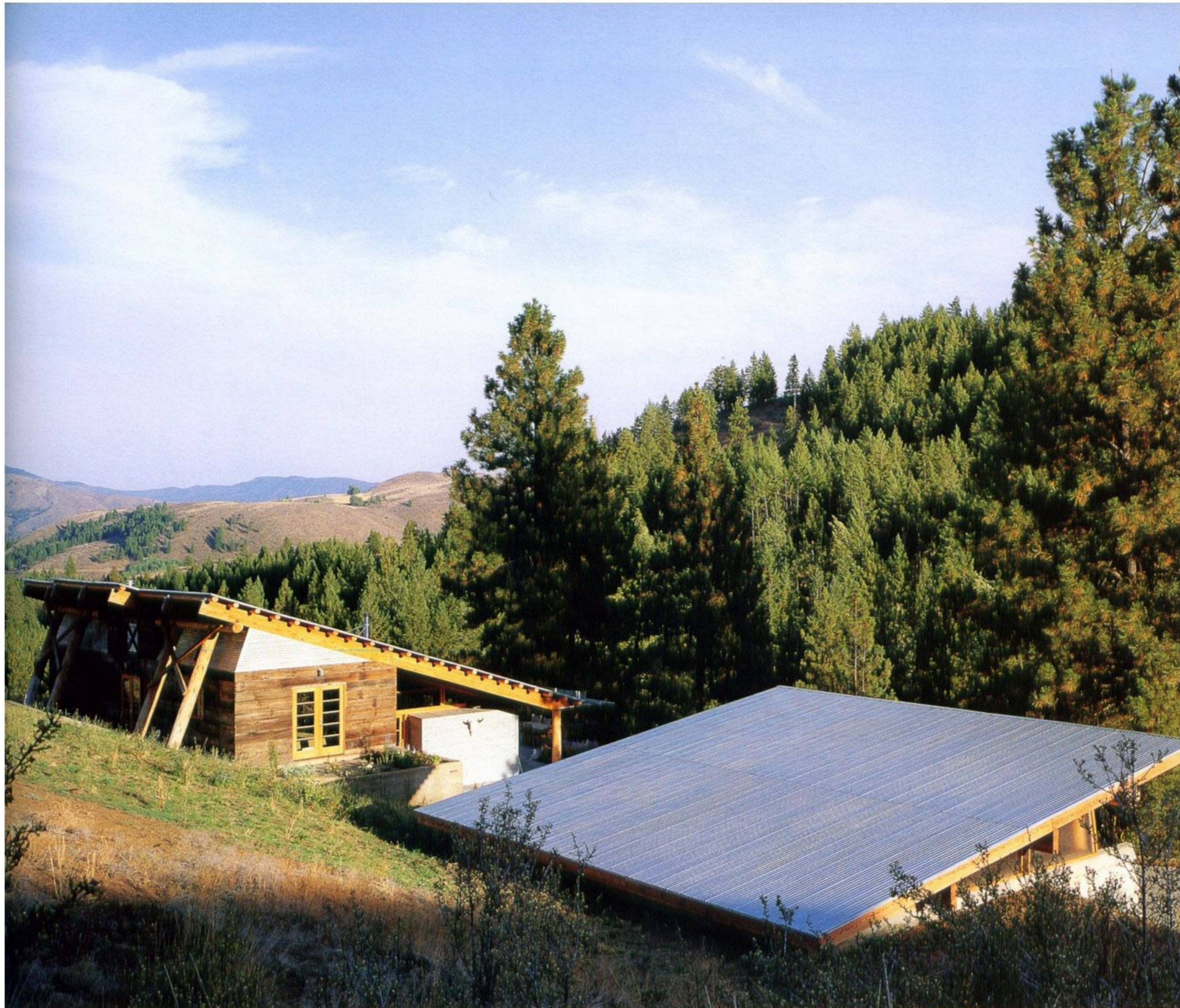
Previous pages, left, and above, views of the house and garage from various elevations, in the winter and summer.
