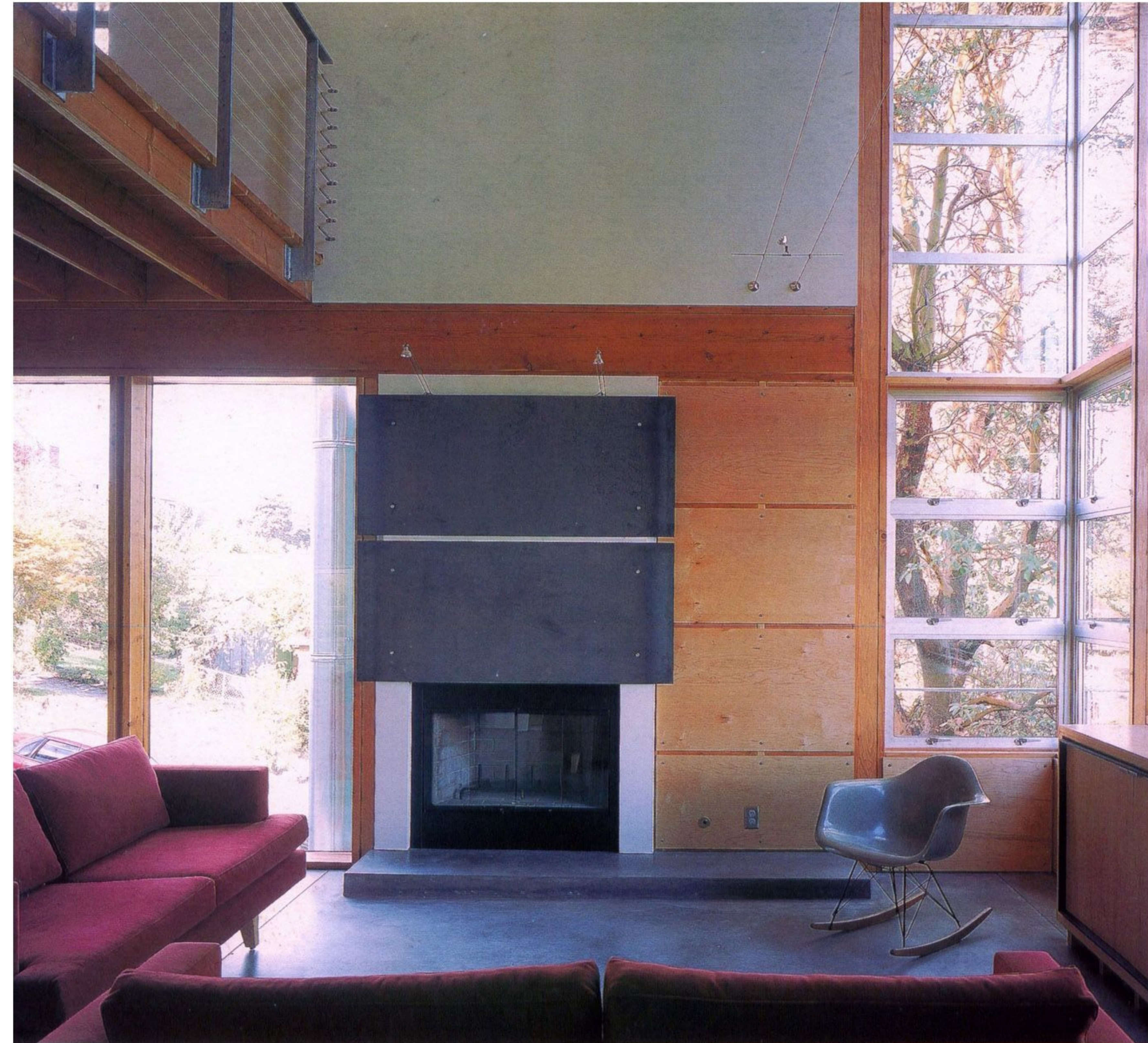
Above, steel plates slip past maple plywood panels at the living room fireplace. Right, a view of the staircase.
