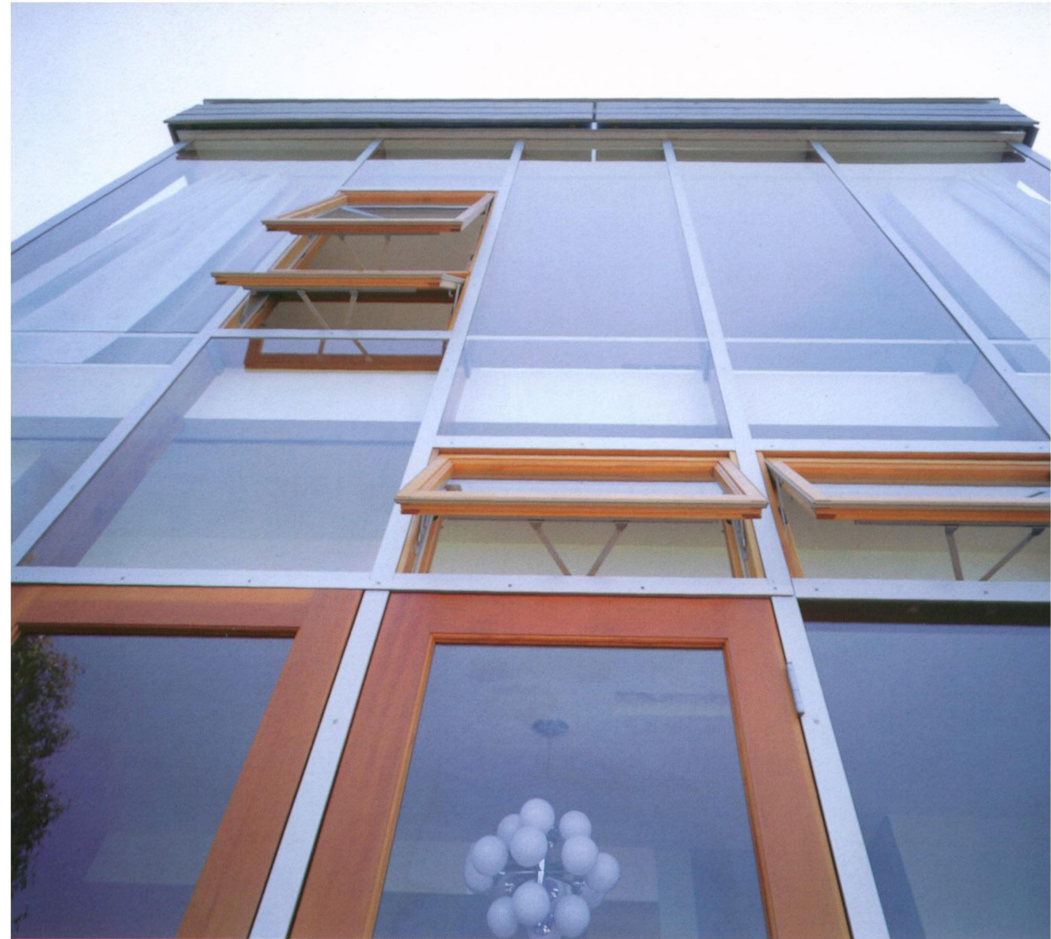
Above, the curtain wall as seen from the street. Right, an exterior detail of by 1-by-6-inch pine slats.
