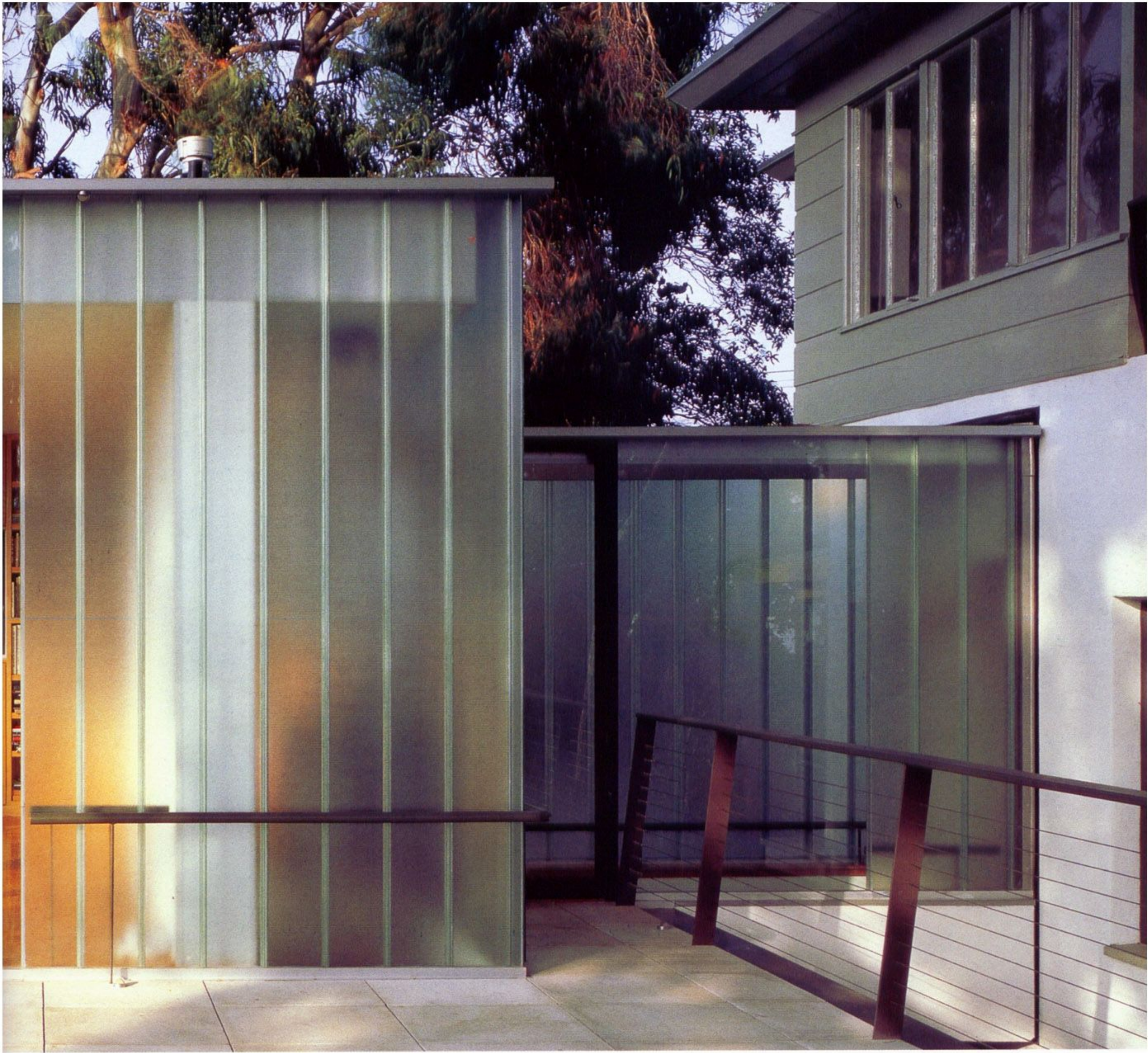
Previous pages, the bedroom wing with the roof terrace library. Above, the channel glass library with bridge to main house.
