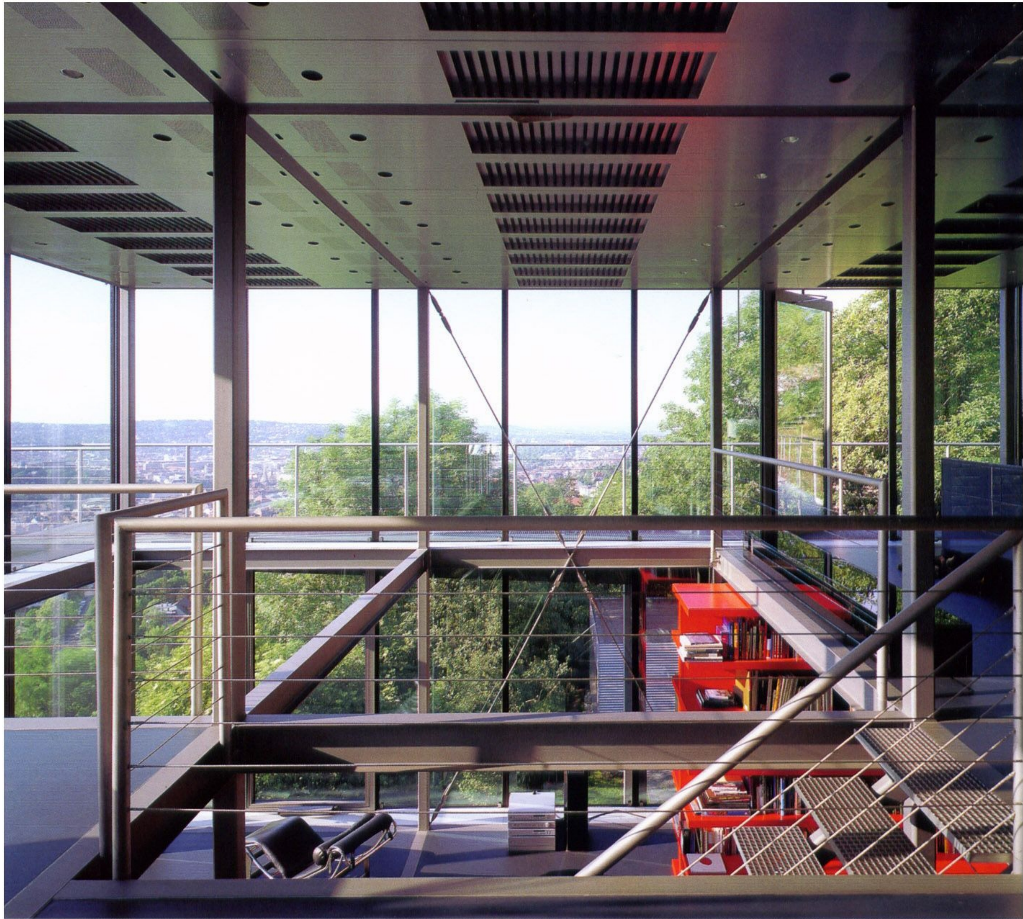
Above, a view from the top floor entrance hall with the living area below. The heating and cooling panels are visible in the ceiling. Right, a detail of the stair case.
