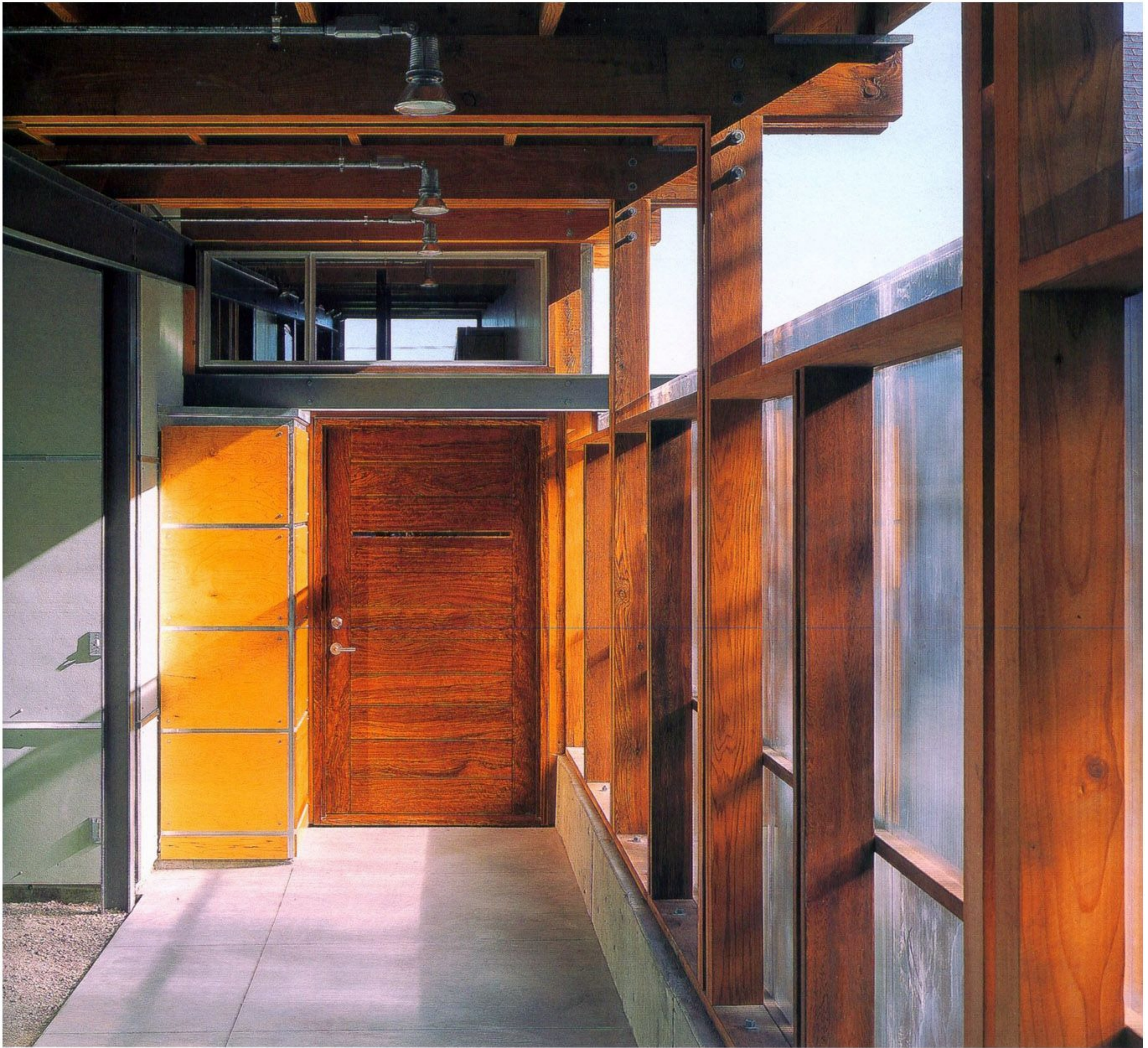
Above, the entrance as seen from the garage with polycarbonate glazing on the right allowing filtered light into the space.
