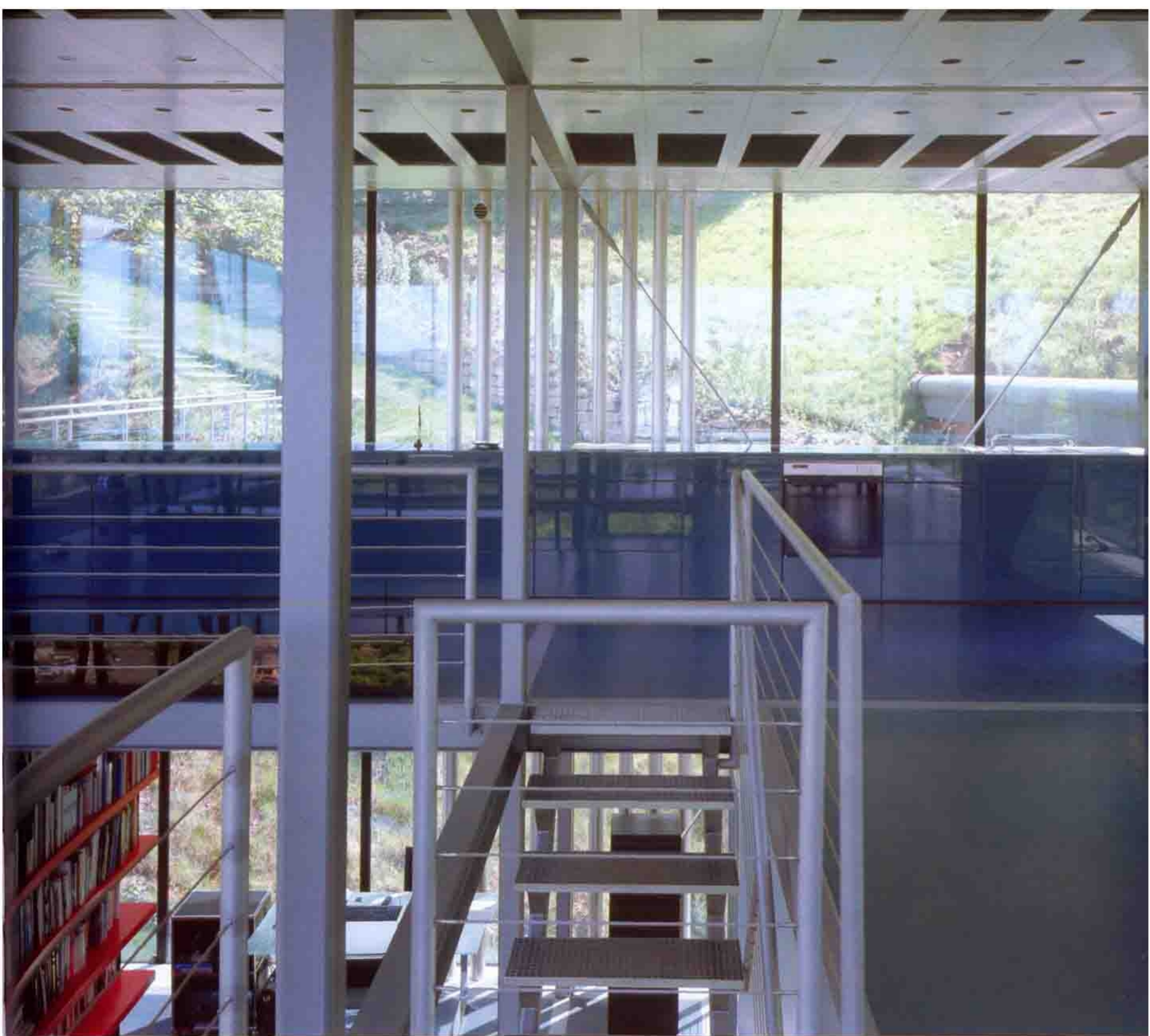
Left, each floor contains electronically controlled hinged windows of the same dimensions as the fixed glazing. Above left, a detail of the façade and loadbearing structure. Above, the kitchen.
