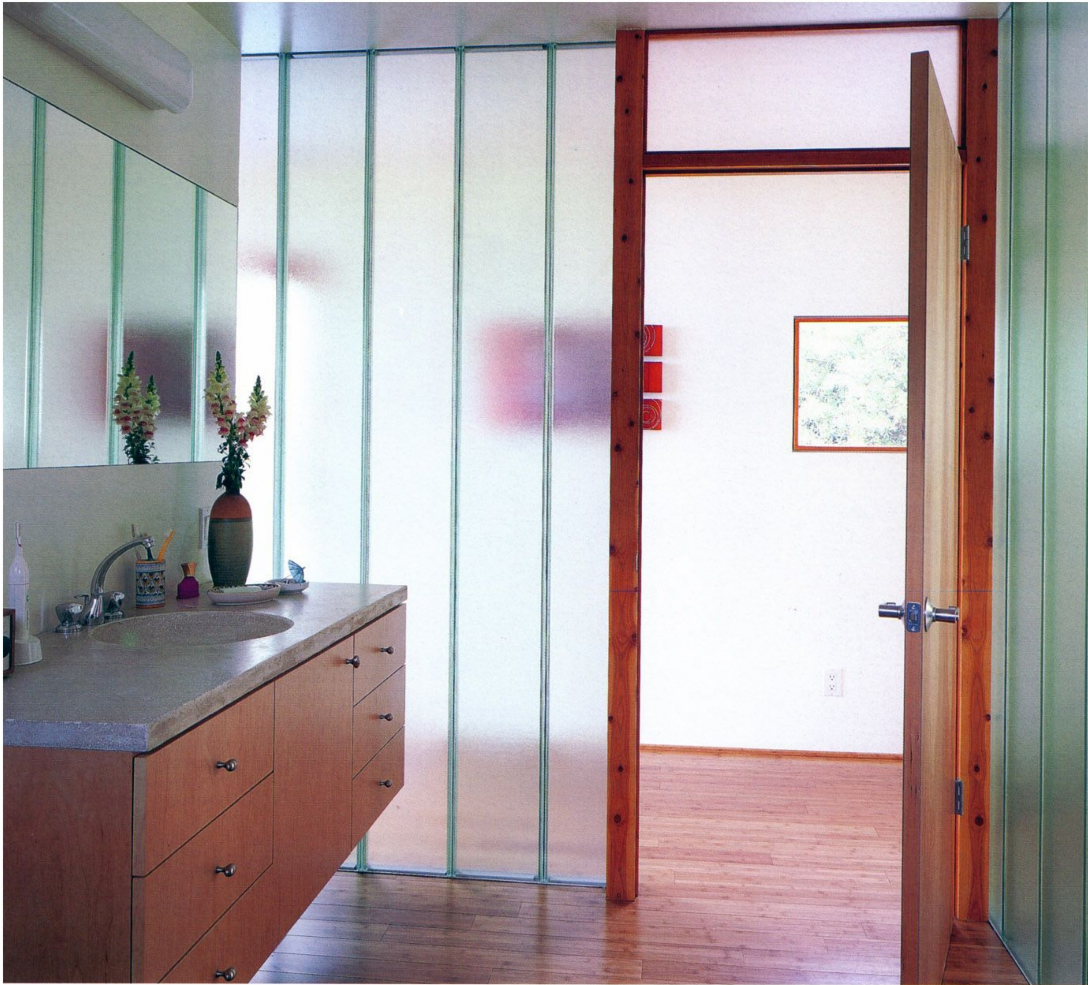
Above and right, the master bath with channel glass walls separating it from the master bedroom.
