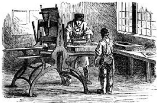
Figure 22 Lithographic press, mid 1850s.
