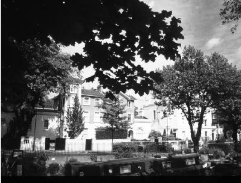
Figure 8 One of several Rural Italianate houses with towers in Little Venice, early 1840s.
