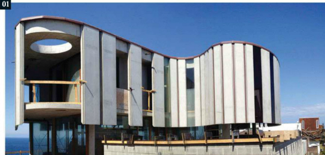
01 The Light House by Peter Stutchbury Architecture under construction. Photograph: Peter Stutchbury and James Stockwell.
