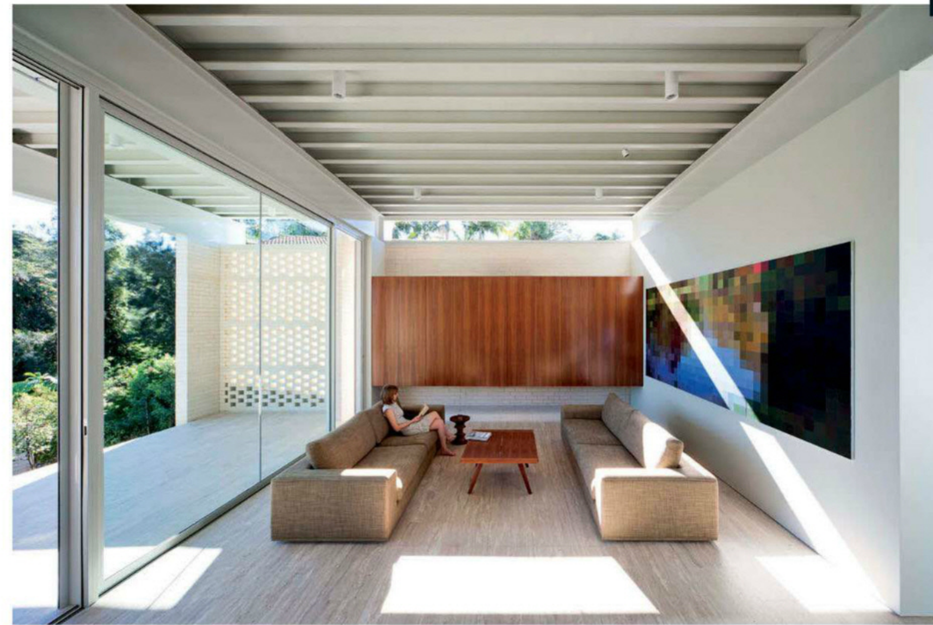
03 The deep structural elements of the roof discreetly house retractable fire shutters.
