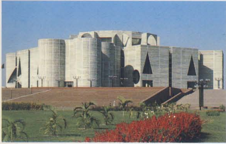
Louis Kahn Sher-e-Bangla Nagar, National Assembly, Capitol Complex Dhaka, Bangladesh, 1962–1984
