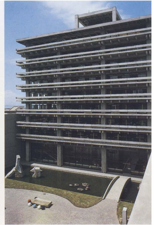
Kenzo Tange Kagawa Prefecture Takamatsu, Japan, 1955–1959 The Prefecture consists of two wings, a square building and a long horizontal structure raised on columns (shown here in part). It leaves the ground plane open allowing a clear connection to the landscape.
