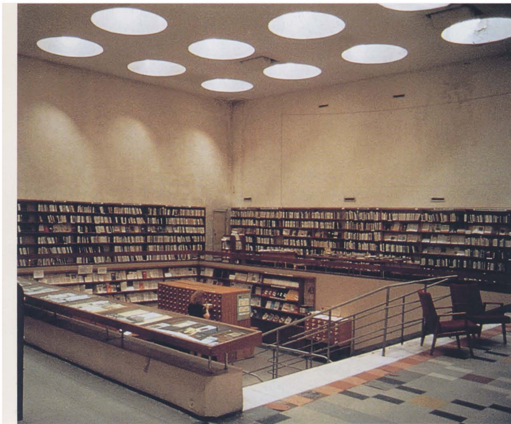
Alvar Aalto Viipuri Public Library Viipuri, Finland, 1927, 1930–1935 In general, the main block contains the library and conference rooms, while the narrower block houses the stacks and offices. The reading rooms were carefully designed to be isolated from traffic movement and noise, and were lit indirectly by funnel-shaped skylights by day, and by spotlights that bounced light off the walls by night.
