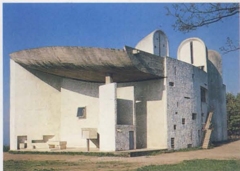
Le Corbusier Chapel of Notre-Dame-du-Haut Ronchamp, France, 1950–1955 The pilgrimage chapel, one of the architect's most published and memorable images, with its dramatic curving dark roof and white-washed concrete sculptural surfaces, is a manipulation of forms, and light and shade, which illuminates the interiors through carefully placed openings in the walls.
