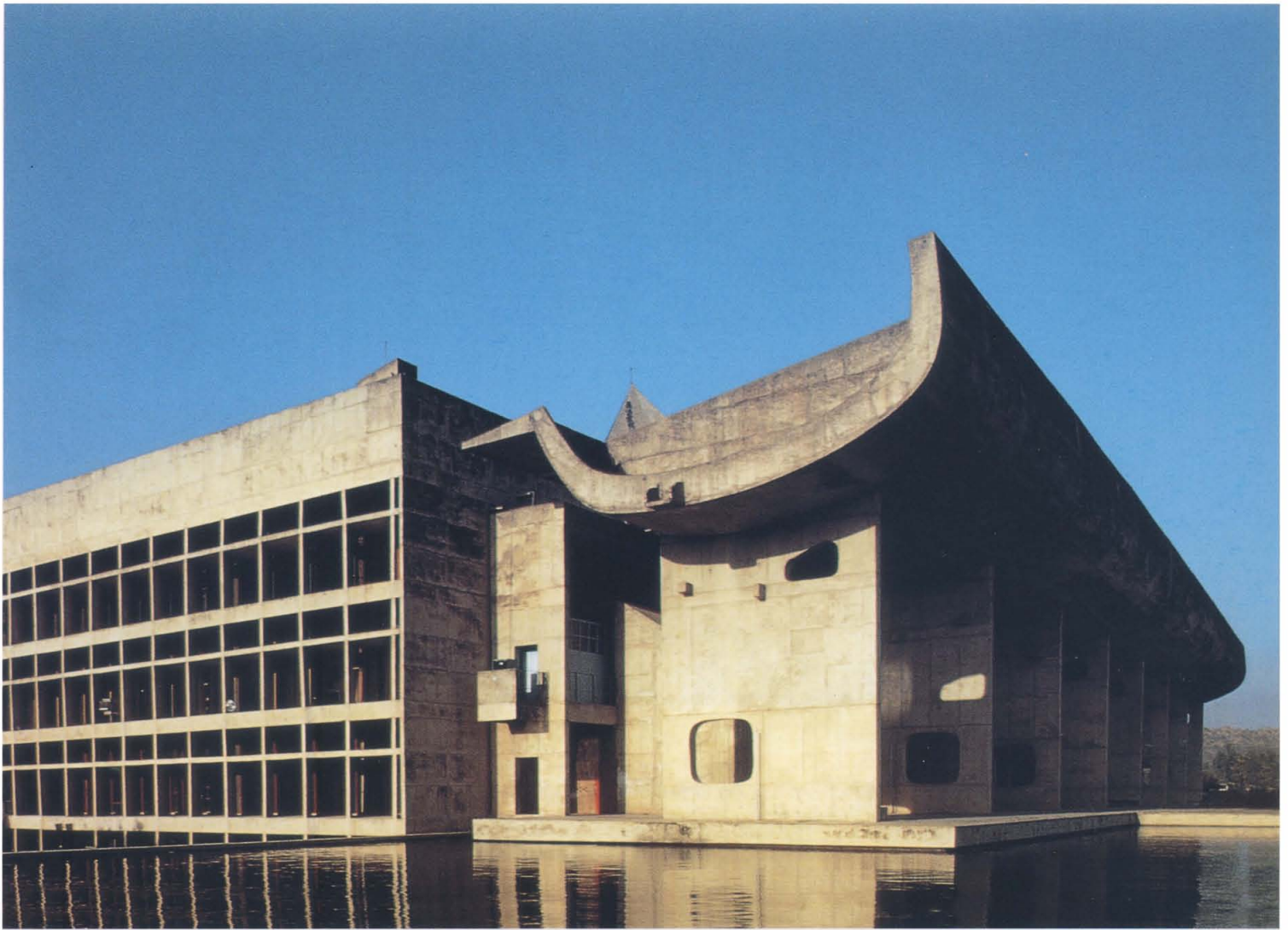
Le Corbusier Parliament or Palace of Assembly, Capitol Complex Chandigarh, India, 1951–1962 Under the dramatic roof supported by fin-like piers, the Assembly overlooks the esplanade. The attached building, to the left, houses the upper and lower chambers under sculptural shapes and surrounded by a cubic box of offices, which seems to float above the water. The great 8 m square ceremonial entrance door with its symbols of cosmic and indigenous natural forms was designed by Le Corbusier and installed in 1964.
