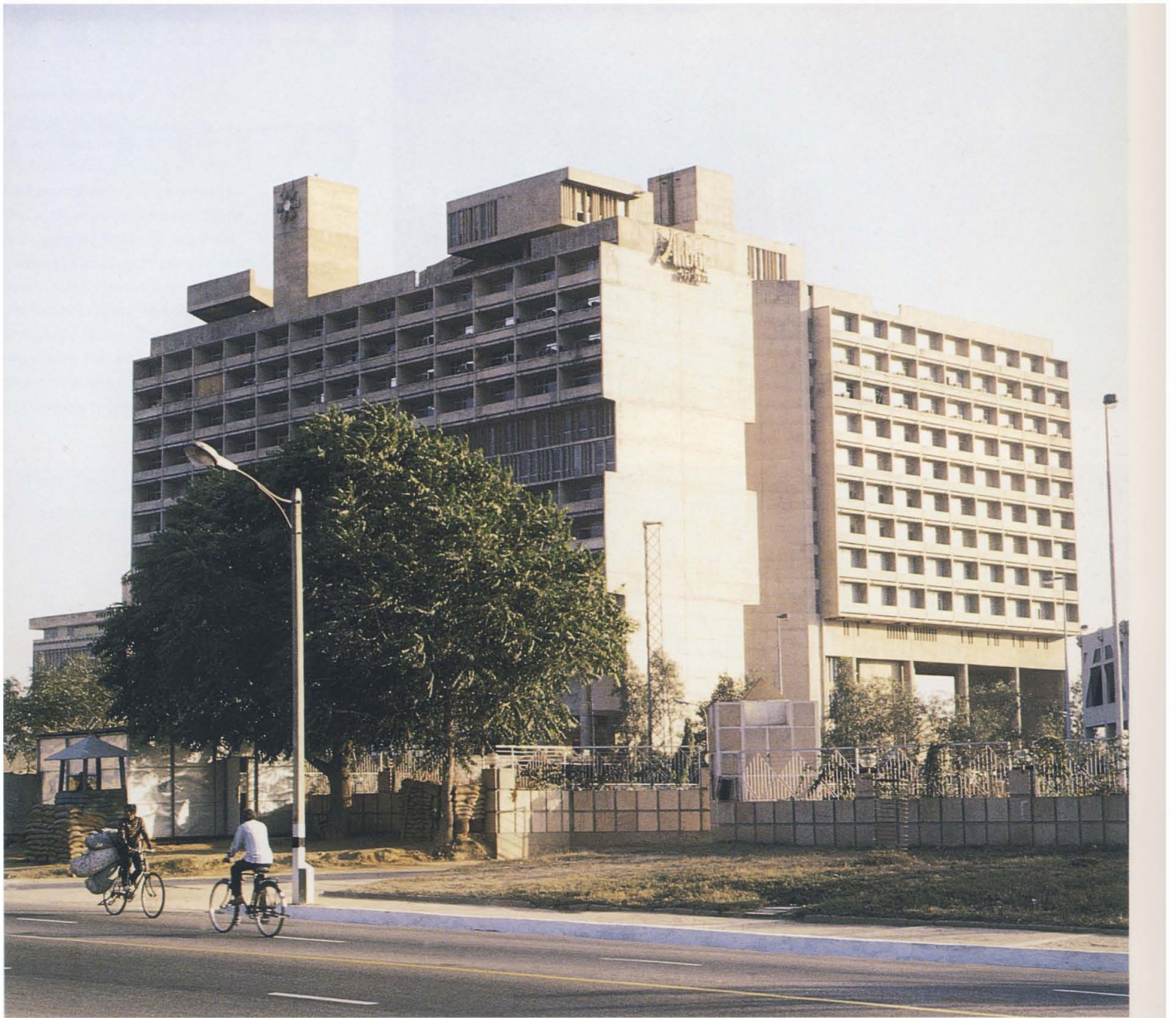
Shiv Nath Prasad Akbar Hotel New Delhi, India, 1965–69 Indebted to Le Corbusier, the modernist hotel in bare-faced concrete ( béton brut ), with deep recesses designed to respond to the Indian climate, changed the image for hotels in the country from that of Victorian to modern.
