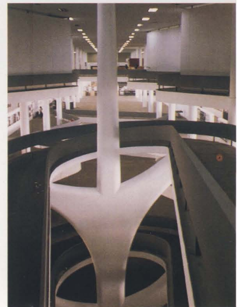
Oscar Niemeyer Interior of the Parque Ibirapuéra Exhibition Complex São Paulo, Brazil, 1951–1954 The large-scale multi-level exhibition space, with its ramps and single uniting roof, was only partially built and was substantially modified during construction.
