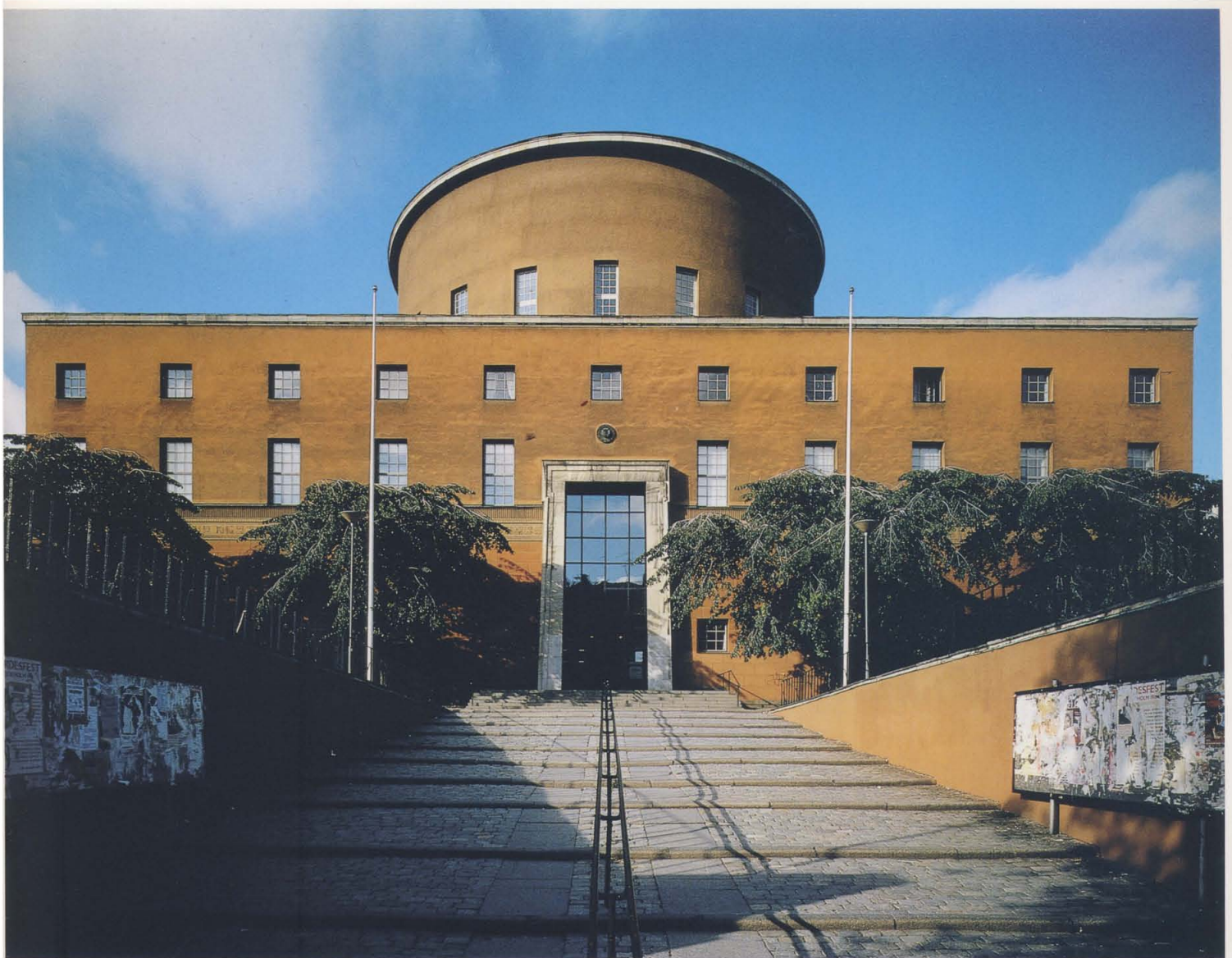
Erik Gunnar Asplund Stockholm Public Library Stockholm, Sweden, 1920–1928 Asplund's neoclassical works influenced Aalto and the Nordic modern architects. His repertoire of details, deliberately eliminating ornamentation, was used to great effect.
