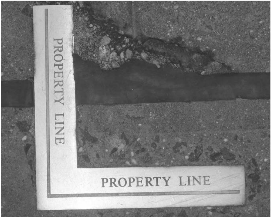
Property line marker embedded in New York City sidewalk.
