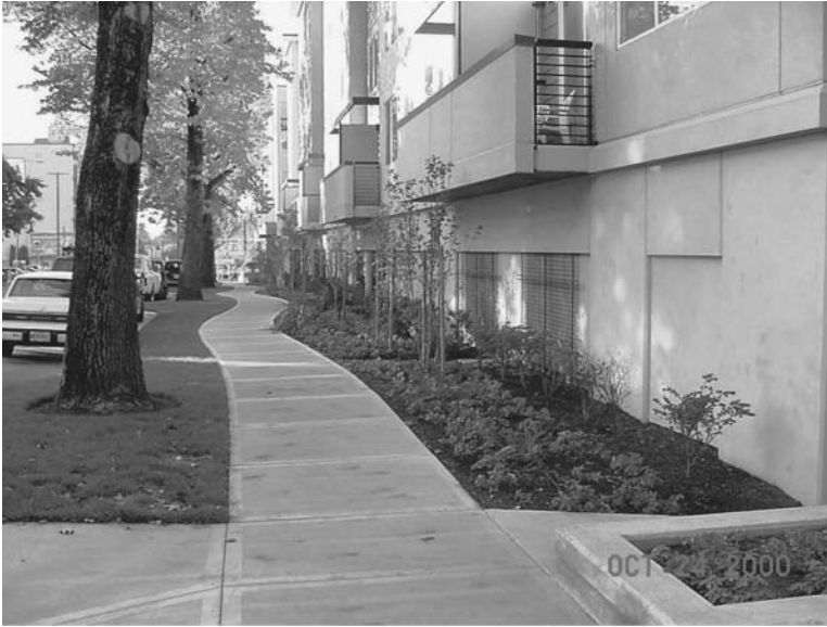
Figure I.6.15 Buckman Terrace stormwater planter at grade. (Color version available at www.gsd.harvard.edu/watercolors . Password: lentic-lotic.)
