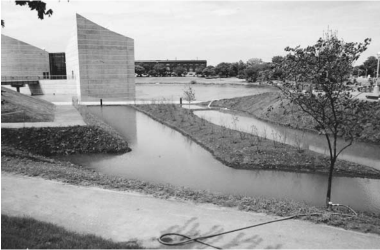
Figure I.12.2 Image of hydrological connections between the treatment wetland and reflecting pool. Water from the latter enters the wetland through the right channel, swings around the central berm, and then exits back to the pool via the large channel in the middle of the photograph. Note how the building seems to “float” on the water of the reflecting pool and river. (Color version available at www.gsd.harvard.edu/watercolors . Password: lentic-lotic.)
