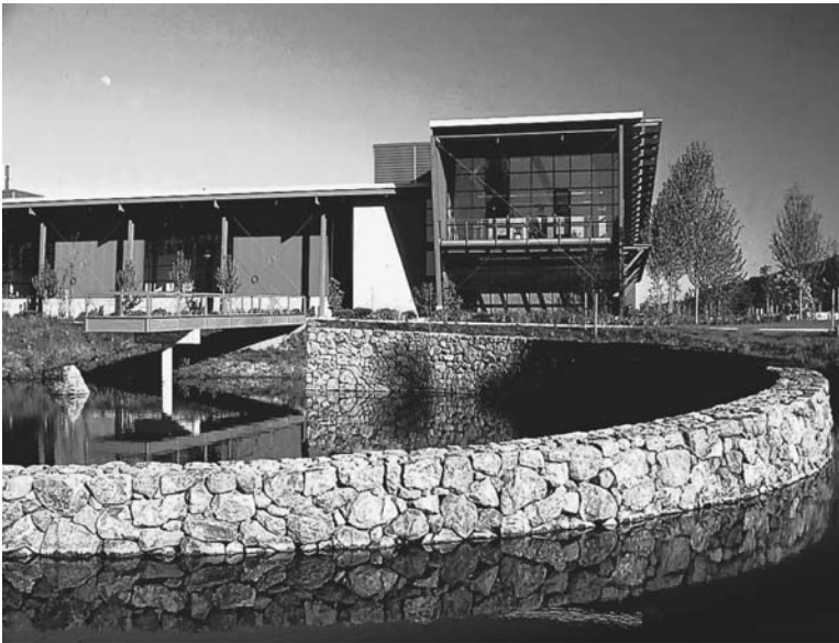
Figure I.6.26 Water garden stone wall outlet structure. (Color version available at www.gsd.harvard.edu/watercolors . Password: lentic-lotic.)
