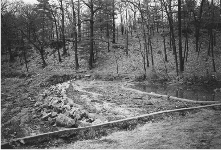
Figure I.11.19 Earthen berm separates the stilling basin from Hill's Pond. (Photo by Clarissa Rowe.)
