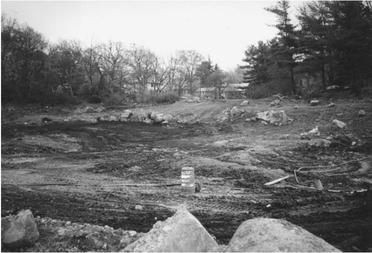
Figure I.11.14 Hill's Pond fully dredged. (Photo by Clarissa Rowe.)
