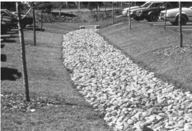
Figure I.1.13 Swale at a Merrill Lynch training office near Princeton, NJ. (Color version available at www.gsd.harvard.edu/watercolors . Password: lentic-lotic.)
