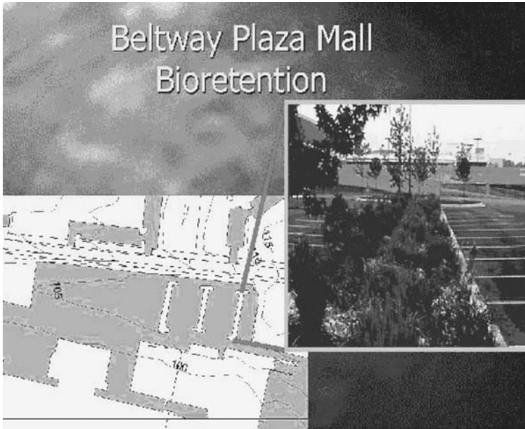
Figure I.15.3 Beltway Plaza Bioretention Site illustrates how the impervious areas from this shopping center expansion were effectively disconnected and treated by designing the landscape islands as bioretention cells. (Color version available at www.gsd.harvard.edu/watercolors . Password: lentic-lotic.)
