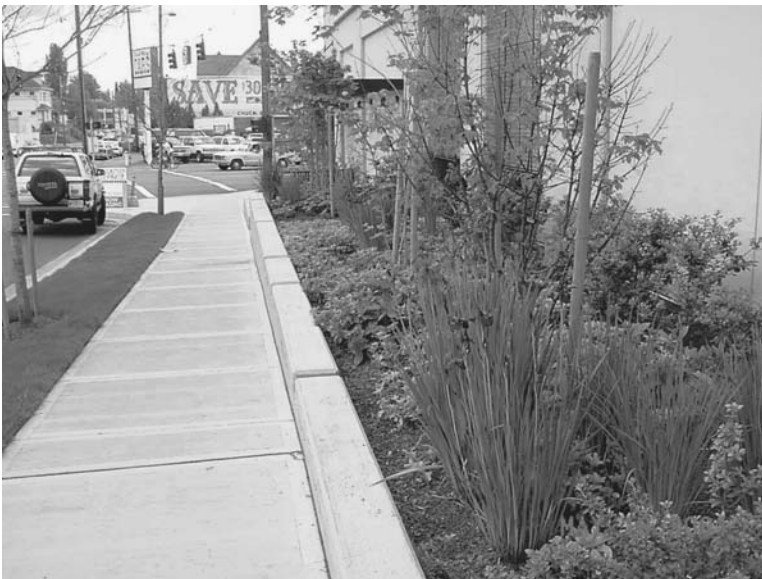
Figure I.6.16 Buckman Terrace raised stormwater planters. (Color version available at www.gsd.harvard.edu/watercolors . Password: lentic-lotic.)
