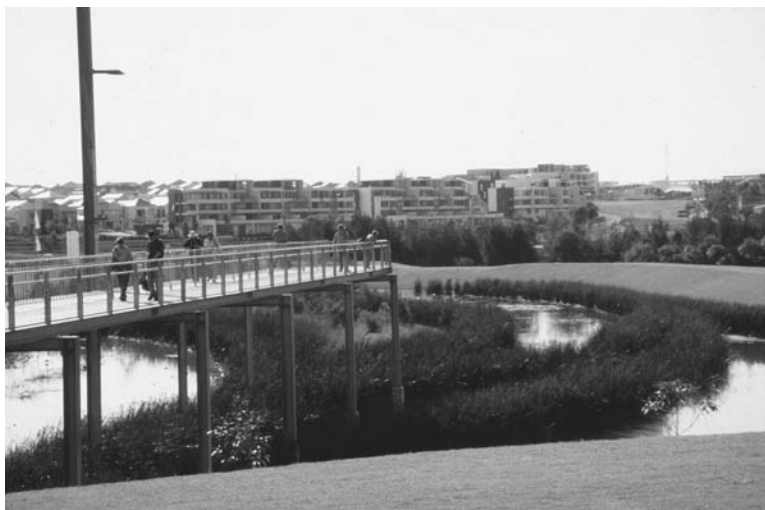
Figure I.13.9 Created Wetland Ponds, showing curvilinear “fingers” of macrophytes and open water areas. (Courtesy of Hargreaves Associates.)
