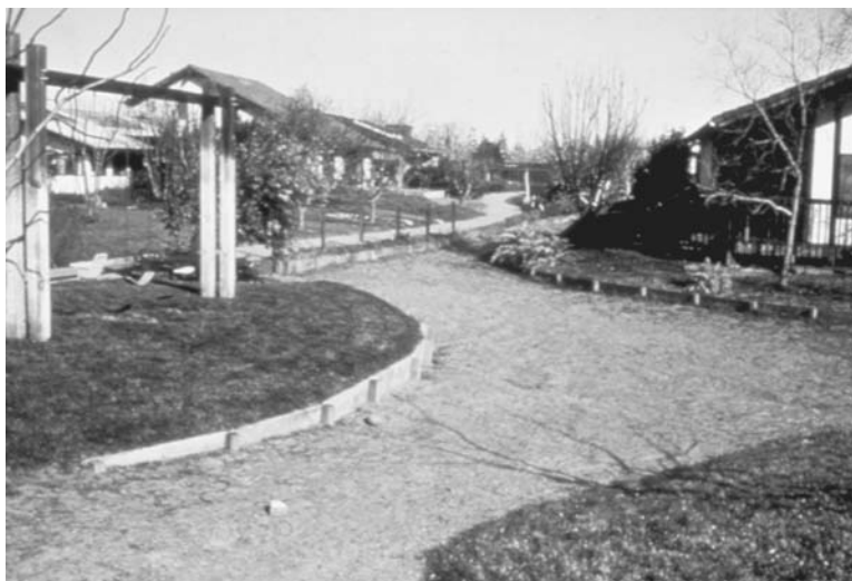
Figure I.1.14 Infiltration basin doubling as a playground at Village Homes, Davis, CA. (Photograph by Roger D. Moore.) (Color version available at www.gsd.harvard.edu/watercolors . Password: lentic-lotic.)
