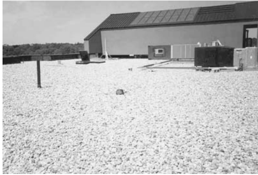
Figure I.2.3a Ballast roof, Milton, MA.
