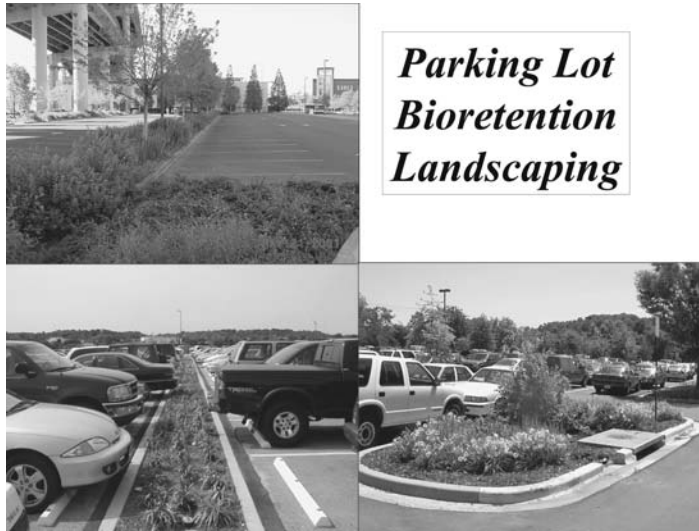
Figure I.5.10 Examples of parking lot bioretention (rain gardens).
