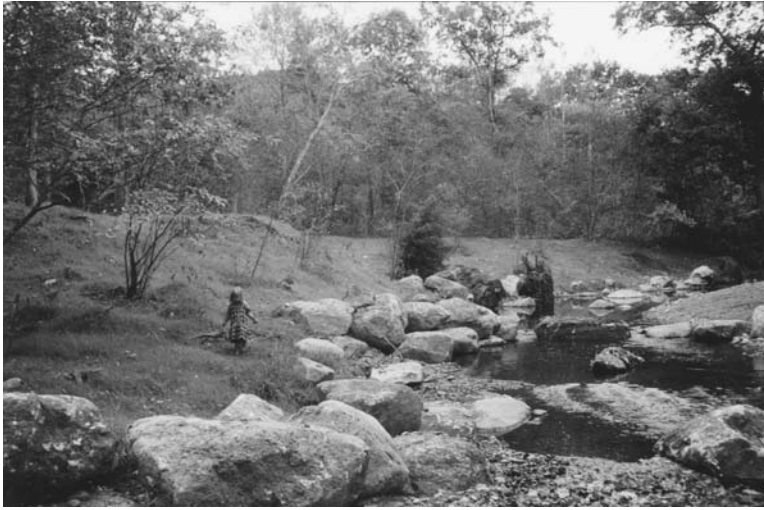
Figure I.17.1 Merrick Brook, Scotland, CT. Newly realigned channel with bank stabilization using root wads and native plantings, plus in-stream enhancements using boulder weirs.
