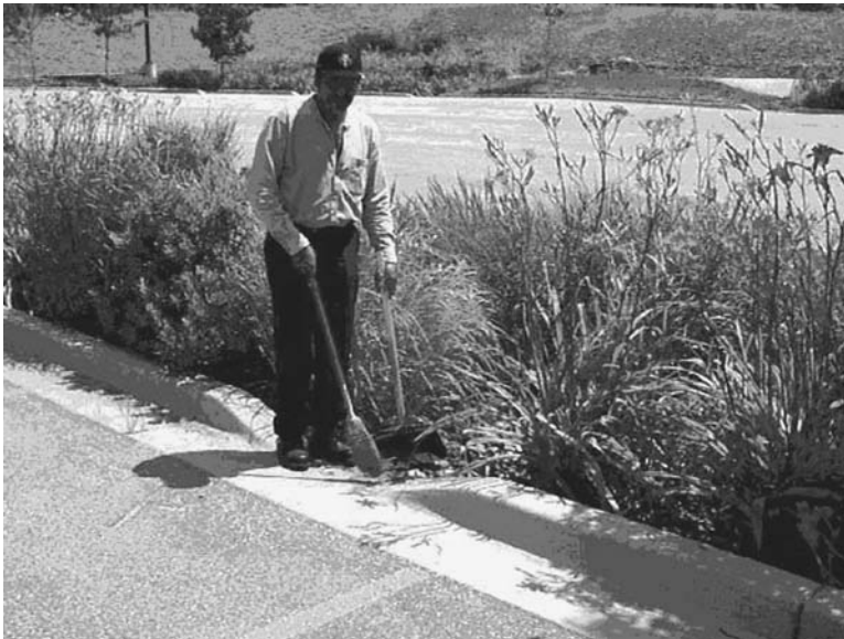
Figure I.15.4 Beltway Plaza bioretention cells. The reported maintenance costs of bioretention cells is low, averaging approximately $200/site. (Color version available at www.gsd.harvard.edu/watercolors . Password: lentic-lotic.)
