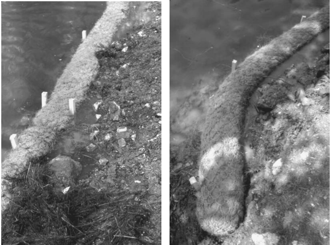
Figure I.16.12 Installation of biologs.
