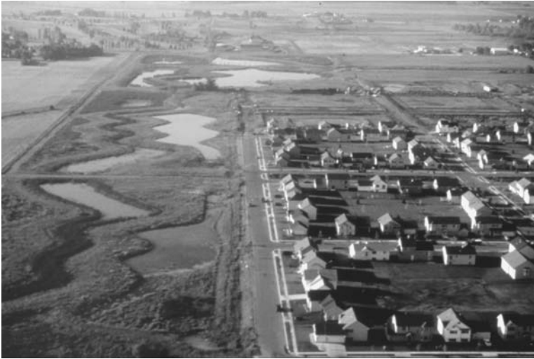
Figure I.8.9 View of the third stage of the Park Place housing development with water system. (Photo by Design Center for American Urban Landscape. © Copyright Balmori Associates.) (Color version available at www.gsd.harvard.edu/watercolors . Password: lentic-lotic.)
