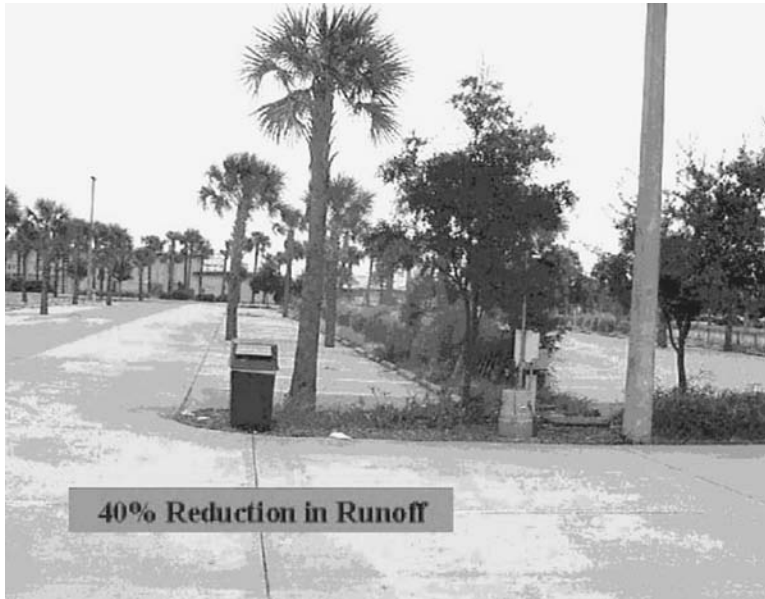
Figure I.15.13 Florida Aquarium site monitoring stations. Porous pavement and bioretention strips help achieve a 40% reduction in runoff. (Color version available at www.gsd.harvard.edu/water-colors . Password: lentic-lotic.)
