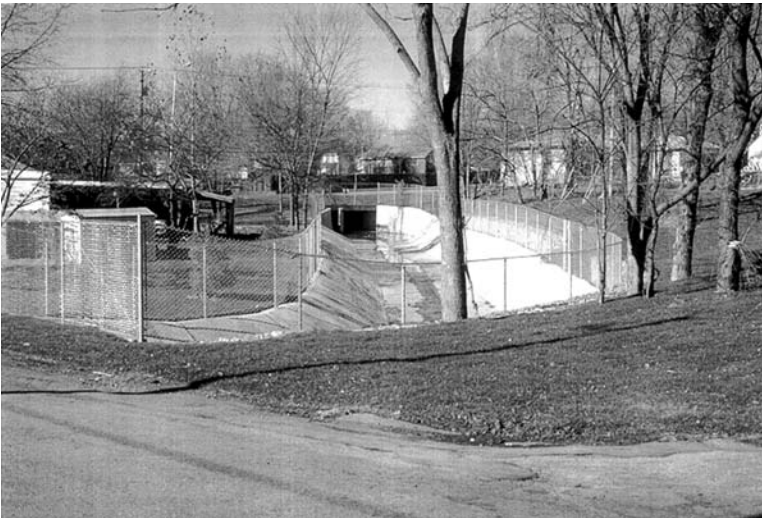
Figure II.8.6 A typical concrete-lined channel storm drainage project located in Overland Park.
