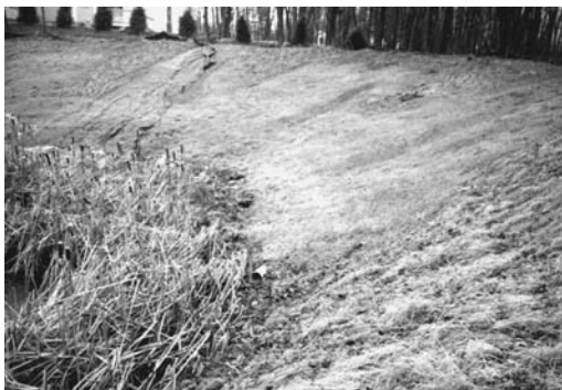
Figure I.2.4d Slope in Figure I.2.4c after restoration.
