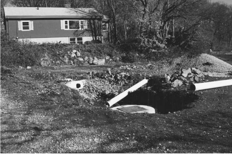
Figure I.11.10 Vortech Box installation at Hill's Pond. (Photo by Clarissa Rowe.)
