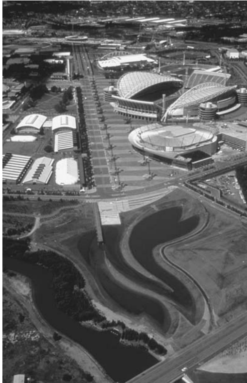
Figure I.13.2 Aerial view of the Northern Water Feature with Olympic Plaza beyond. (Photo by Olympic Coordination Authority. Courtesy of Hargreaves Associates.)
