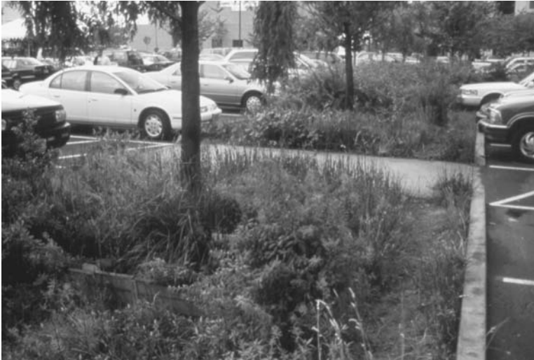
Figure I.1.12 Infiltration swale at the Oregon Museum of Science and Industry in Portland. (Color version available at www.gsd.harvard.edu/watercolors . Password: lentic-lotic.)
