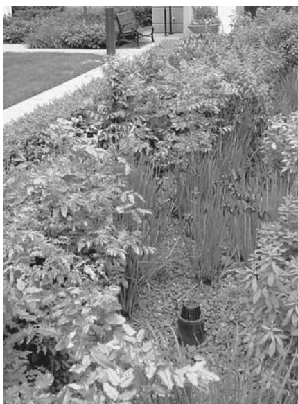
Figure I.6.8 Buckman Heights courtyard infiltration garden, with outlet riser. (Color version available at www.gsd.harvard.edu/watercolors . Password: lentic-lotic.)
