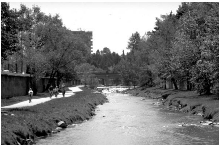
Figure II.3.3 Denver flood channel/greenway, Denver, CO, has transformed several of its urban streams into multiobjective stormwater management, transportation, and recreational corridors. (Photo by Charles Flink.)
