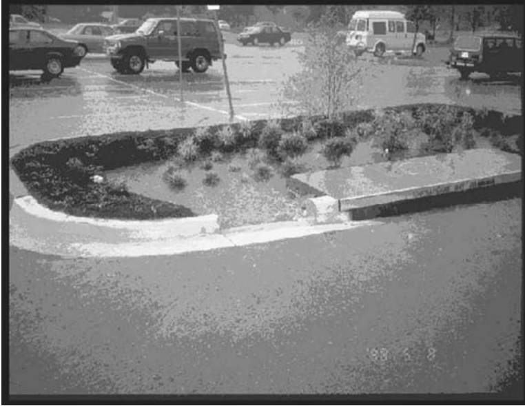
Figure I.15.6 Operation of bioretention cell during a storm — curb cuts intercept and direct runoff into the bioretention cell for storage and treatment. (Color version available at www.gsd.harvard.edu/watercolors . Password: lentic-lotic.)
