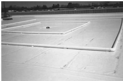
Figure I.2.3b Water dam roof detention, Mansfield, MA.
