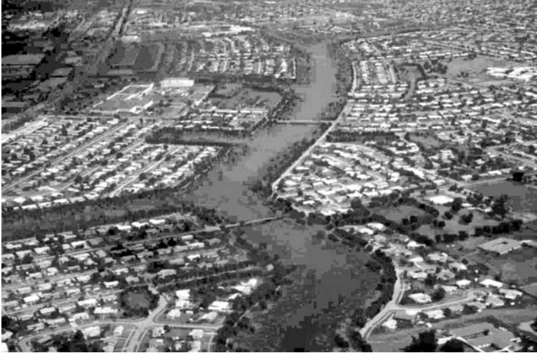
Figure II.11.8b The wetlands have been reclaimed, improving flood protection, adding open space, and increasing property value.
