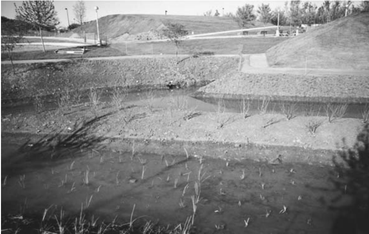
Figure I.12.4 Newly planted wetland showing the importance of grading to plant survival. (Color version available at www.gsd.harvard.edu/watercolors . Password: lentic-lotic.)
