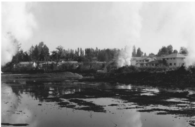
Figure I.9.3 Site during construction. Extensive removal of material was required for stormwater storage. (Photo by Catherine Berris Associates.) (Color version available at www.gsd.harvard.edu/watercolors . Password: lentic-lotic.)
