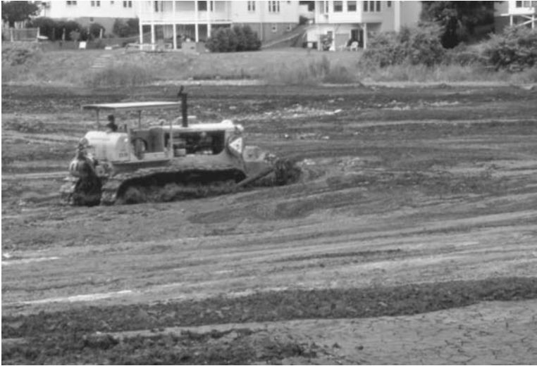
Figure I.16.3 Dredging operations at Chandler Pond in summer 1999.
