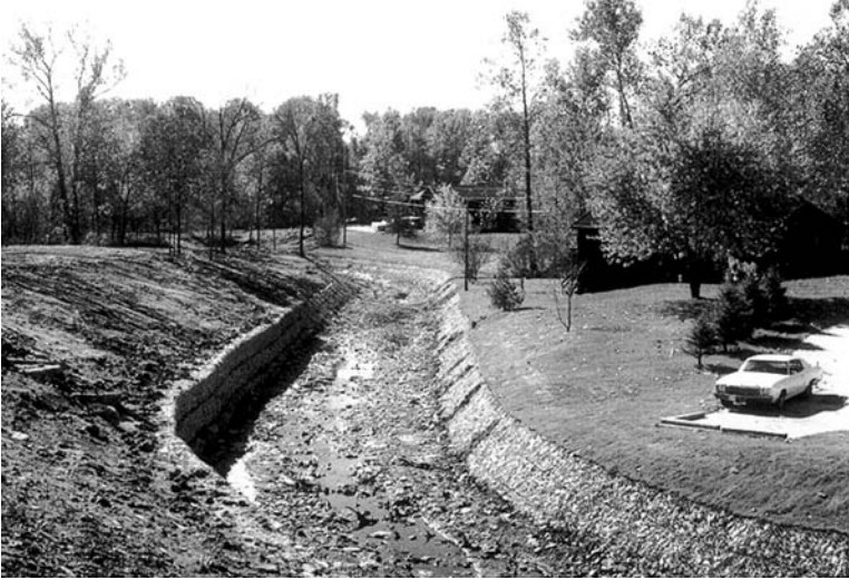
Figure II.8.5 A typical gabion basket storm drainage project located in Lenexa, KS.
