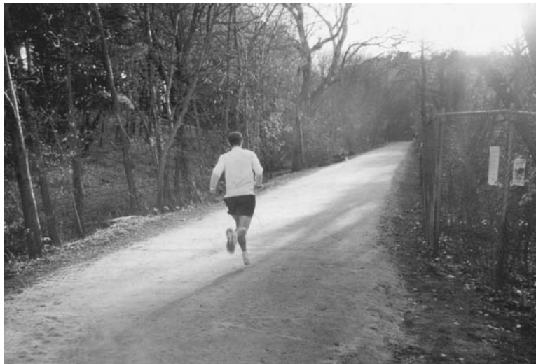
Figure II.4.17 Pilot section of stabilized aggregate Perimeter Road resurfacing. Stabilized aggregate surface is porous, natural in appearance, and easy on the feet. Stabilized aggregate acts as a “sponge” when wet preventing runoff into the reservoir.
