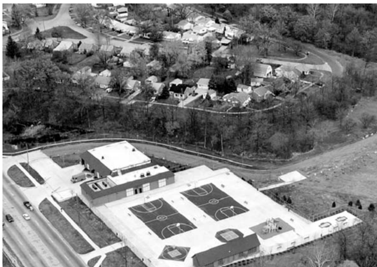
Figure II.9.4 Aerial view of Inkster combined sewer overflow basin in Rouge River Watershed, Inkster, MI. (Courtesy of Rouge River National Wet Weather Demonstration Project, Detroit.)
