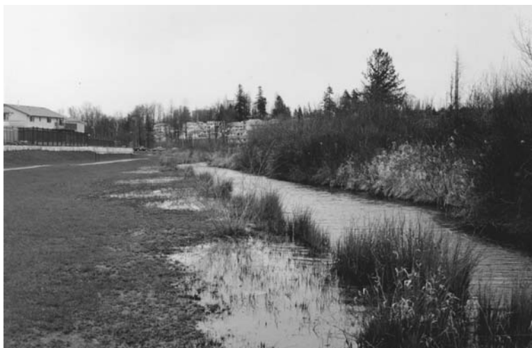
Figure I.9.2 Small park area near creek prior to construction. Note mowed grass park, walkway, and flooding of creek. (Photo by Catherine Berris Associates.) (Color version available at www.gsd.harvard.edu/watercolors . Password: lentic-lotic.)
