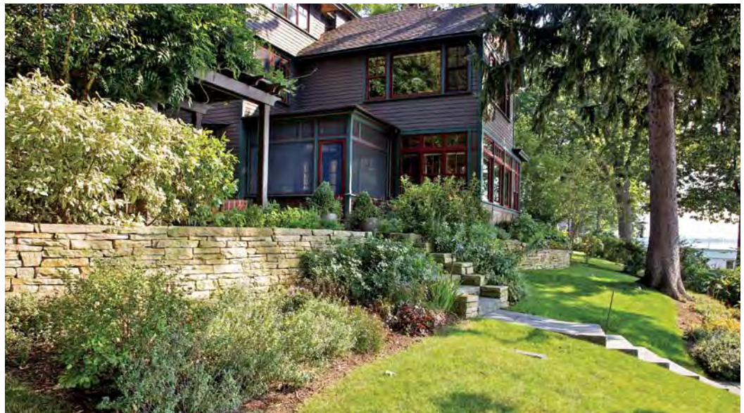
above • A softly curving retaining wall forms one of the terraces that turns this steep slope into usable living space.
