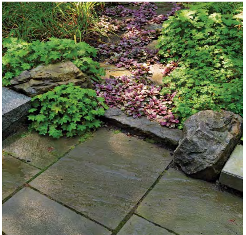
above • Both the natural and quarried version of Pennsylvania bluestone are used to handsome effect in this garden. The cut bluestone walkway edged by granite gives way to a flat fieldstone path.
