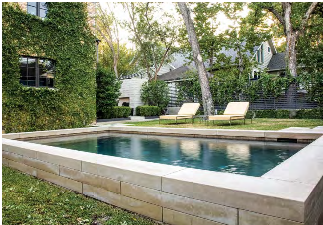
Swim spas are small pools built for exercising against an artificially generated current. This pool is set into a freestanding limestone wall that supports a small raised terrace area.
