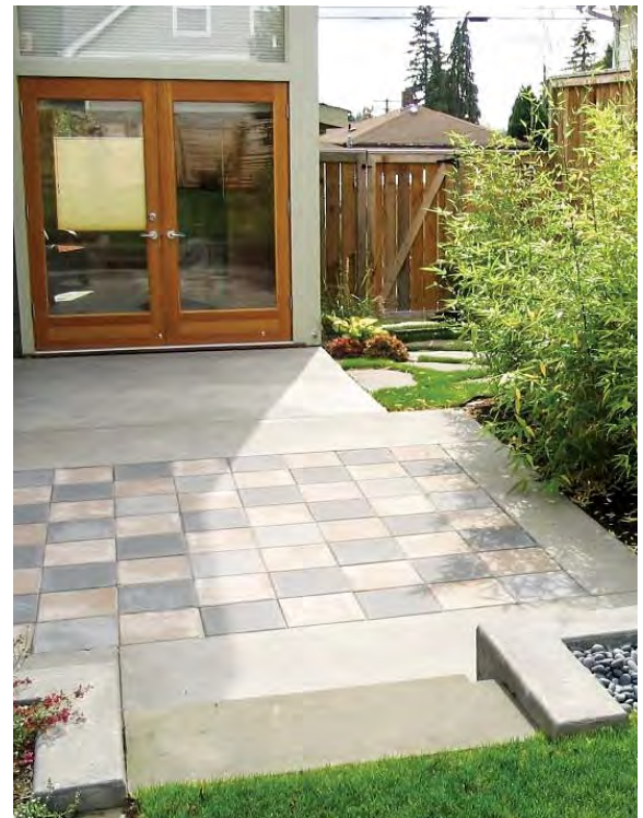
CAST-IN-PLACE AND TINTED CONCRETE PAVERS
