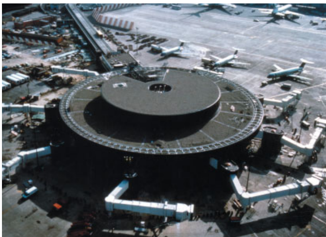
YRM, Gatwick Airport, South Terminal, 1985.
