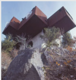
Kisho Kurokawa, Capsule 'K' Summer House, Nagano, 1973 This project, in Corten steel rather than concrete, as at Nakagin, or stainless steel at Sony, is clustered as a number of rooms around a site-built core.
