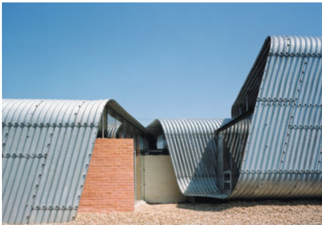
Shuhei Endo, 'Springecture' B, Shiga prefecture, Japan, 2002 On the southern facade, the corrugated-steel sheeting is wrapped in a spiralling form on an east-west axis, and earthquake-resistant brick walls cover the openings.
