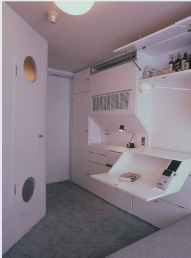
Kisho Kurokawa, Nakagin Capsule Tower, Tokyo, 1972 Kisho Kurokawa in front of the tower in 1972. All the utilities, fittings and appliances for the interior – including the TV – were installed in the factory, an approach that raises the question of design life and upgrade.
