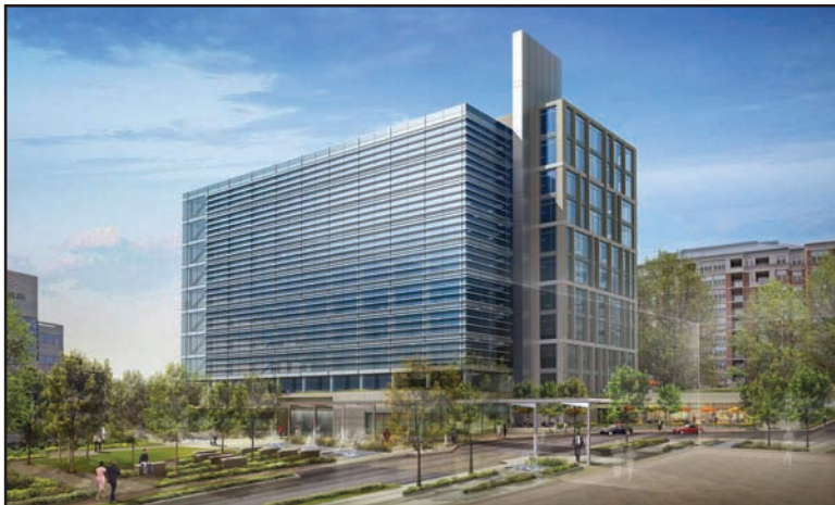
Reston Heights, Reston VA Owner: The JBG Companies, Architect— HOK; Washington, DC MEP Engineers— R.G. Vanderweil; Boston, MA
