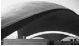
12.4 >Isler's shell for the Deitingen gas station was derived from the shape of a hanging fabric. The same formwork could be used for both shells.
