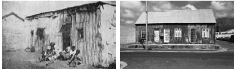
16.3 >Left: Corrugated-iron dwelling at the periphery of the city. Right: 1920s Municipal sponsored corrugated-iron dwelling in Athlone, Cape Town (photographed in 2002).
