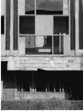
8.8 >La Tourette Monastery - courtyard facade detail.
