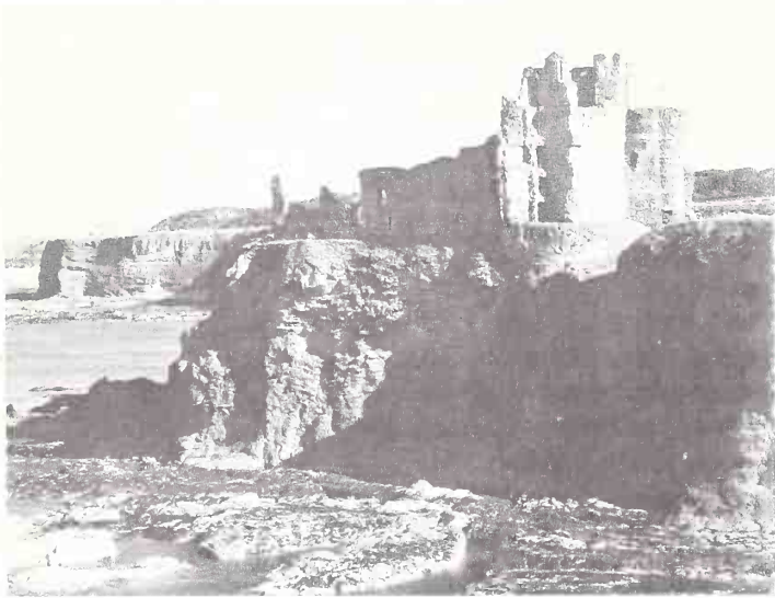
Two methods of blocking the enemy's advance. Tantallon, built in the late fourteenth century on a headland jutting into the Firth of Forth, has a sort of schildmauer, with a tower at each end and a gatehouse in the centre. Château Gaillard, built 1195–8 on a cliff by the river Seine, has a keep (K), inside an inner bailey (IB) and middle bailey (MB). The only practicable approach is blocked by the formidable outer bailey (OB) and its deep ditches.
