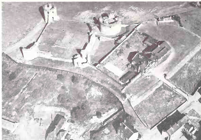
At Flint (plan, page 34) the circular keep acts as corner tower to the inner bailey and dominates the weak outer, but is also an independent stronghold with its own moat. The idea may have been copied from Coucy (page 19) or the Spanish torres albarranas, or even from the old mottes, which normally stood outside their baileys.
