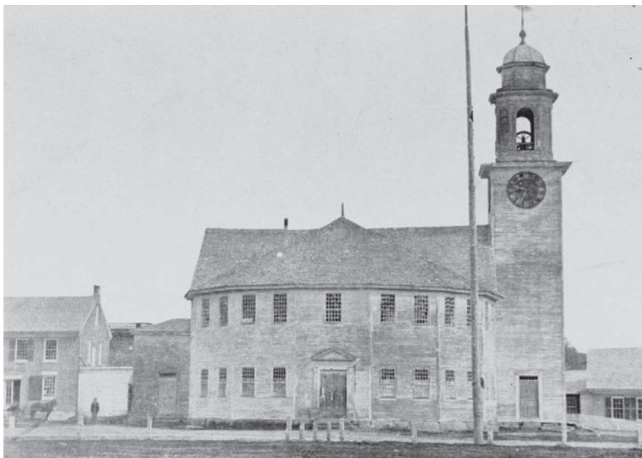
Figure 6.30. Meetinghouse in Claremont, New Hampshire, showing the 1808 semicircular addition to the long side of this 1783 structure. Photograph circa 1857. Collection of the Fiske Free Library, Claremont, New Hampshire.
