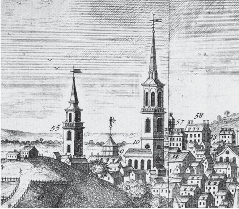
Figure 6.16. The Old South meetinghouse (10) of the Third Church in Boston, as seen in the William Price and William Burgis view. Erected 1729, this house was the third brick meetinghouse in New England and features the same compass-headed windows as the New Brick. The tower on the left (55) is the Irish meetinghouse raised the same year. From A South East View of the Great Towns of Boston in New England in America , 1743. Courtesy of the American Antiquarian Society.
