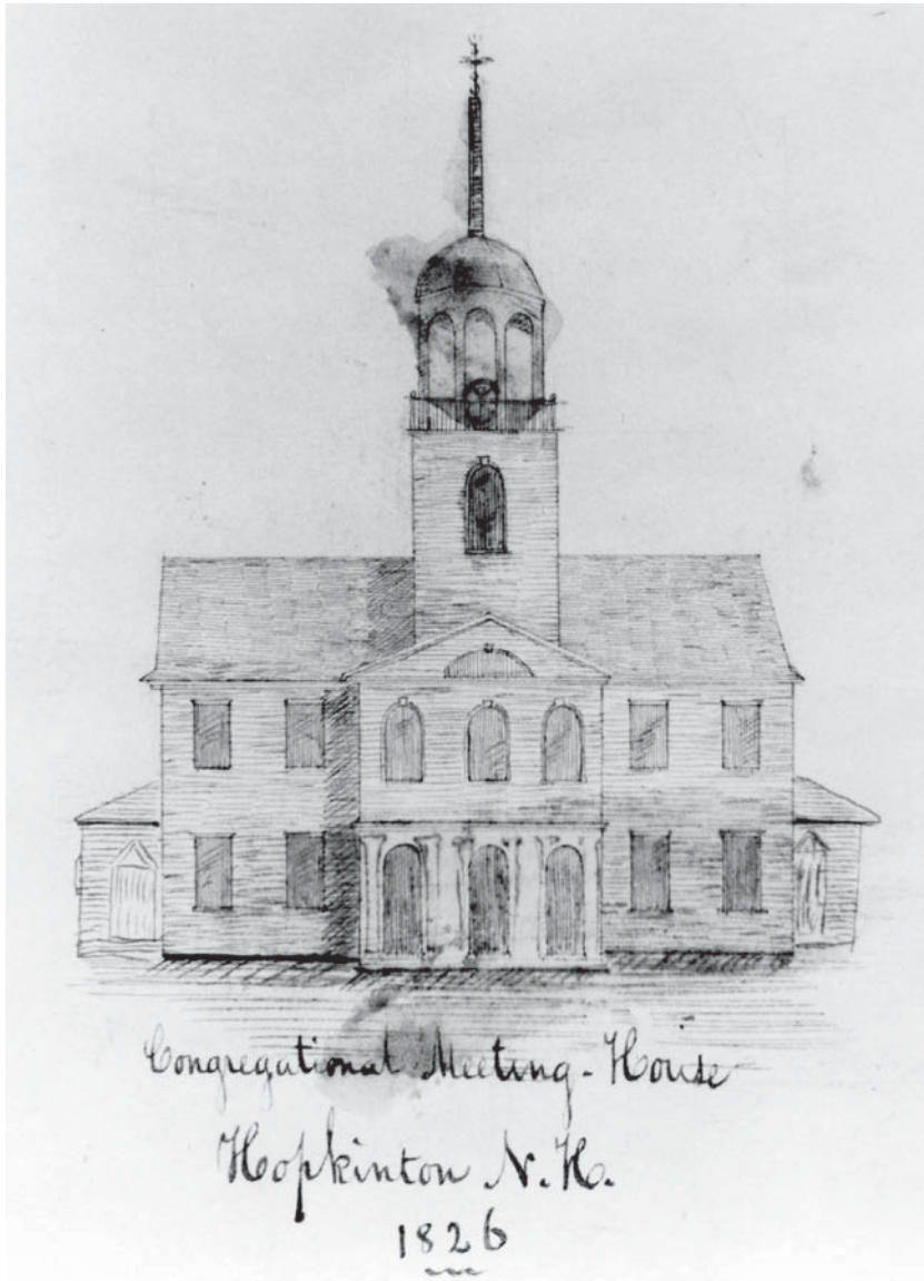
Figure 7.6. Congregational Meeting-House / Hopkinton N.H. / 1826 . View of the 1789 twin-porch meeting-house in Hopkinton after a pavilion and bell tower were built on the long side. The pavilion was added about 1800; the tower erected between 1809 and 1811. New Hampshire Historical Society.
