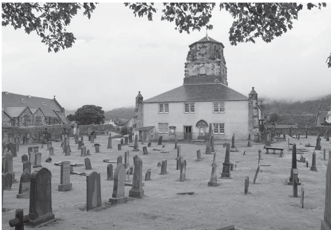
Figure 5.5. Burntisland Parish kirk, Fife, Scotland, erected by mason John Roche in 1592. This meetinghouse was heavily altered in the eighteenth and early nineteenth centuries, with stone buttresses added to each corner and a wooden turret replaced with a stone tower. Photograph by Ian Macdonald, 2007.
