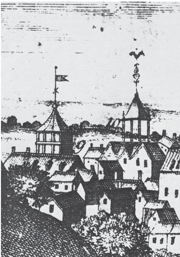
Figure 5.18. “Old Cedar,” seen on the right (10), was the first meetinghouse of the Third Church, Boston, erected 1669. The image reveals three gables and a raised turret with a pyramid at each corner. The lean-to just below it may be one of its three stairwells. From William Burgis and William Price, A South East View of the Great Town of Boston in New England in America , 1725. I. N. Phelps Stokes Collection, Miriam and Ira D. Wallach Division of Art, Prints and Photographs, The New York Public Library, Astor, Lenox and Tilden Foundations.
