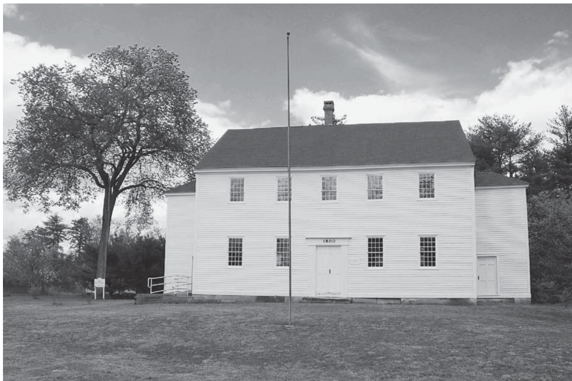
Figure 6.37. Twin-porch meetinghouse in Poplin, New Hampshire, now the town of Fremont. Built by public subscription in 1800, the meetinghouse served as a house of worship and as a town house through 1911. Each porch provides both an entrance to the meetinghouse and stairwell access to the gallery. Photograph by Paul Wainwright, 2008.
