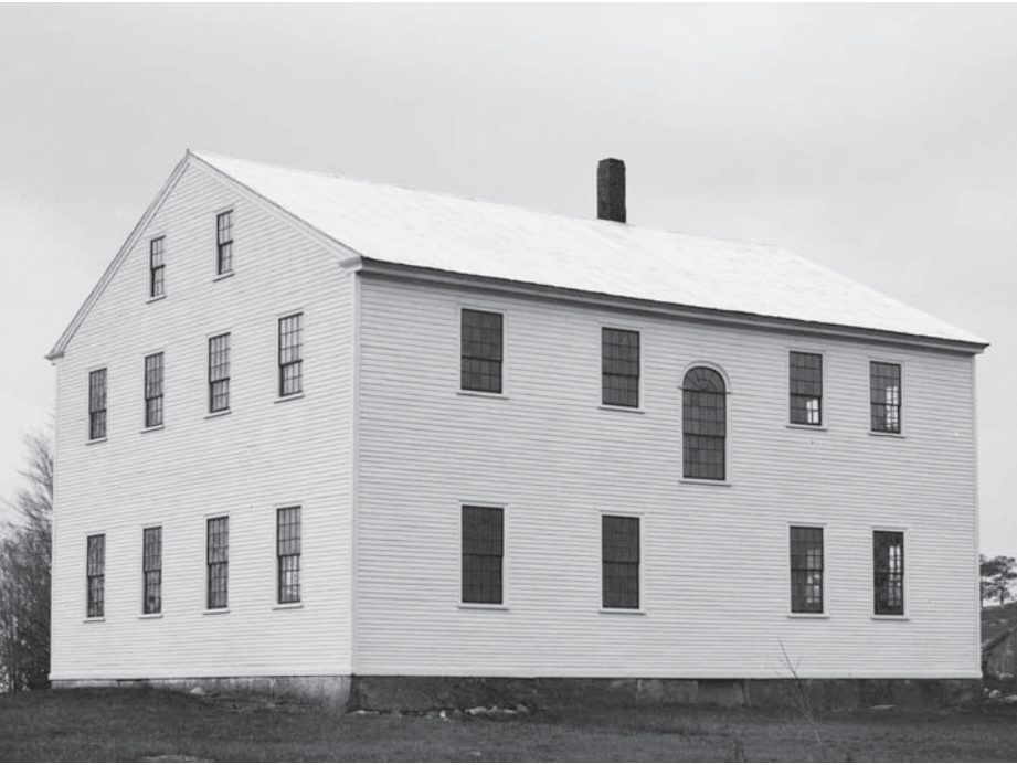
Figure 6.7. North view of the “Old Bullockite” meetinghouse built in Porter, Maine, in 1818, showing the compass-headed window providing light to the pulpit. Named after Elder Jeremiah Bullock, a fundamentalist Baptist preacher, this house was one of the last eighteenth-century meetinghouse types raised in New England. Photograph taken in 1936 by Josiah T. Tubby. Historic American Buildings Survey, Library of Congress, Washington, D.C.
