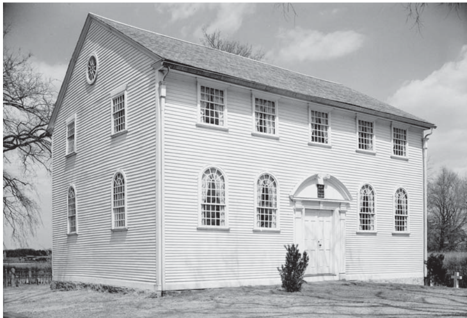
Figures 6.2 and 6.3. Exterior and interior views of St. Paul's Church in Wickford, Rhode Island. This Anglican church took a "meetinghouse form" with the pulpit (on left) opposite the doorway (on right), but the builders nevertheless made sure to use compass-headed windows. Exterior photograph by Stanley P. Mixon, 1940. Interior photograph by Arthur W. LeBoef, 1937. Historic American Buildings Survey, Library of Congress, Washington, D.C.
