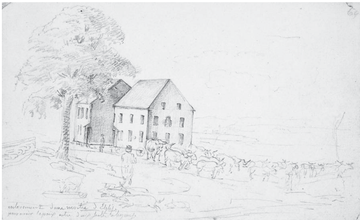
Figure 6.32. Enlèvement d'une moitié d'une église pour avoir la paix entre deux sectes religieuses. [Removal of half of a church in order to have peace between two religious sects.] A sketch taken in New Bedford, Massachusetts, 1816, by Charles-Alexandre Lesueur, showing workmen separating two sides of a meetinghouse, mounting one-half on wheels and hauling it away with oxen. It was the same process used by parishes to enlarge the meetinghouse by pulling one-half from the other and framing in the space. Muséum d'histoire naturelle, Le Harve, France.
