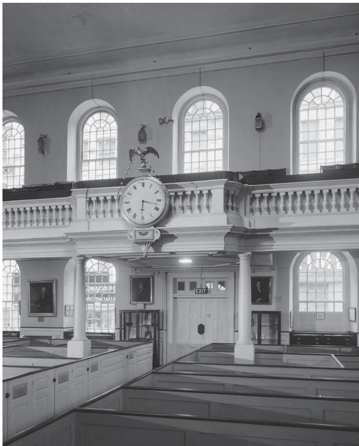
Figure 6.6. Interior view of the 1729 Old South meetinghouse, Boston, Massachusetts, showing the use of compass-headed windows extending throughout the building, including the pulpit window. Historic American Buildings Survey, undated photograph taken circa 1950 to 1960. Library of Congress, Washington, D.C.
