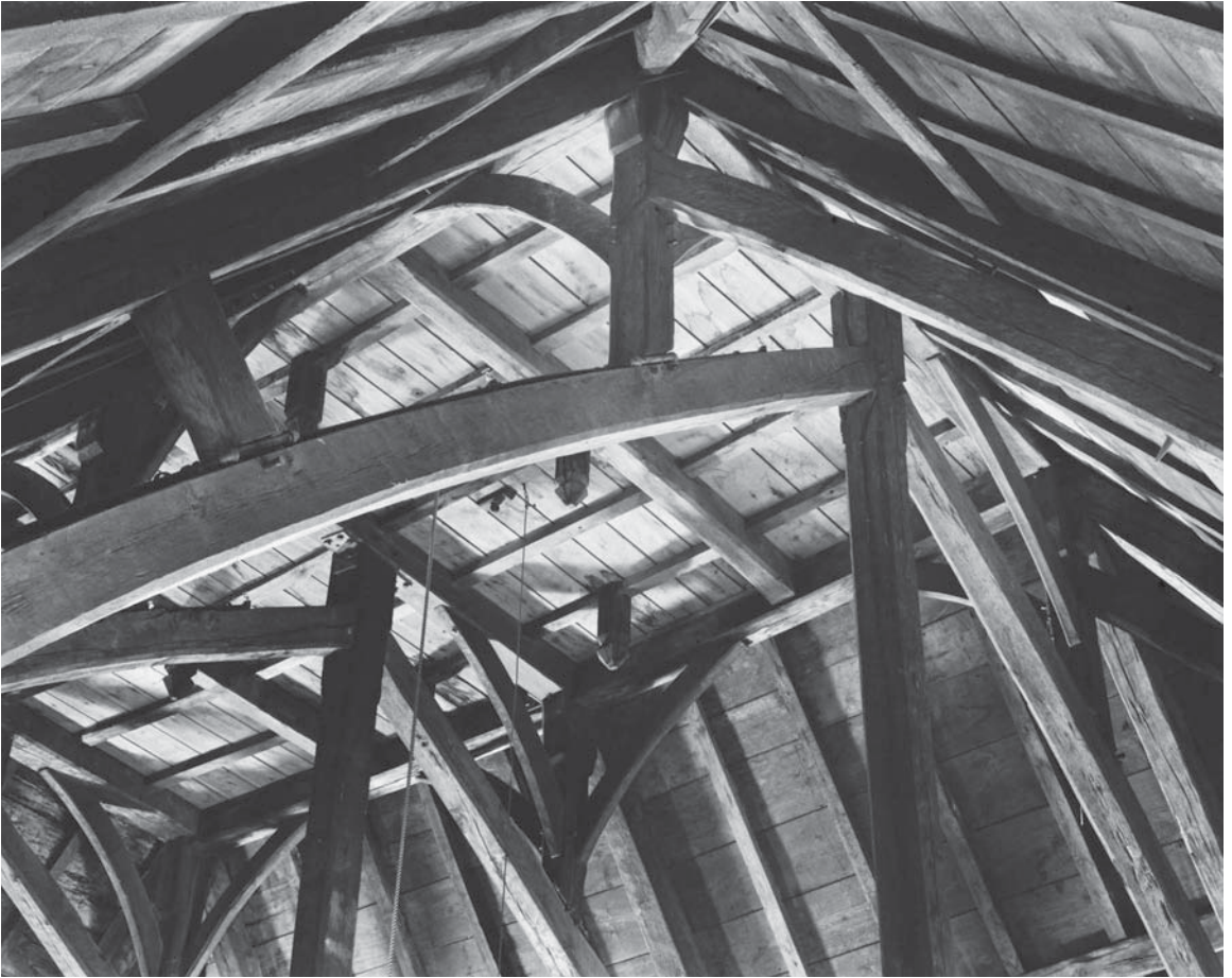
Figure 1.5. Trusses supporting the roof and belfry of the second meetinghouse built in Hingham, Massachusetts, in 1681. The appearance of these timbers led to its name, the “Old Ship.” Photograph by Paul Wainwright, 2008.
