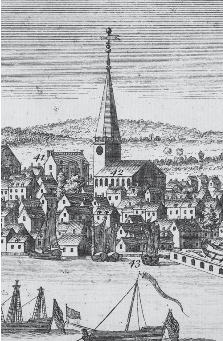
Figure 6.11. Detail from William Burgis and William Price's view of the 1714 New North meeting-house in Boston, showing an octagonal steeple rising from the top of the bell tower battlements. This may have been the first "dissenting steeple" in New England. A South East View of the Great Town of Boston in New England in America , 1743. Courtesy of the American Antiquarian Society.
