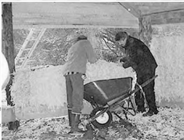
3.2b: Shredded paper bales being installed within a frame.
