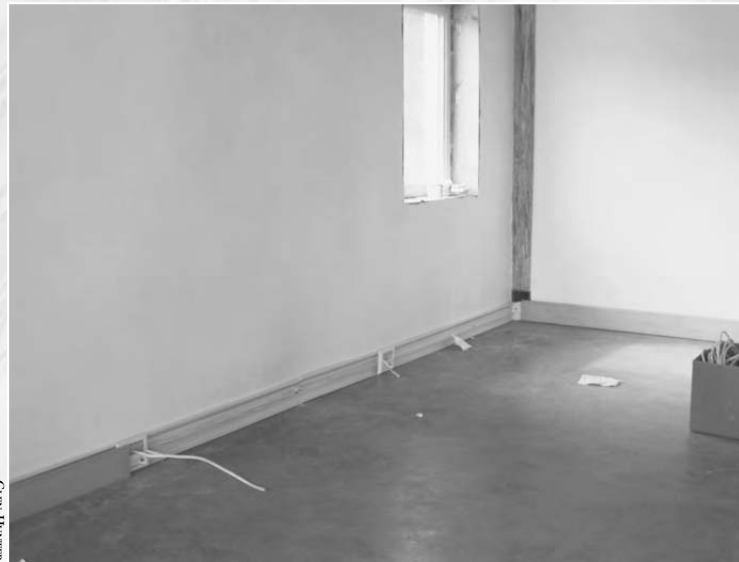
10.8: Baseboard wiring keeps all lines out of the walls. They allow access to wiring; the trade-off is cost.
