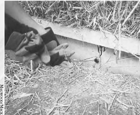
18-20: Wire is passed through the foundation and over the top plate.
