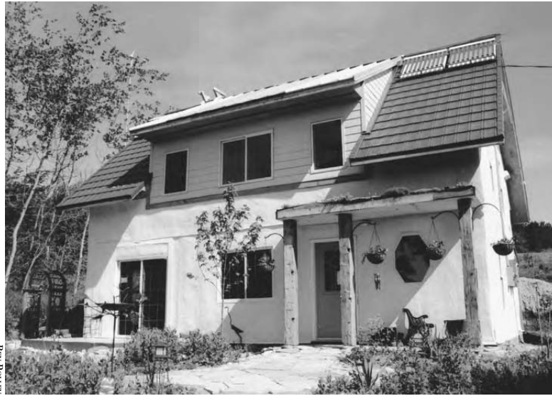
20.5: Silicate paints, used on the exterior of this home, are ideally suited to plastered bale walls, as they are designed to bond with mineral surfaces to eliminate water penetration but still allow the walls to “breathe.”
