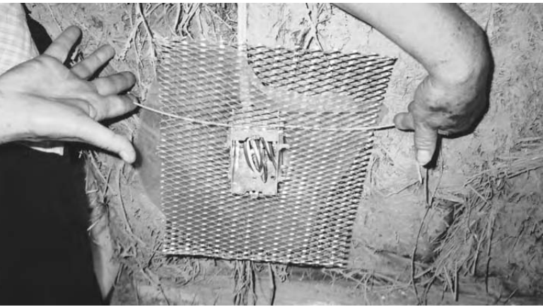
18.14: A metal electrical box has been vapor barriered, meshed, and is being attached to the wall using galvanized wire run through the mesh and the screw holes in the box. Wire pins hold everything snug against the straw.
