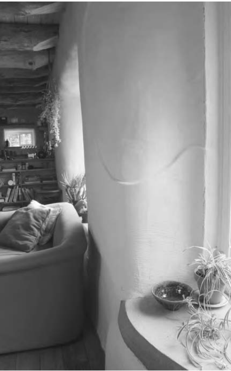
20.2: The top coat and relief work around this window seat are a gypsum and sand mix with a gypsum wash coat.
