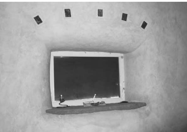
20.3: These tiles are set into a white clay top coat, and a hempcrete mixture forms the window sill.
