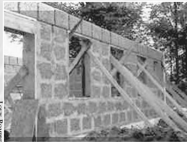
3.2d: Stranbloc is made from any waste fibre.
