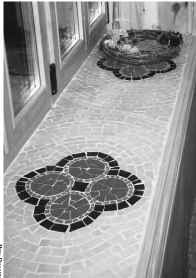
20.6: Window sills can be plastered, covered with a nice piece of wood, or artistically finished with a mosaic as pictured here.
