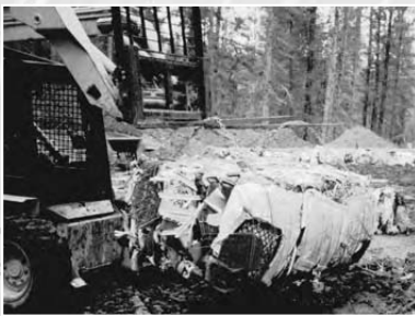
3.2c: Plastic bales being used as a foundation.
