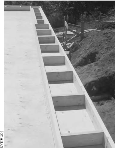
12.11: The top plate for a load-bearing building is usually a simple affair: two side rails, some blocking, and a plywood base. It will be built on the foundation prior to the bales being raised. The cavities will be filled with insulation and the box topped with plywood once it is in place.
