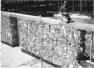
3.2a: Boxboard bales used as a load-bearing wall.
