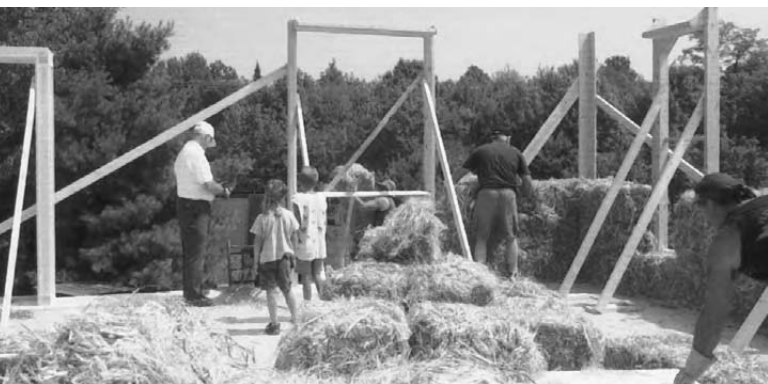
18.4: Door and window bucks must be braced plumb and square. They will likely see lots of abuse!
