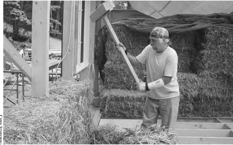
18.12: A quick tap with the beater settles new bales into the wall.
