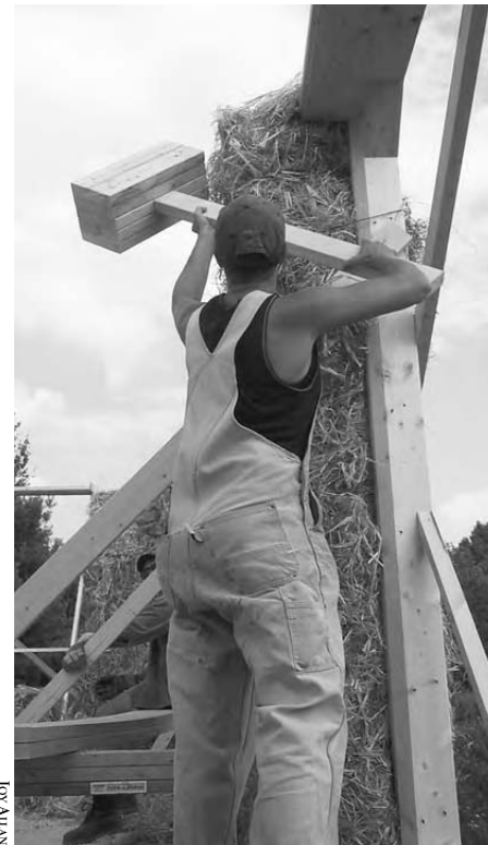
18.32: Gently persuading the bales into line.
