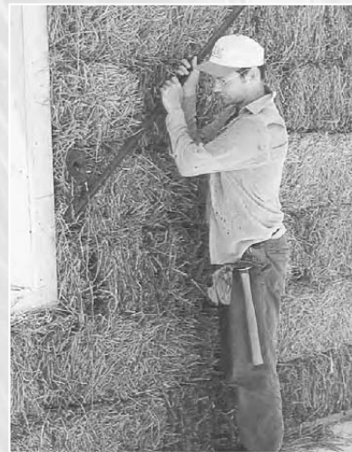
18-25: A downward force is applied to the bar or come-along drawing the top plate down.
