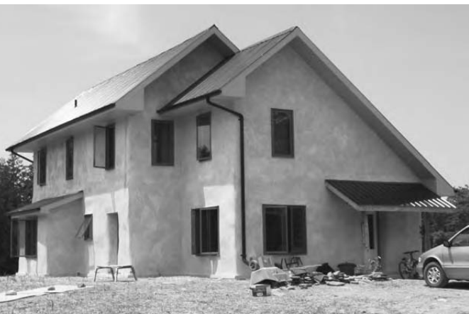
15.1: The Soltan residence.
