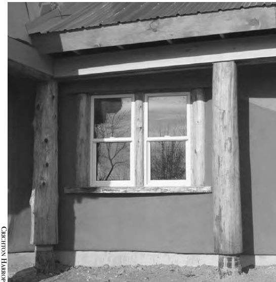
20.7: Deep, rich colours can be achieved using clay-based tints in a clay paint. Coated with a clear silicate finish, this is a long-lasting colour.
