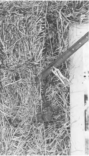
18-22: A come-along is clipped to a fence-stretcher in readiness for pre-compression.
