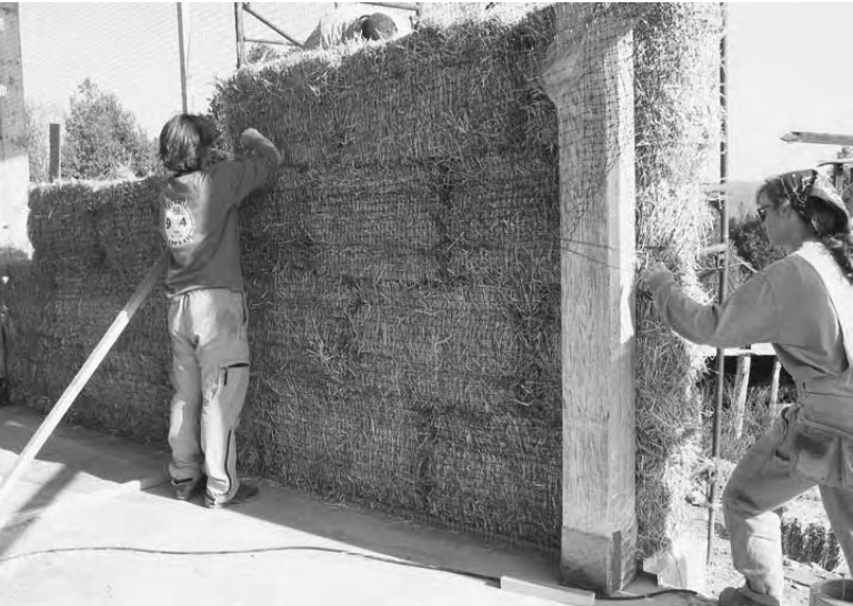
18.18: Sometimes bales simply refuse to rest snugly against a post. Tie them to the post temporarily; once the first coat of plaster is on they won't move and you can cut the strings.
