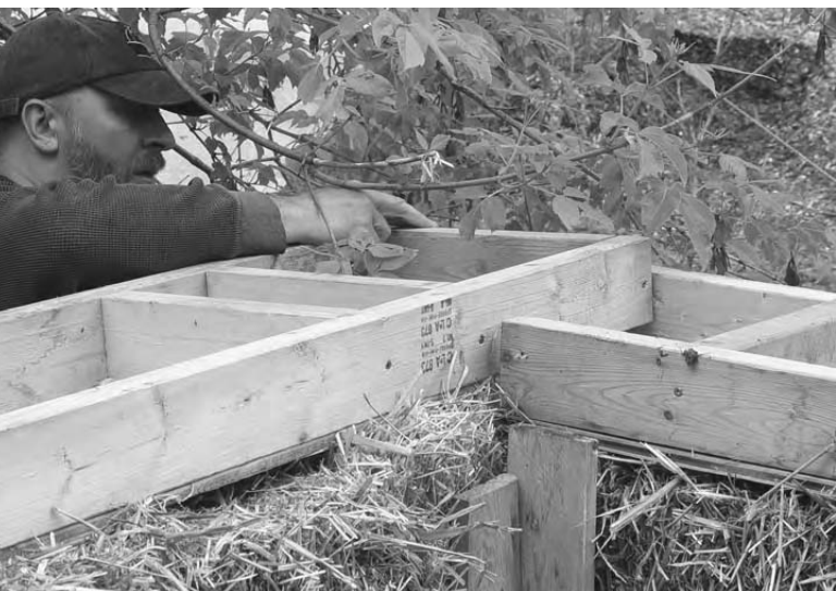
18.30: Top plates need to fit together snugly and up against the corner guide which is checked for plumb.
