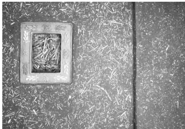
20.4: A high quantity of chopped straw in a clay finish coat can add texture and color to the finish.
