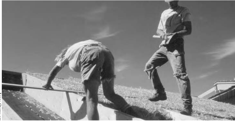
8.8: Bales go into a roof with framing that is spaced perfectly to fit.
