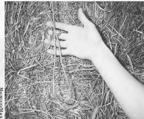
18-21: A loop is created in the upper end of the wire with a saddle clamp.
