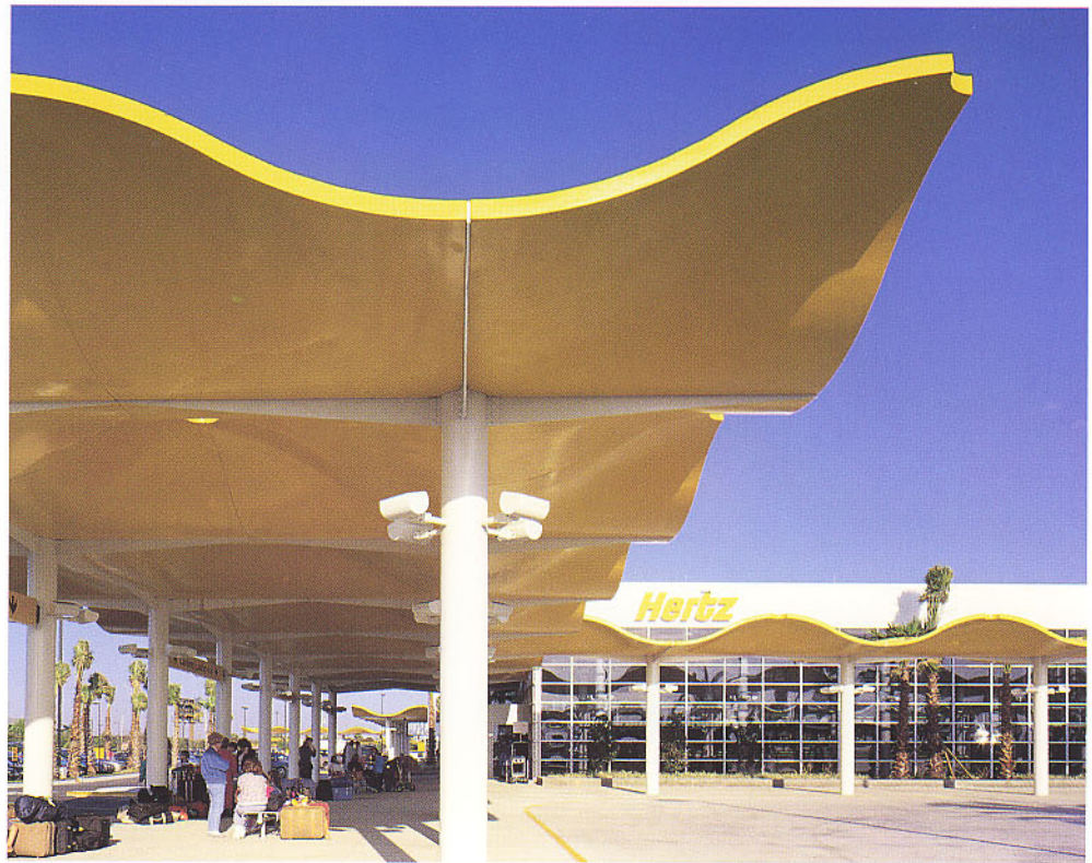
The reception bay is protected by undulating modules of fibreglass supported by a structure of metal pillars.
