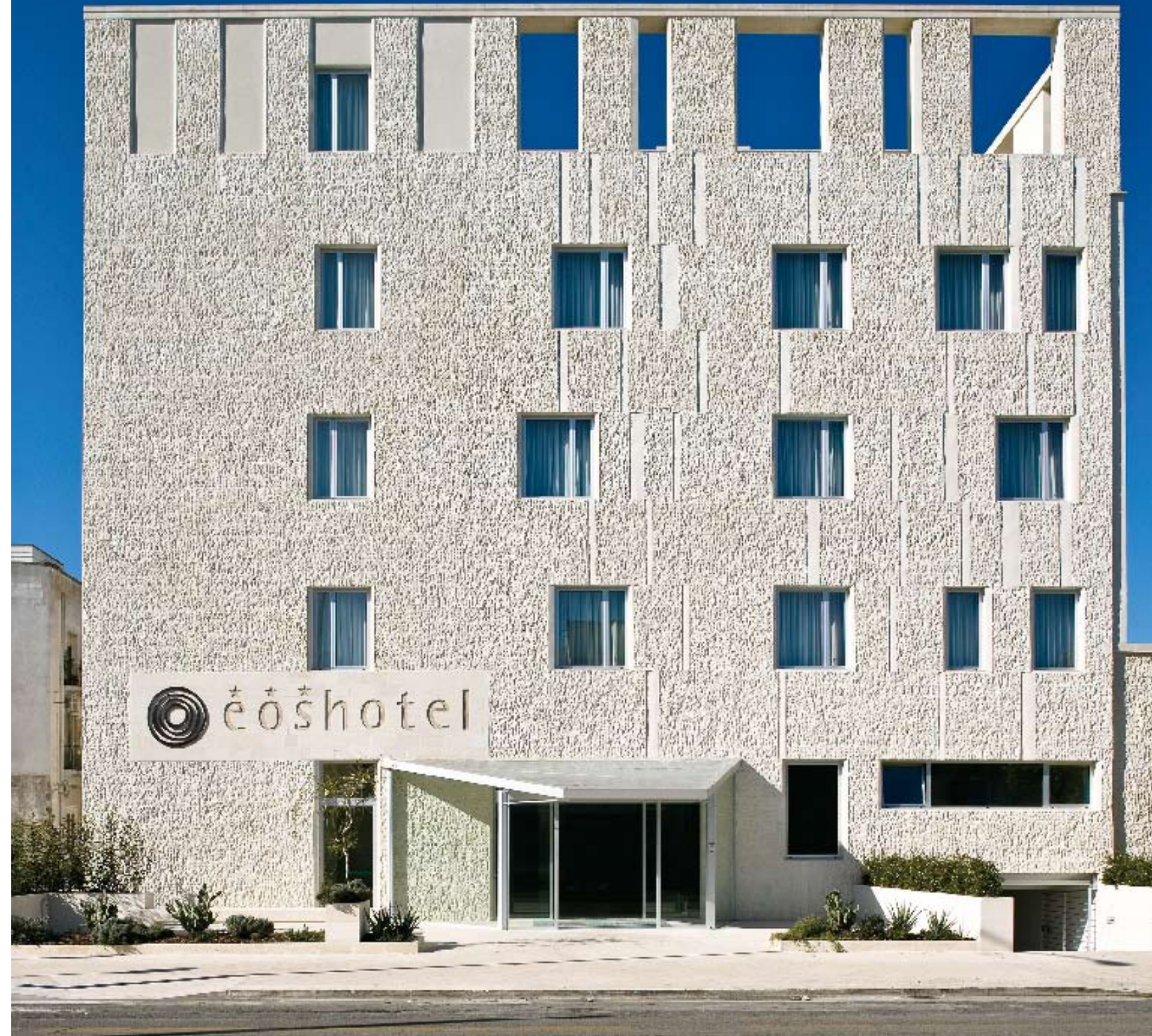
1-2. Eos Hotel building site 3. Façade in "leccese" stone of Eos Hotel
