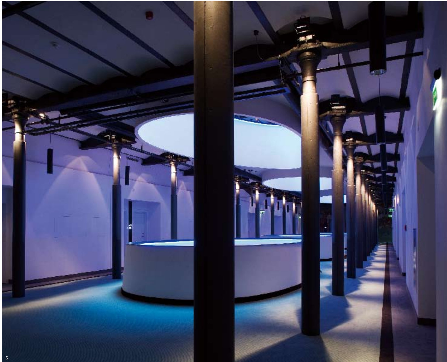
9. Bedrooms are located to the perimeter of the upper levels to take advantage of the natural light from the high factory windows 10. Three stacks of elliptical light wells punched through the full height of the building
