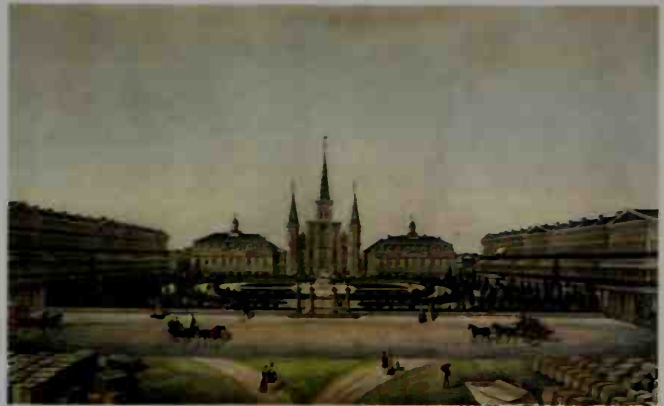
The Pontalba Rows face each other across Jackson Square, newly landscaped as a French garden in this late-1850s view. The houses completed the architectural ensemble on the square (begun with St. Louis Cathedral)—and revitalized the Vieux Carré.
