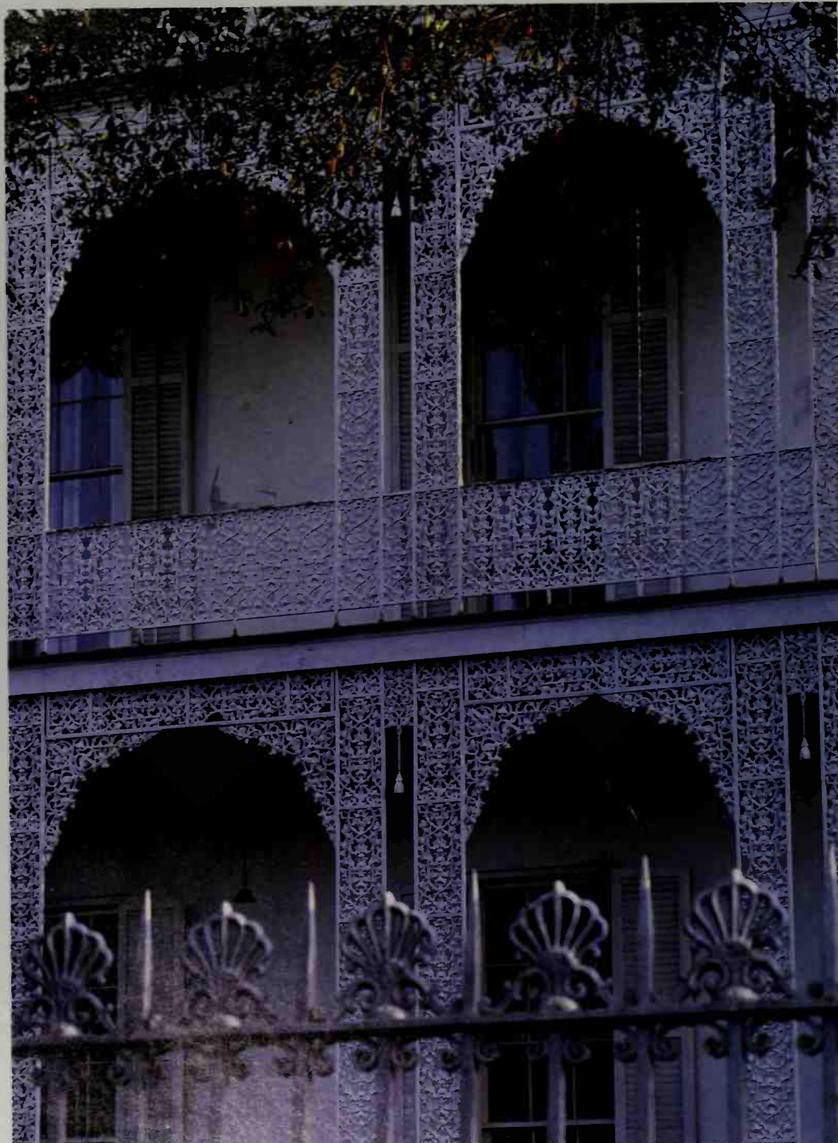
A scrim of white cast iron turns a grand house into a summer pavilion—it is refreshing even to look at the lacy, arched framework of iron. Palmetto fans and spears alternate in the fence surrounding the property.
