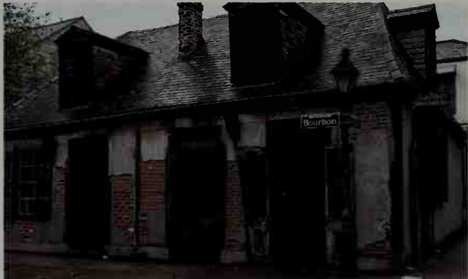
This early cottage on Bourbon Street is known as Laffite's Blacksmith Shop—the French pirate Jean Laffite allegedly used it as a cover for smuggling operations. The stucco has eroded, exposing the standard brick-between-posts construction.
