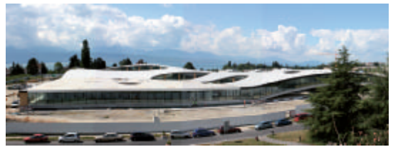
The mild curvatures of the shell roof at the Rolex Learning Center by SAANA necessitate several intermediate supports for the largest shell, thus creating a hybrid structure that would have been difficult at best to be designed without computational analysis (photo: Matan Mayer)
