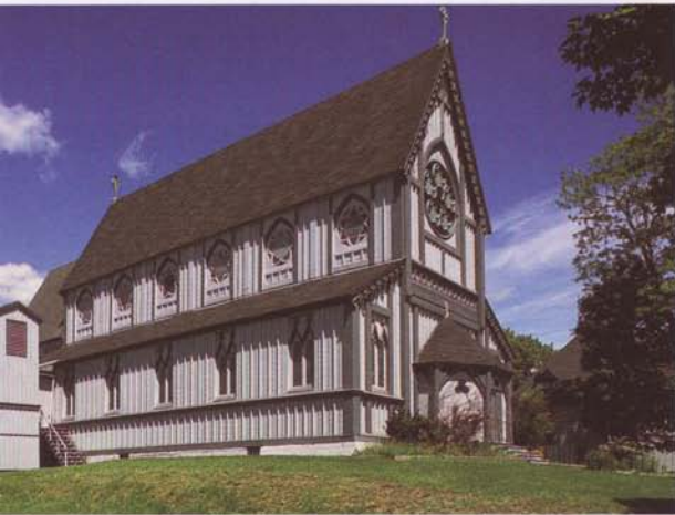
3-26 – Christ Church, St. Stephen, New Brunswick, exterior from north-west.
