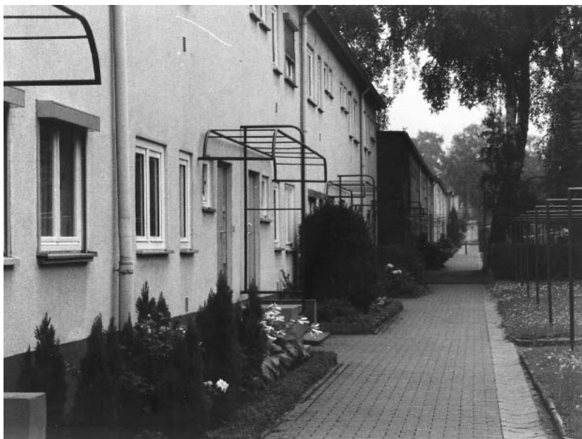
Westhausen, pedestrian path giving access to dwellings and gardens.
