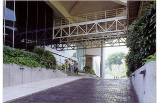
BELOW: Entrance drop off; main lobby; office floor partitioning; OPPOSITE, L TO R: East elevation; architect's studies for 'vertical landscaping' into the facades and the 'sky court'
