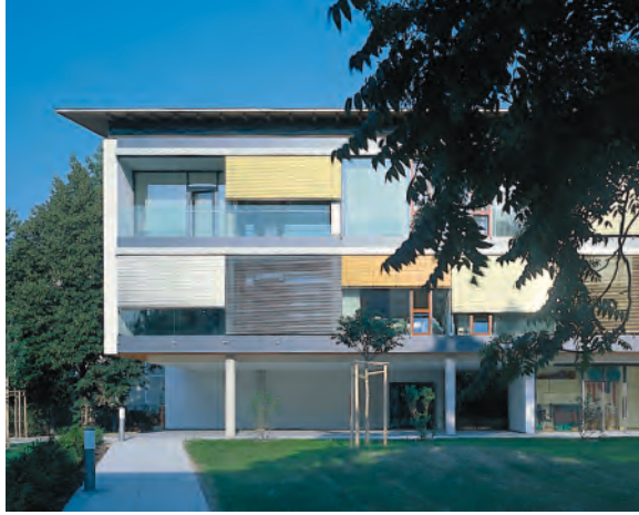
Facade, St. Georg Hospital, Leipzig Architecture: HPP Laage & Partner, Stuttgart/Leipzig
