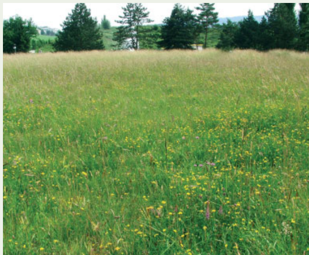
Part of the sward on the 3-hectare (7.4-acre) living roofs of the Moos lakewater filtration plant in Willishofen, Zurich. This sward is now the only remaining example of this grassland type in this canton of Switzerland and has been proposed as a national park. There are more than 175 plant species on the roof, among them seven orchid species, including around 6,000 green-winged orchids.
