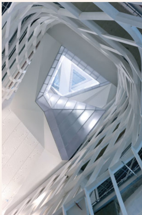
A spiralling atrium sweeps through the new building filling the entire interior with light and physically connecting the activities on all nine levels with a central staircase and 'skybridges'. But in the spirit of the mystery suggested by the facade, the atrium is just out of view of the entrance. Its south wall is covered with perforated glass-fibre-reinforced gypsum acoustical panelling on the inside and glass-fibre-reinforced concrete panelling on the outside of the building.
