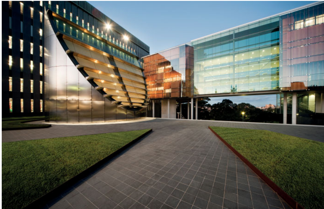
View across the Eastern Avenue forecourt.
