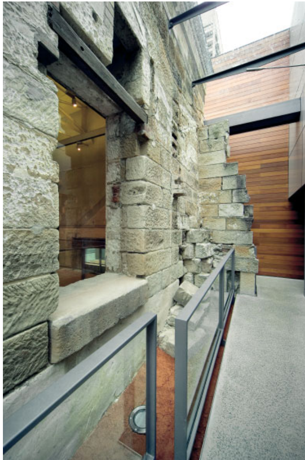
Insertion of new elements within the building's traditional fabric.
