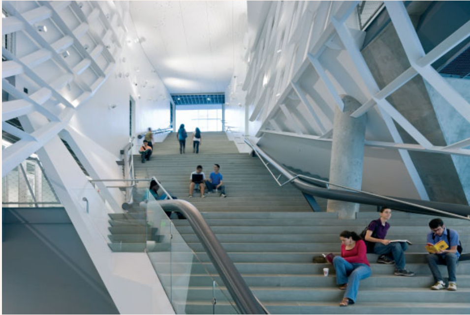
The angular central staircase, which sweeps from the ground level through the third floor, is enveloped in and defined by a porous 'mega mesh' lattice wall, ingeniously composed of a combination of straight and curved steel tubes. Contractors devised a clever system to build it, sliding steel balls precisely on to the horizontal pipes, welding them in place, and connecting the diagonals with the steel balls, then covering them all with glass-fibre-reinforced gypsum to create the diamond profile of the moulded form.
