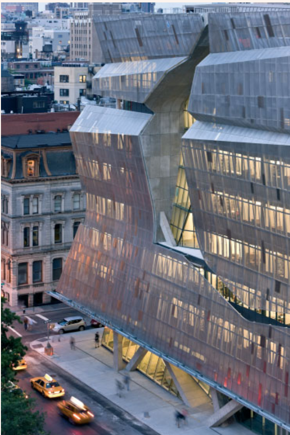
At dusk, 41 Cooper Square looks brighter and more welcoming than it does during the day. The convoluted, perforated stainless-steel skin, which projects as much as 2.4 metres (8 feet) in some areas and less than half a metre in others (especially on the north, south and east sides), reveals the activity inside and the regular column grid behind the window wall that takes over from the V-shaped columns at the bottom of the second floor, which rest on transfer beams below. Floor framing consists of a cast-in-place reinforced-concrete one-way slab system supported by beams and flat two-way reinforced concrete slabs.
