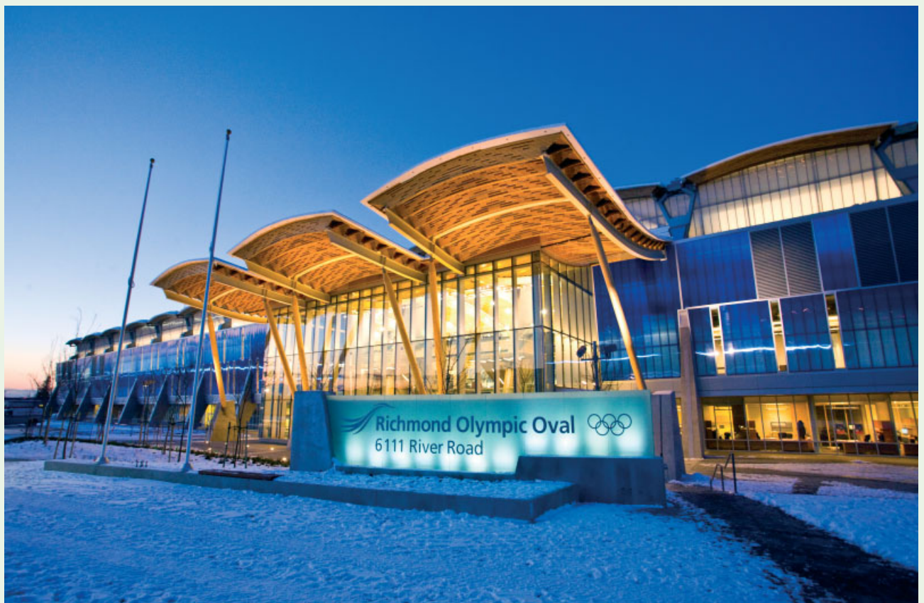
Canon Design, Richmond Olympic Oval, Richmond, British Columbia, 2008 The roof of this 33,000-square-metre (355,220-square-foot) building, the 2010 speed-skating area, is constructed largely of timber; each of the glulam beams is assembled from four elements.
