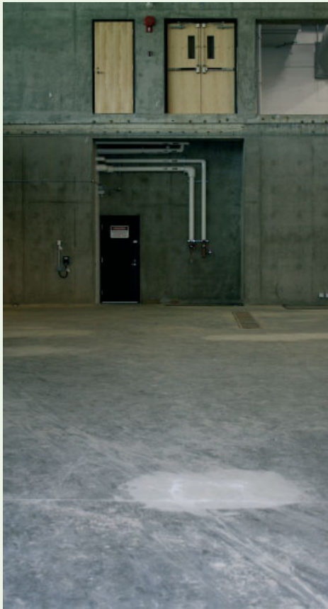
Hughes Condon Marler Architects, Olympic curling venue, Hillcrest Park, Vancouver, 2009–10 Interior of the curling centre, only 'half built' before being completed for its legacy mode. Doors appear high up in walls; the patch in the foreground indicates the position of a future column.
