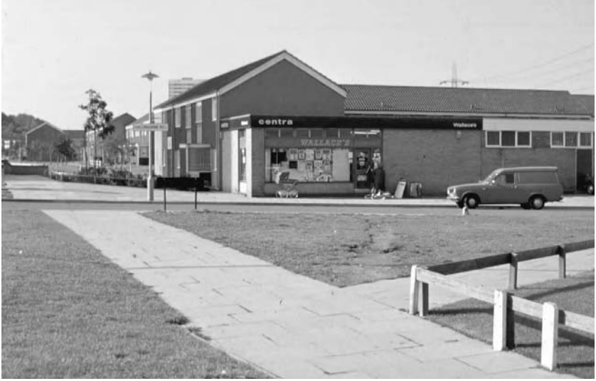
8.8 The idea that people will walk where the hard landscape goes is so silly that one wonders how designers can become so detached from reality!
