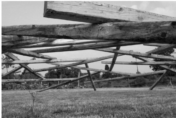
Fig. 5. Second dome completed
