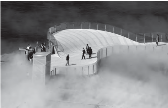
3.3 Diller Scofidio + Renfro, Blur Building, Yverdon-les-Bains, Switzerland, 2002. Copyright, Diller Scofidio + Renfro; courtesy of Diller Scofidio + Renfro.
