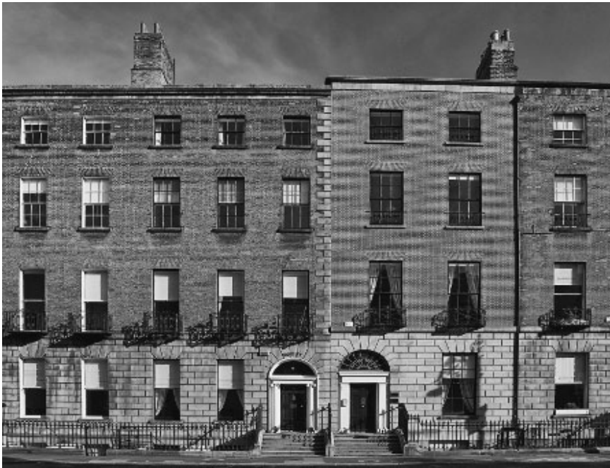
FIGURE 9.1 Buildings on Henrietta Street
