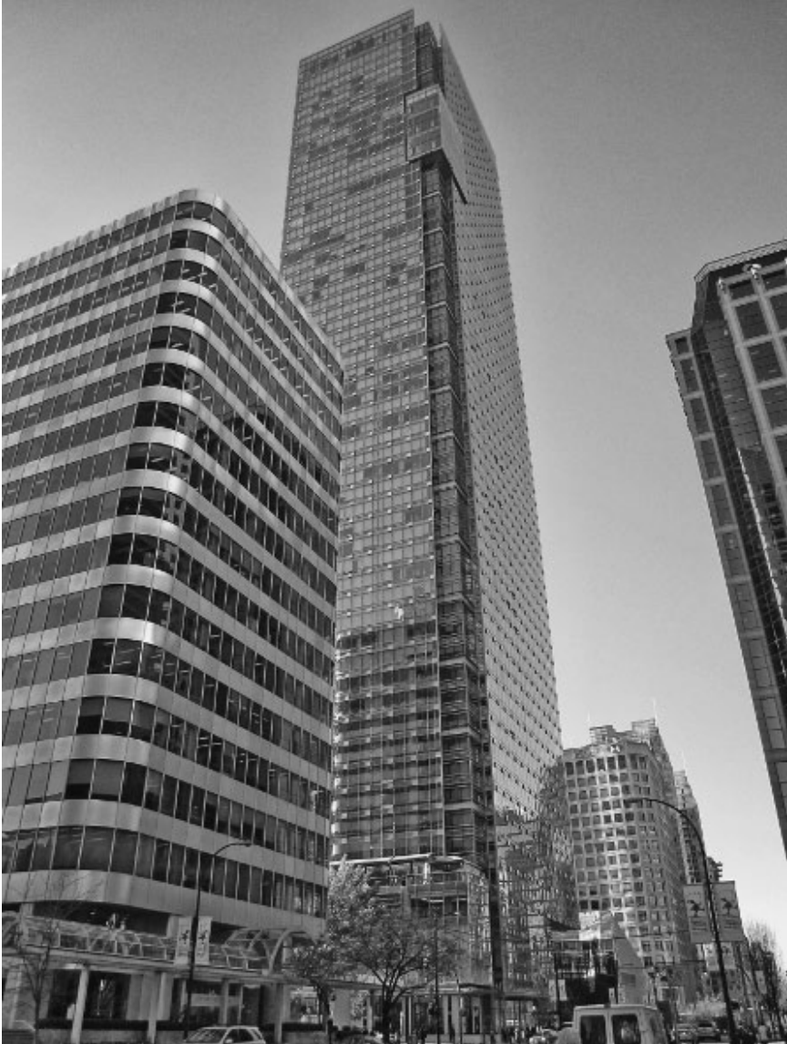
FIGURE 11.7 Shangri-La tower, West Georgia Street, looking north-west
