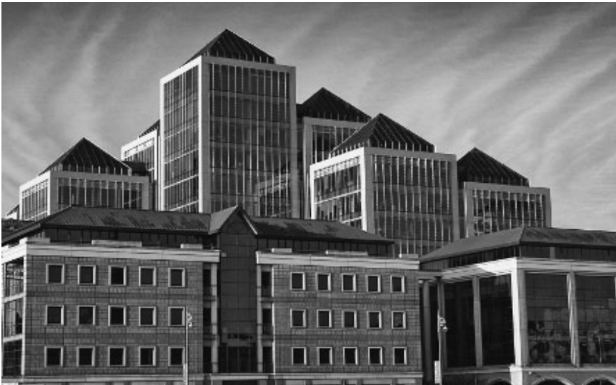
FIGURE 9.2 Looking east towards Docklands from the Four Courts
