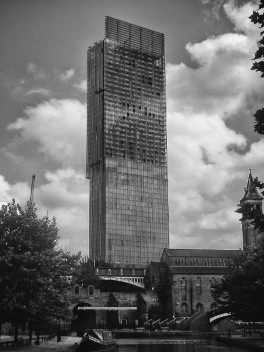
FIGURE 6.1 The Beetham Tower, Manchester
