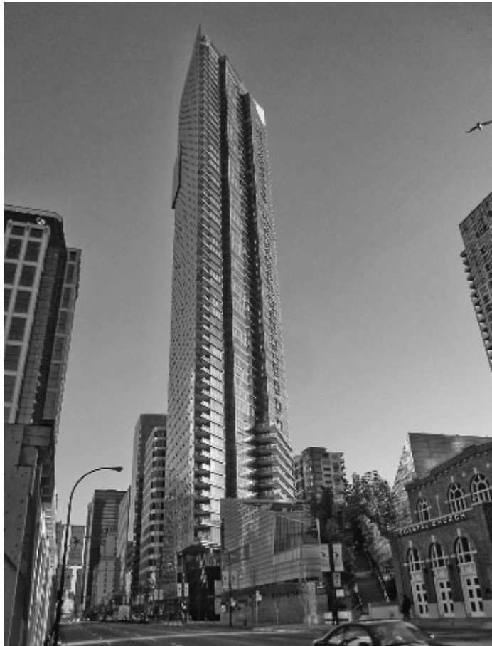
FIGURE 11.6 Shangri-La tower, West Georgia Street, looking south- east
