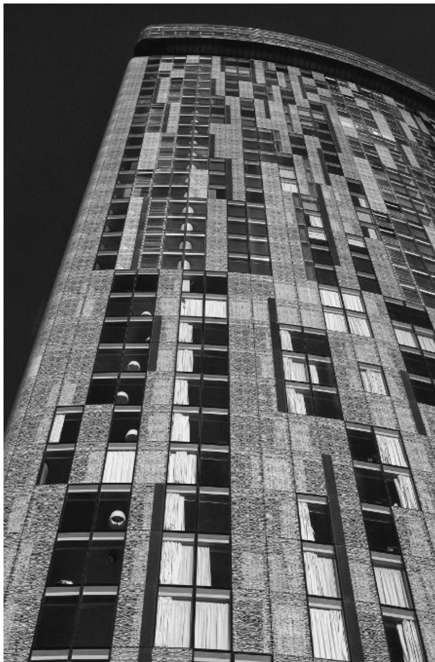
FIGURE 7.5 (above) Completed Beetham Tower
