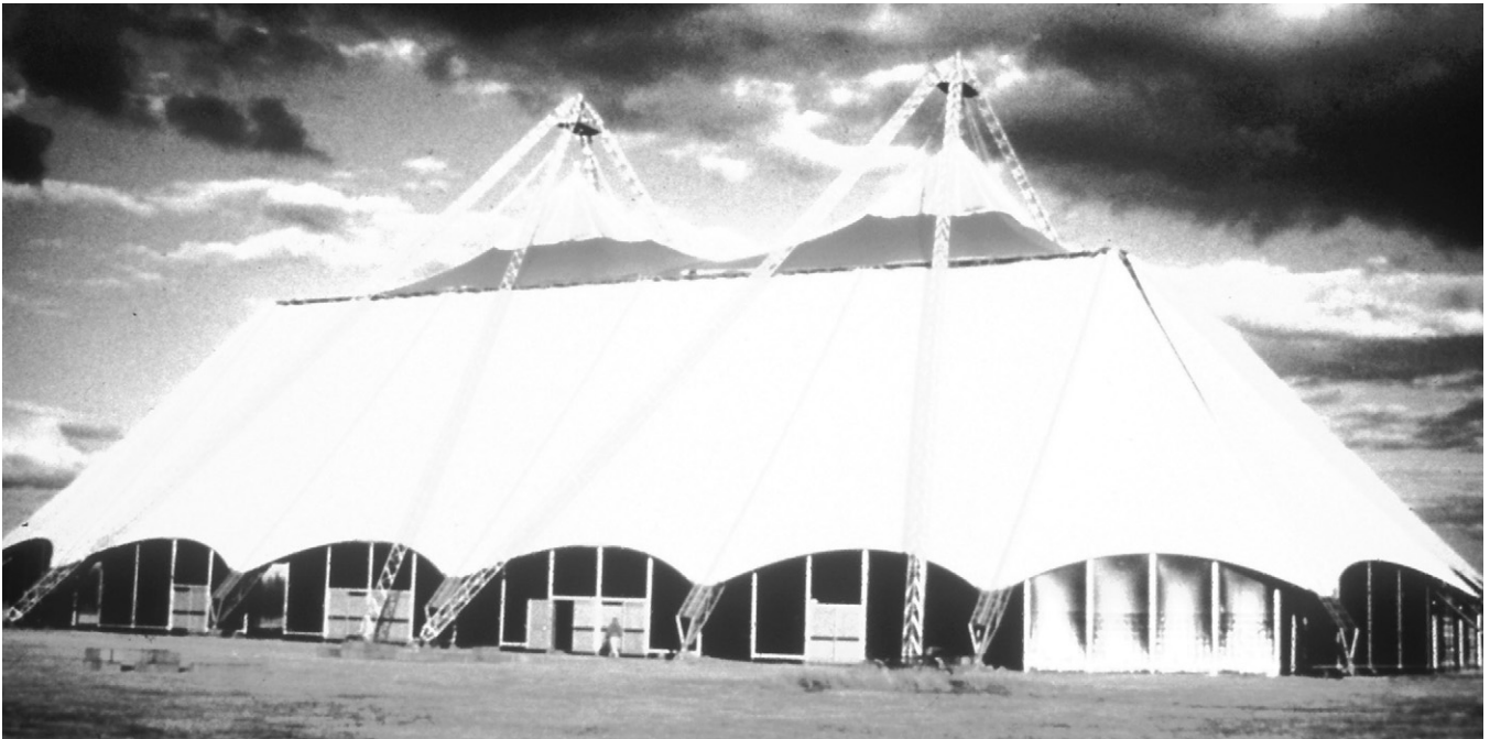
Fig. 9.6 The completed building.
