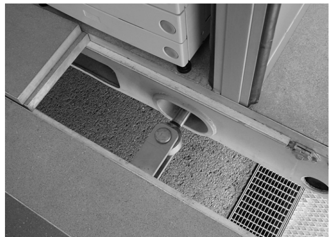
Fig. 5.14 Hydraulic rams concealed in the floor locate the pods accurately.
