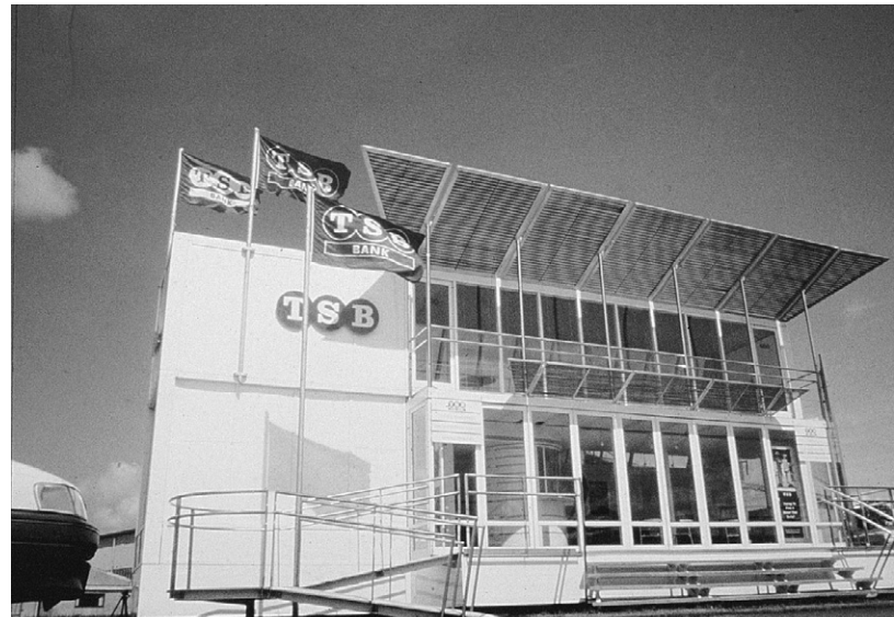
Fig. 6.9 The trailer base is hidden in order to reinforce the image of a building.
