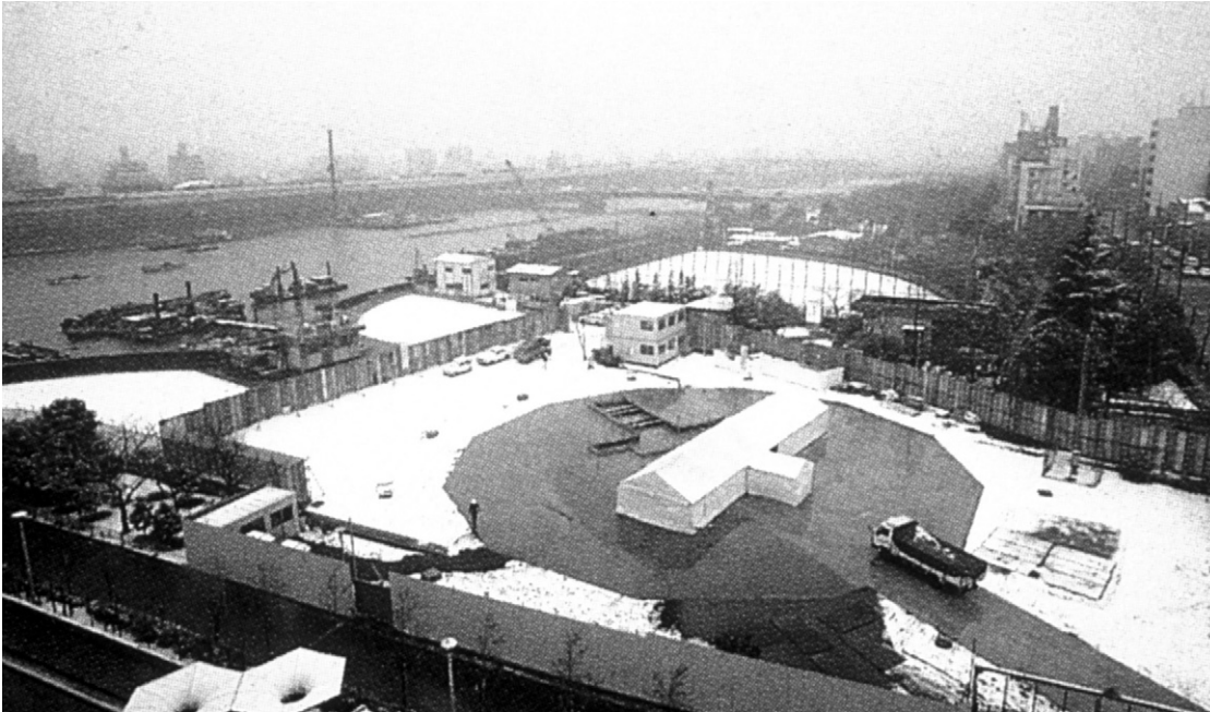
Fig. 2.5 Erection process. The site set out with delivery of scaffolding underway.
