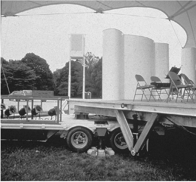
Fig. 12.6 The stage is supported on trailers which are stabilised by foot pads. The vertical white pillars provide a backdrop to the stage and help project sound out to the audience. One of the vertical speaker units.
