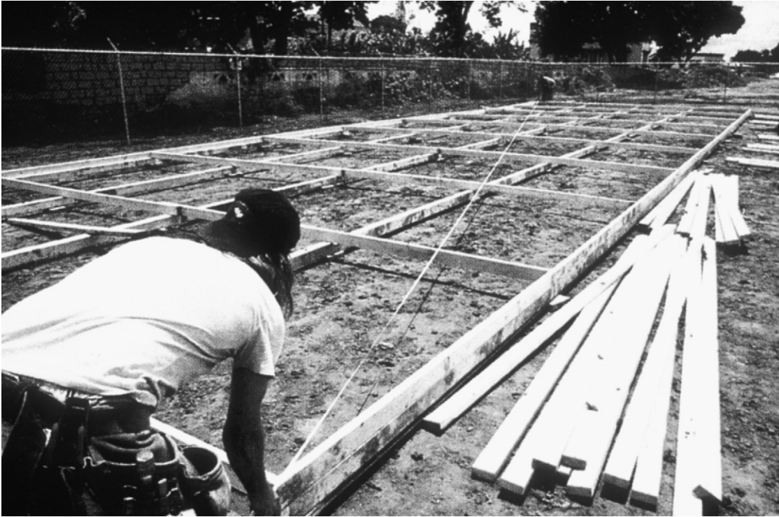
Fig. 16.3 'Series 8' floor being made in a warm climate situation.
