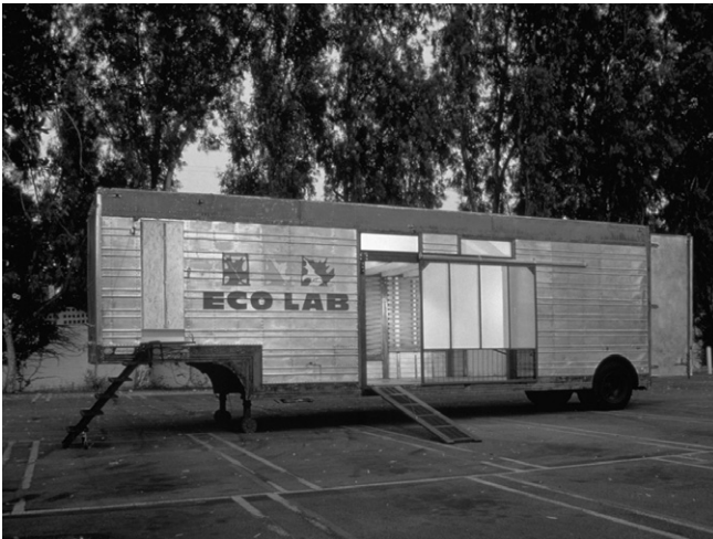
Figure I.34 OMD's Eco-Lab, a mobile building made from recycled components and materials.
