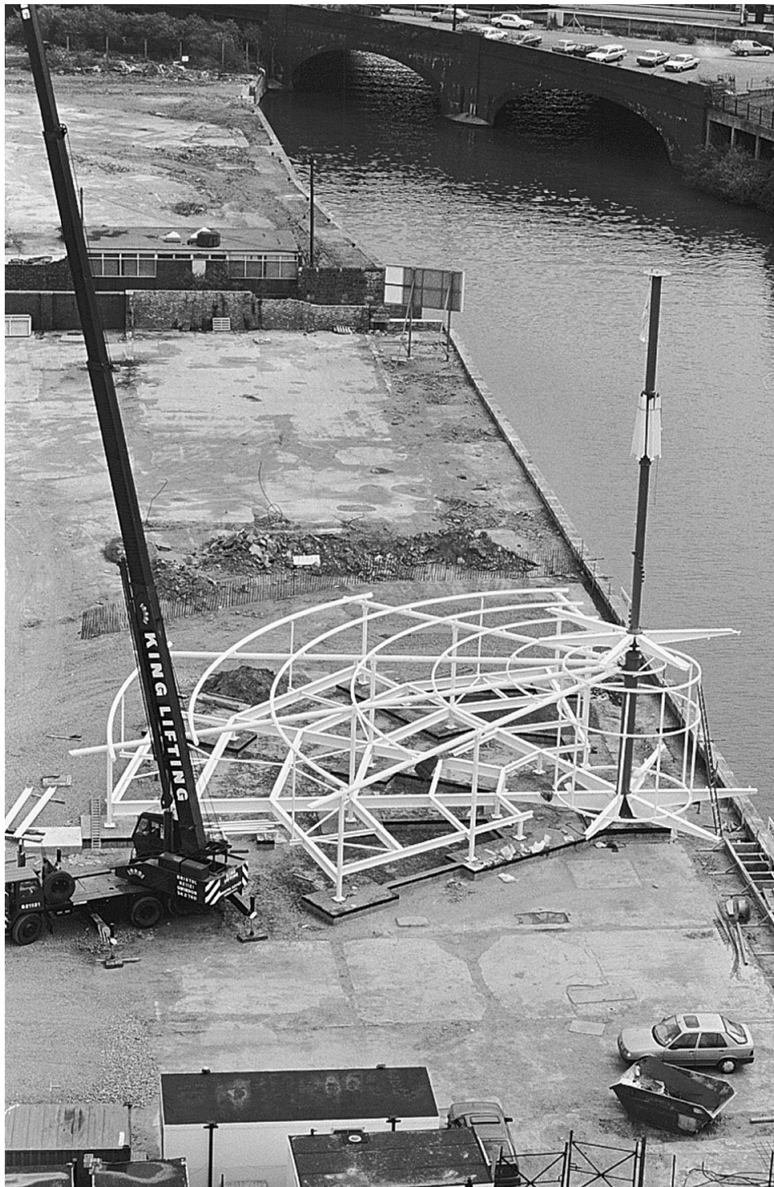
Fig. 7.8 The structure partially erected.
