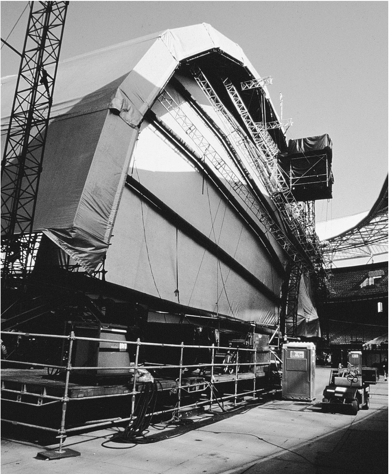
Fig. 13.9 Rear of the set. The rear wall has a twinned structure of radial steel lattice beams and air beams that brace the membrane projection screen.
