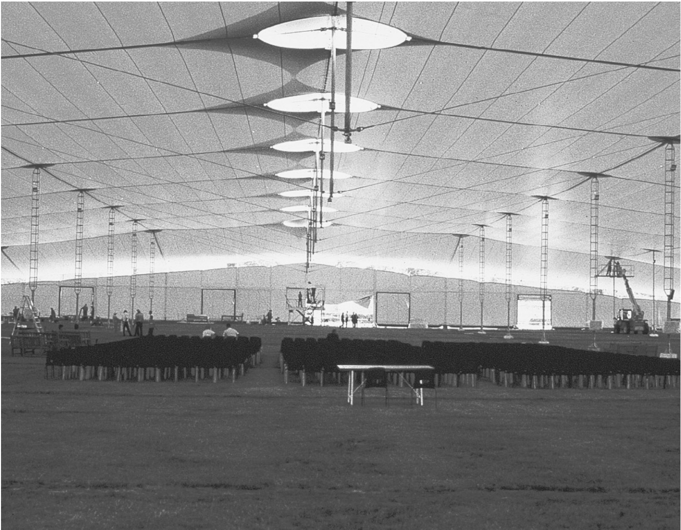
Fig. 9.13 The internal space. A Tensegrity system supports the central bay with openings for ventilation and light protected by separate conical membranes. The columns on either side are triangulated members, the rest are tubes.
