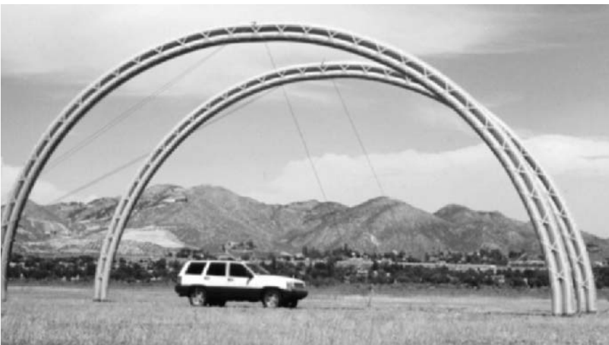
Fig. 12.25 The new generation of slender air-beam tubes.
