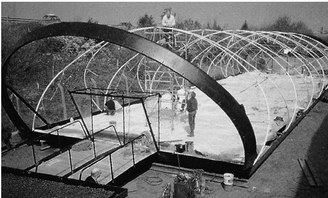
Fig. 3.7 The bare structure before cladding with the PTFE membrane.
