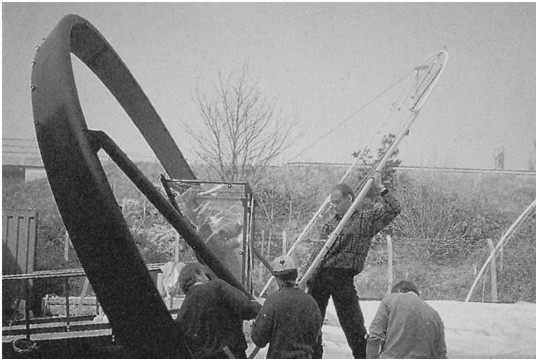
Fig. 3.6 Erection of the end arch section.
