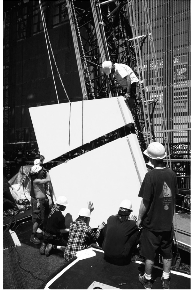
Fig. 13.16 Arch panel assembly.
