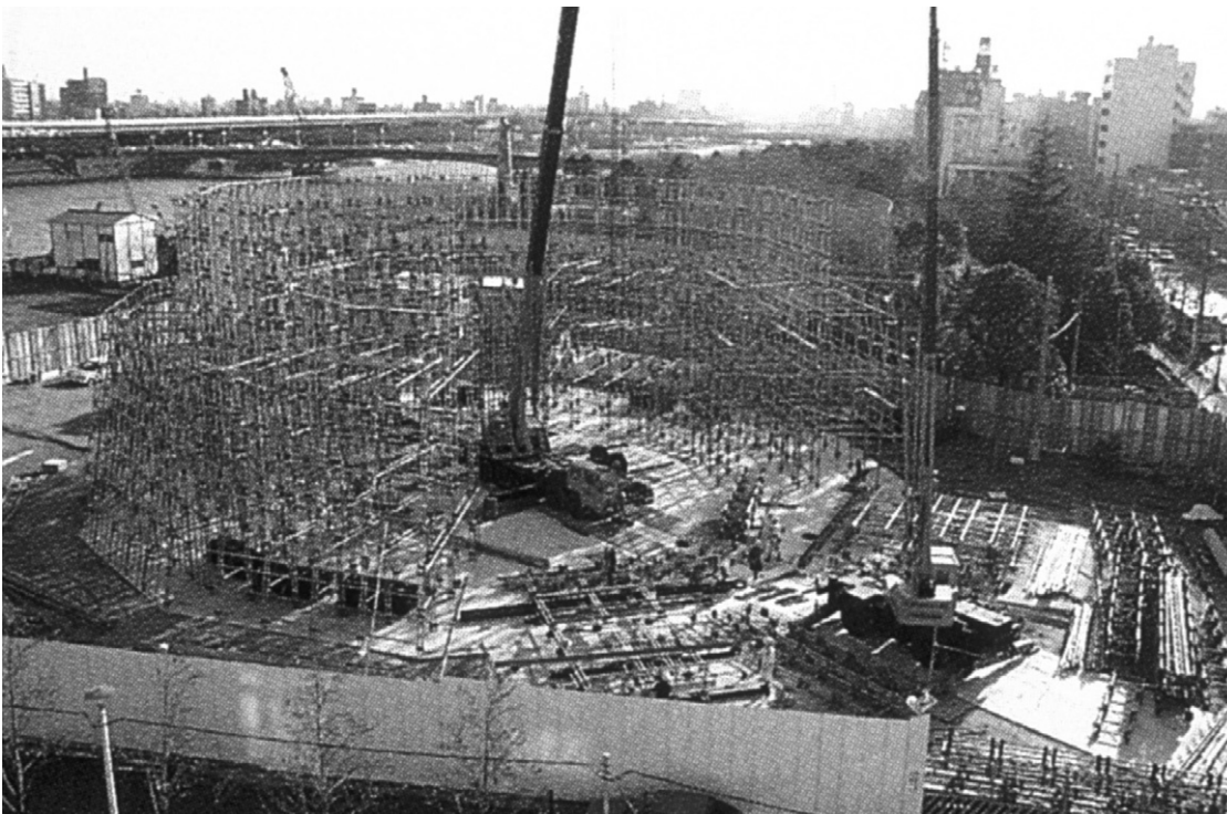
Fig. 2.6 Wall structure under construction.
