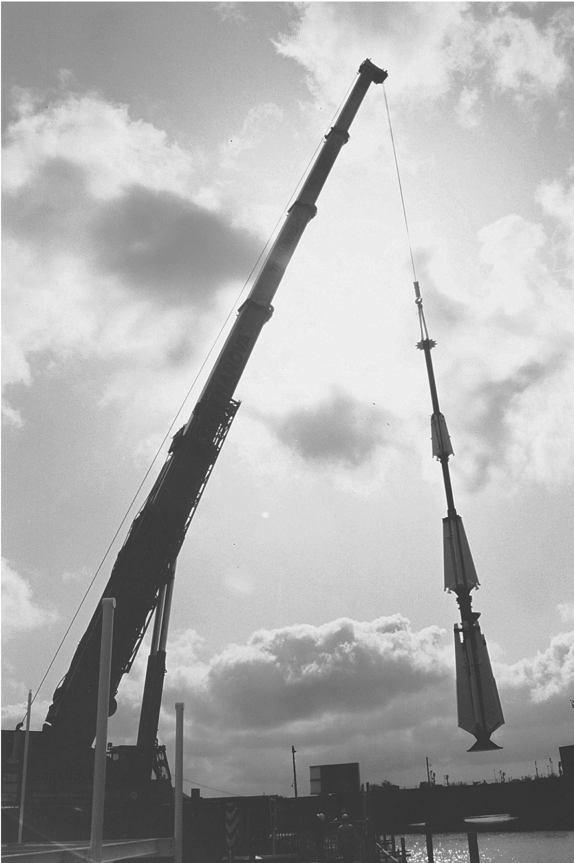
Fig. 7.6 Deployment of the mast.
