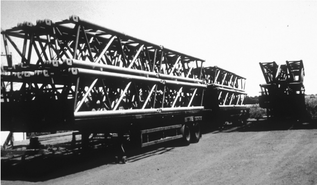
Fig. 9.2 MEC Arena, Buro Happold, 1990. The structure is transported on articulated lorry trailers.
