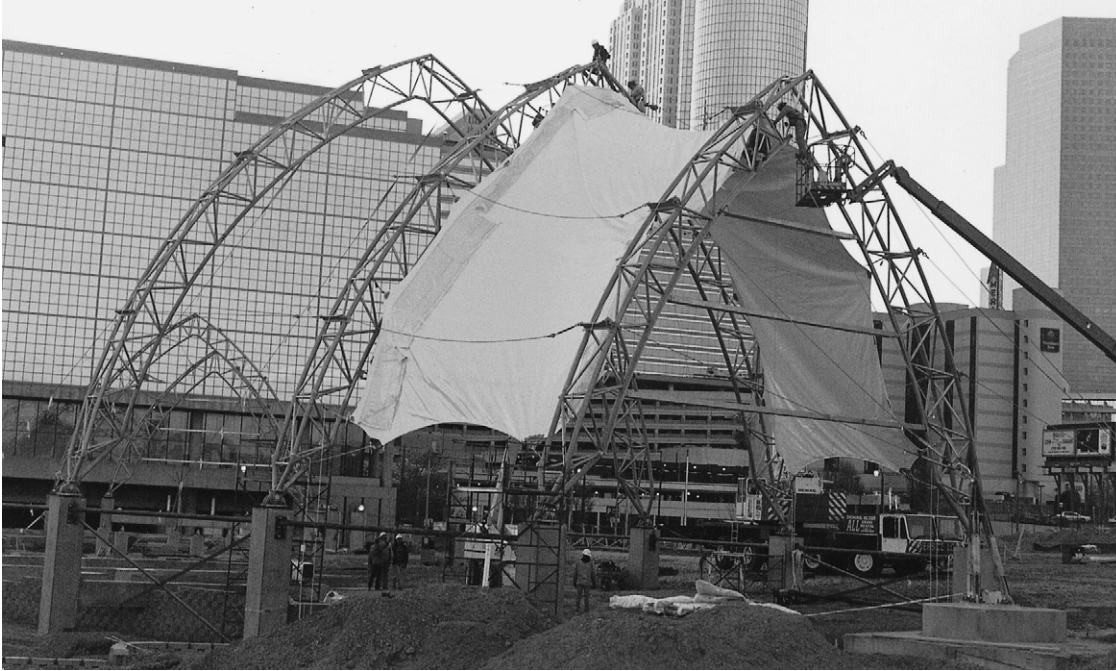
Fig. 12.28 AT&T membrane being deployed.
