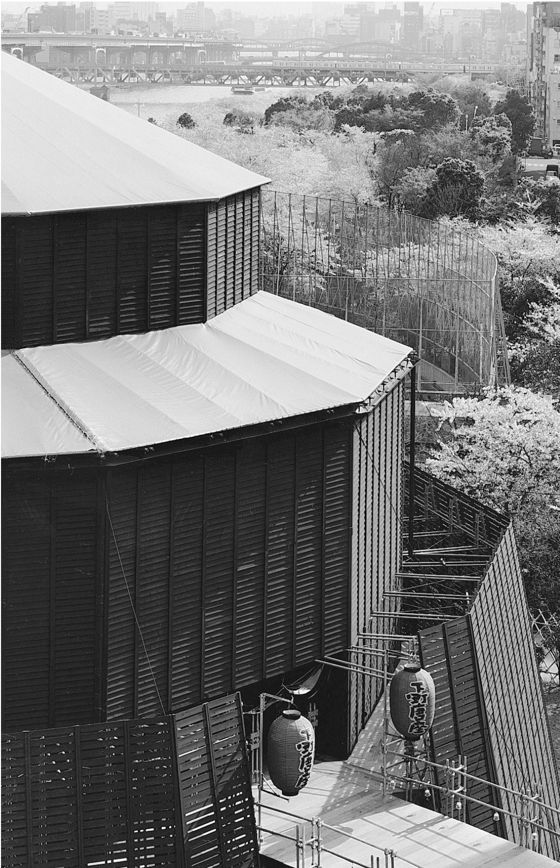
Fig. 2.8 Completed building showing the tension membrane roof and boarded cladding.
