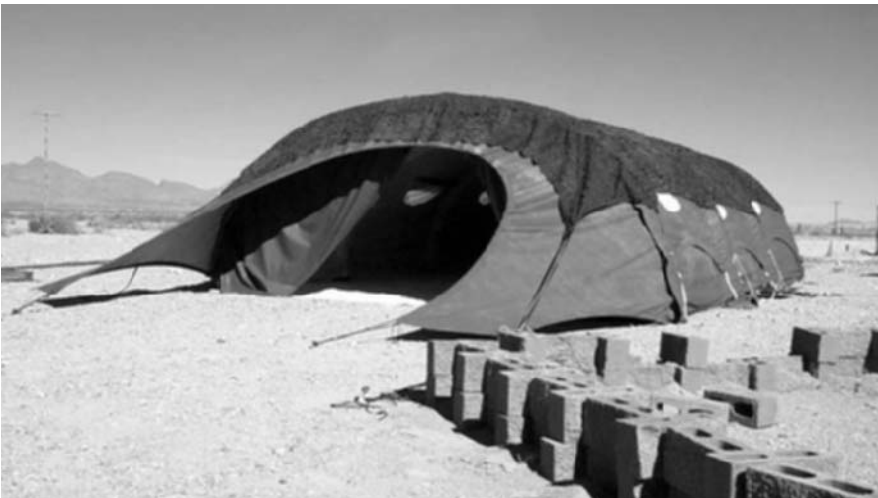
Fig. 12.24 The Small Air Force Shelter (SAFS), an air-beam supported portable shelter built by Vertigo Inc.
