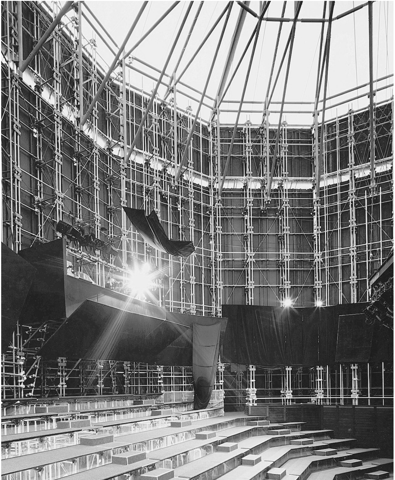
Fig. 2.9 Interior. Carpet covered bleacher-type seating. The dark fabric covered panels conceal access gangways and production equipment.
