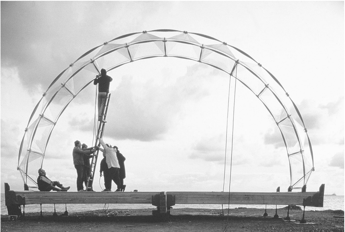
Fig. 1.9 Mounting of a prototype arch for Renzo Piano's IBM pavilion.
