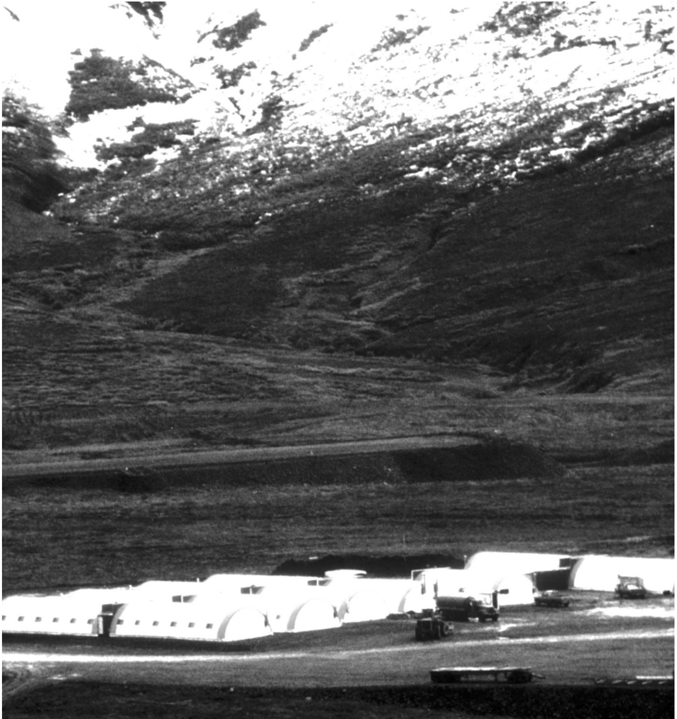
Fig. 16.4 A remote base created primarily from the 'Series '4' shelter system. All units are linked with enclosed corridors.
