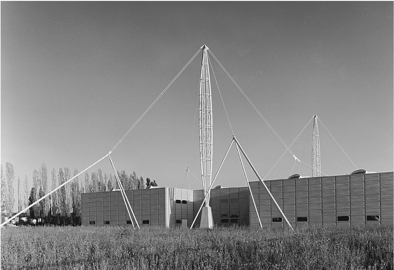
Fig. 8.8 The first phase of the building was built with two masts and one and a half courtyards complete.
