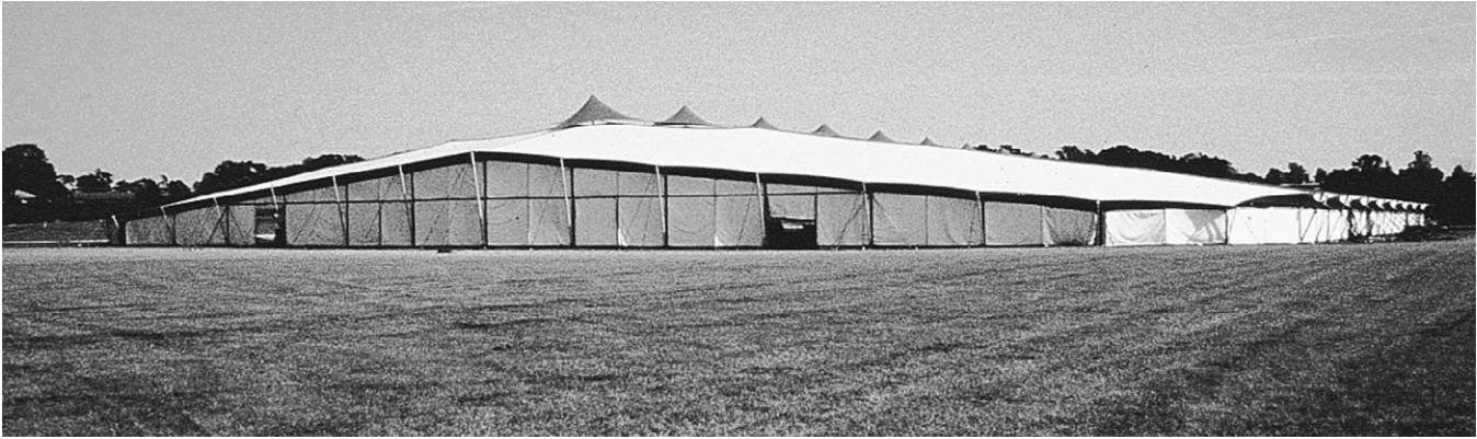
Fig. 9.14 External view. The building has a very low profile despite the larger spans involved.
