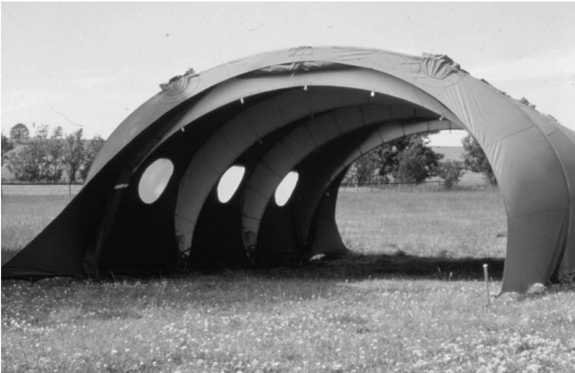
Figure I.31 MOD deployable shelter by J.T. Inglis and the Lightweight Structures Unit at the University of Dundee.
