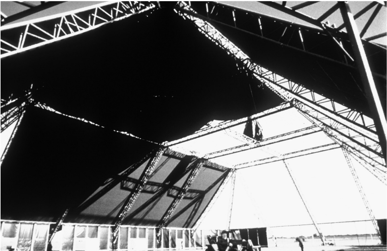
Fig. 9.5 A modular partition system is used for the ground level perimeter cladding.
