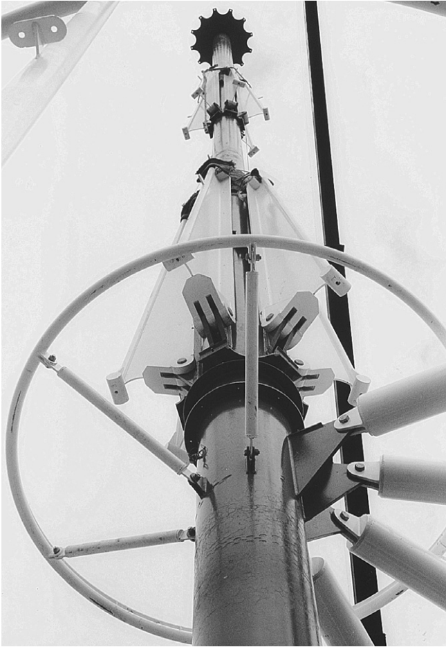
Fig. 7.7 View from the base of the mast with the main horizontal roof beams deployed. The platform beams are still in their travelling position against the mast.
