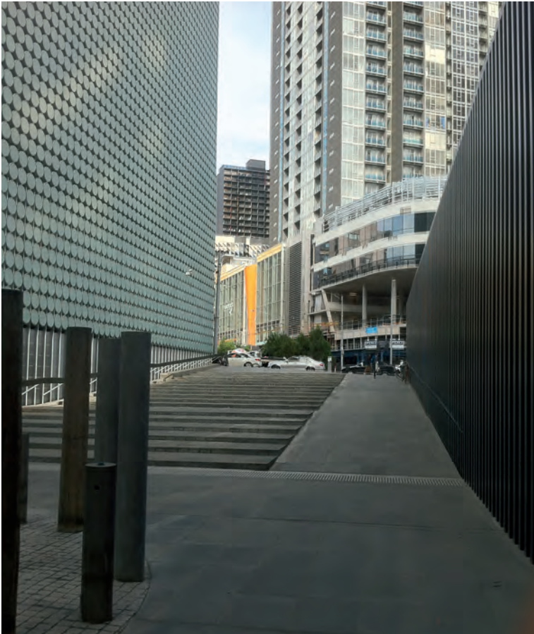
Sean Godsell Architects, RMIT Design Hub, Melbourne, 2012 The Design Hub creates a critique of the less considered buildings around it.
