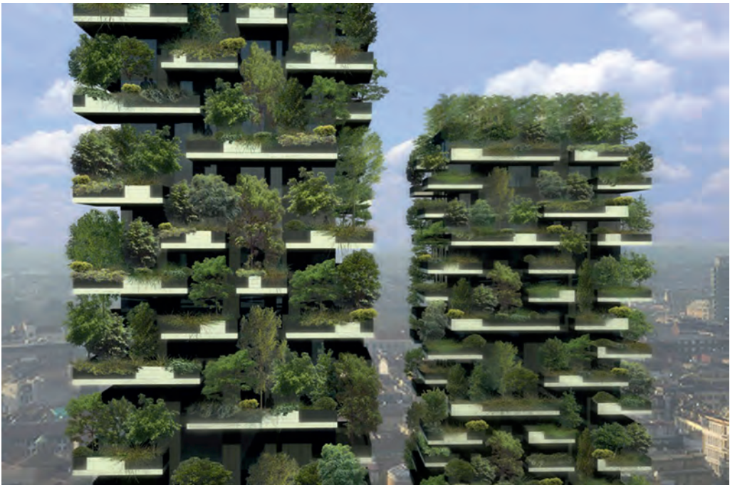
Companion to The Oliv , Singapore: Stefano Boeri, rendering of Bosco Verticale , Milan, 2014 Trees grown off site during the period of construction were craned into position when the building was completed.
