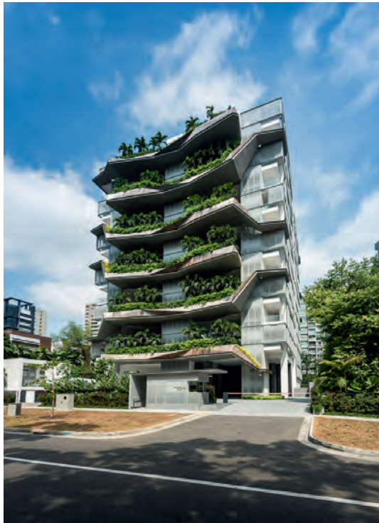
W Architects, The Oliv, Singapore, 2013 View of the apartment building with its sky terraces. Note how these kick up and down at the right-hand side.
