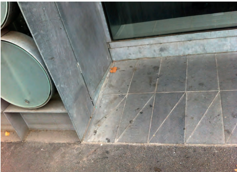
Sean Godsell Architects, RMIT Design Hub, Melbourne, 2012 The subtle accommodation of the entry threshold to the slope to the left is achieved with triangulated pavers.
