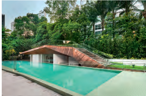
W Architects, The Oliv , Singapore, 2013 A fragment of the twisting timber-clad sky terrace is used to make the roof and roof deck over the pool room and gym.
