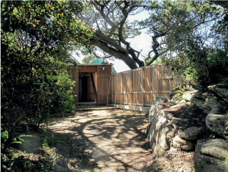
Feary + Heron, Plant Room, Eagle's Nest, Zennor, Cornwall, England, ongoing The Plant Room with its slanting column seen from the sheltered courtyard, one of the rooms that the boulders delineate.
