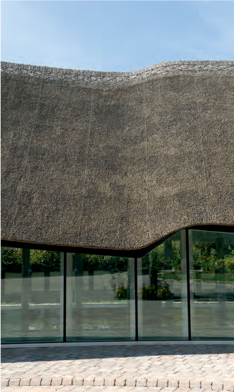
Ushida Findlay, Poolhouse 2, Home Counties, England, 2009 Poolhouse 2 shows Ushida Findlay using thatch as a material that lends itself to the forms that emerge from algorithmic designing.
