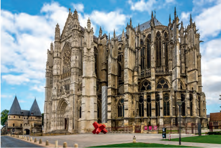
The Cathedral of Saint Peter of Beauvais, Beauvais, France, 1284 At 48 metres (157 feet) high, this was to be the tallest cathedral in France. The collapse of some bays in the choir during construction in 1284 ended this ambition and terminated the search for height in Gothic architecture.
