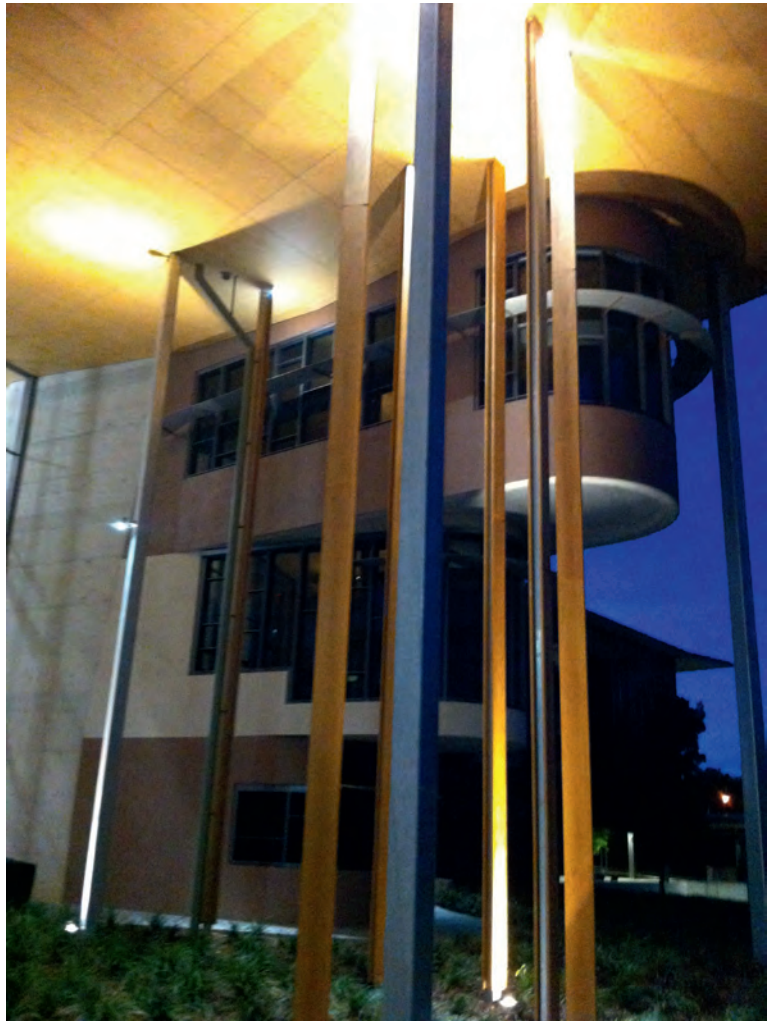
CRAB studio, Abedian School of Architecture, Robina, Queensland, Australia, 2014 Mushroom plate roofs swell out to shelter the entry from sun and tropical rainstorms.
