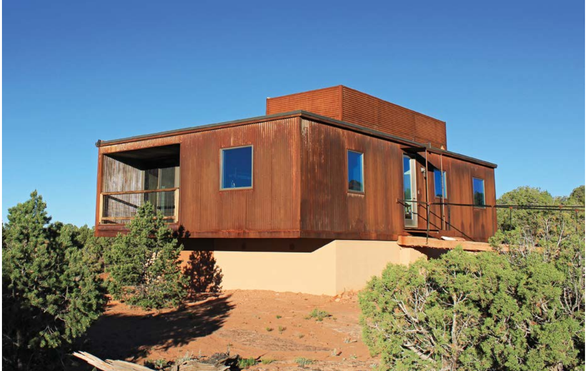
The solar thermal panels on the roof are covered, as mandated by local guidelines.
