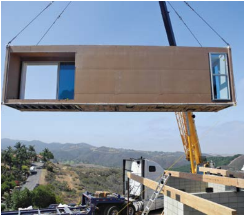
TOP: The modules under construction in the factory.
