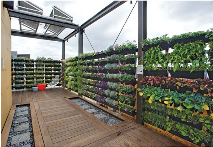
The recycled steel post and beams provide a structure for the house, PV panels, and a vertical garden.
