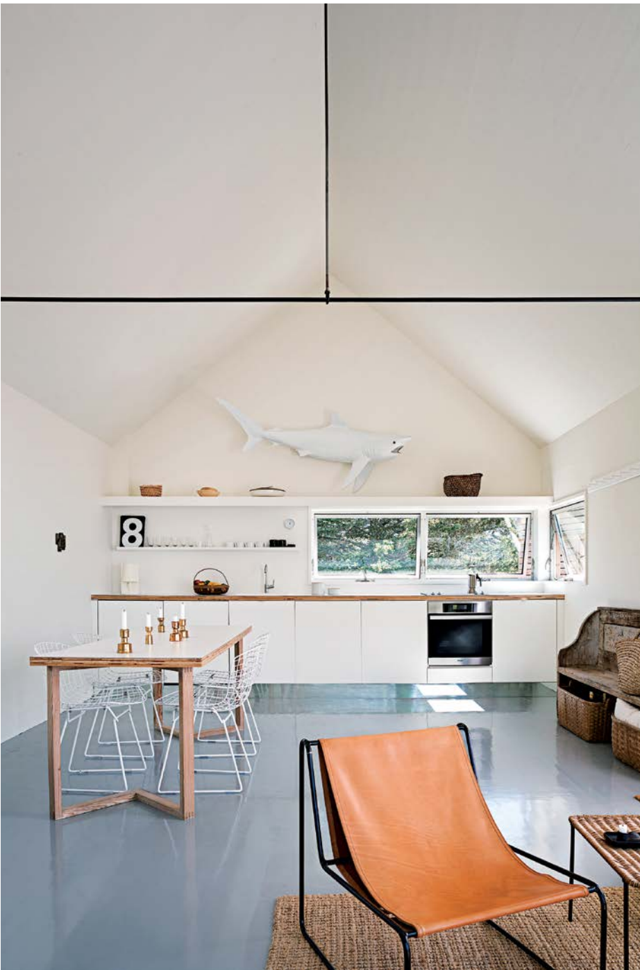
The flooring in the main part of the cabin is CLT, which was sanded and painted. The kitchen flooring is laminate.
