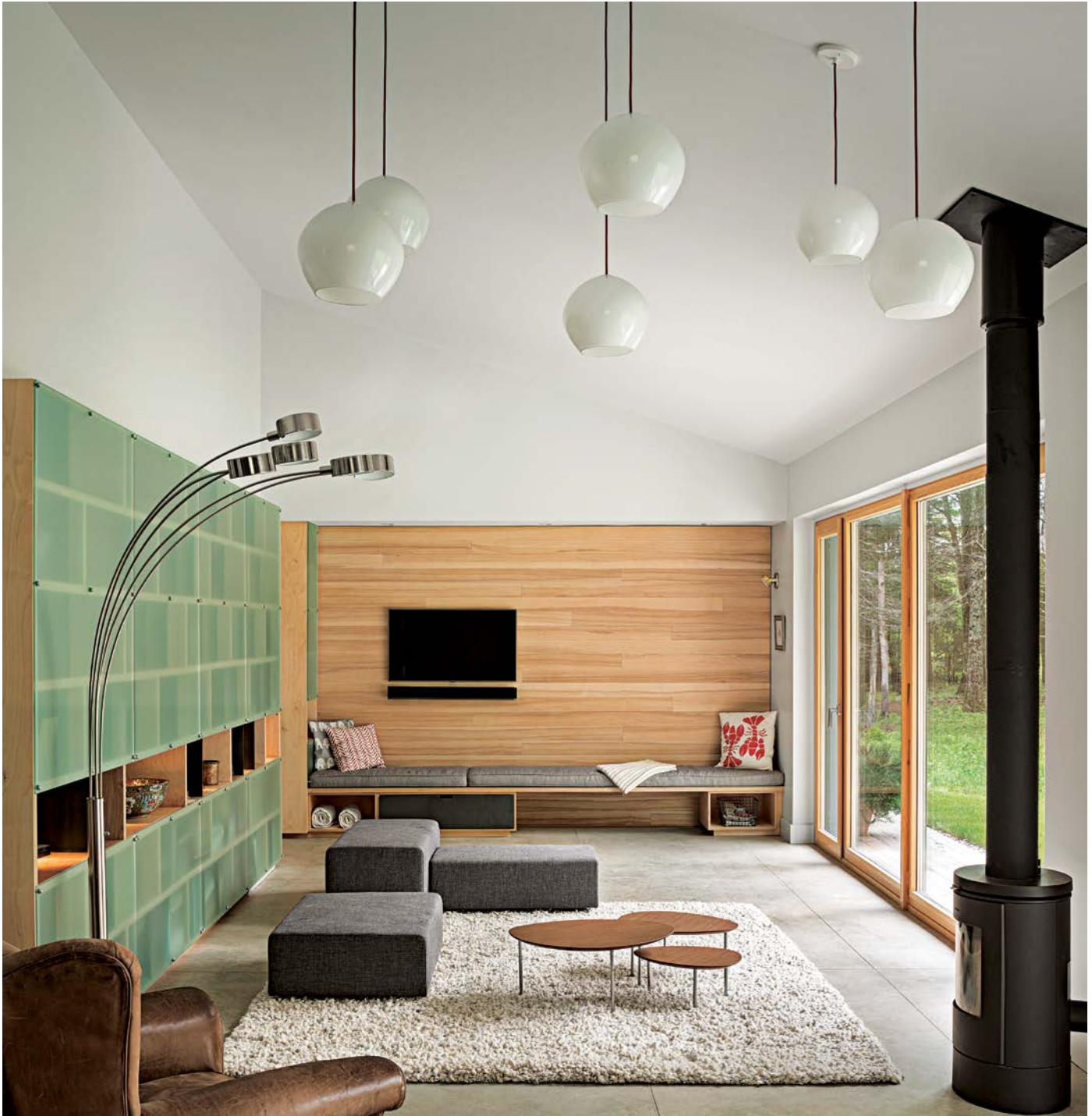
In the living room, large expanses of glass and a high cathedral ceiling create a generous sense of space for the home's small footprint. Crafted of clear-finished Baltic birch plywood with mill-finished steel dividers, the bookcase has integrated lighting in the display shelf. Its acid-etched glass is backlit from the hallway at night.
