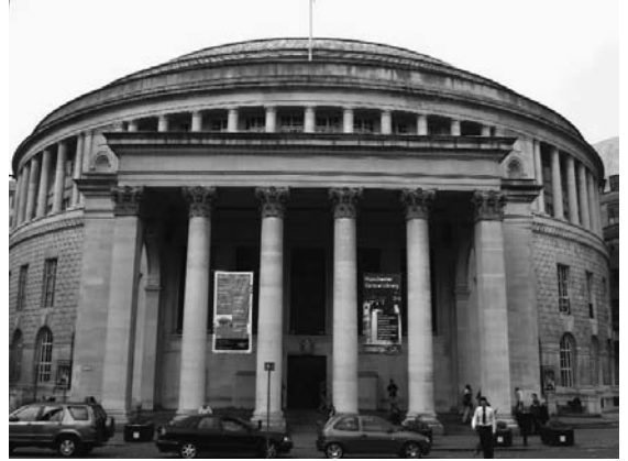
Figure 11.3 Manchester Central Library. Photograph by author.
