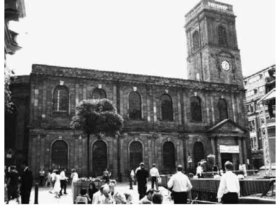
Figure 11.1 St Ann's Church, Manchester. Photograph by author.
