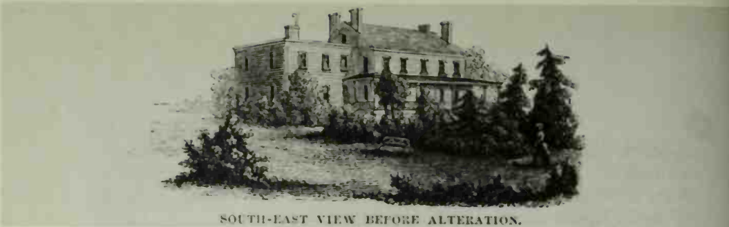
SOUTH-EAST VIEW BEFORE ALTERATION.
