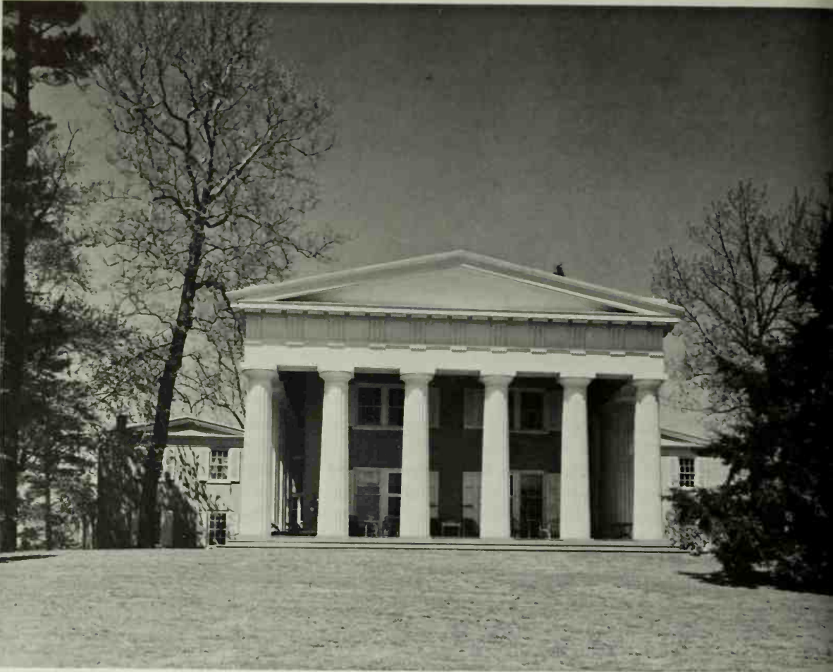
Andalusia, Andalusia Pa. (Photograph, Wayne Andrews)
