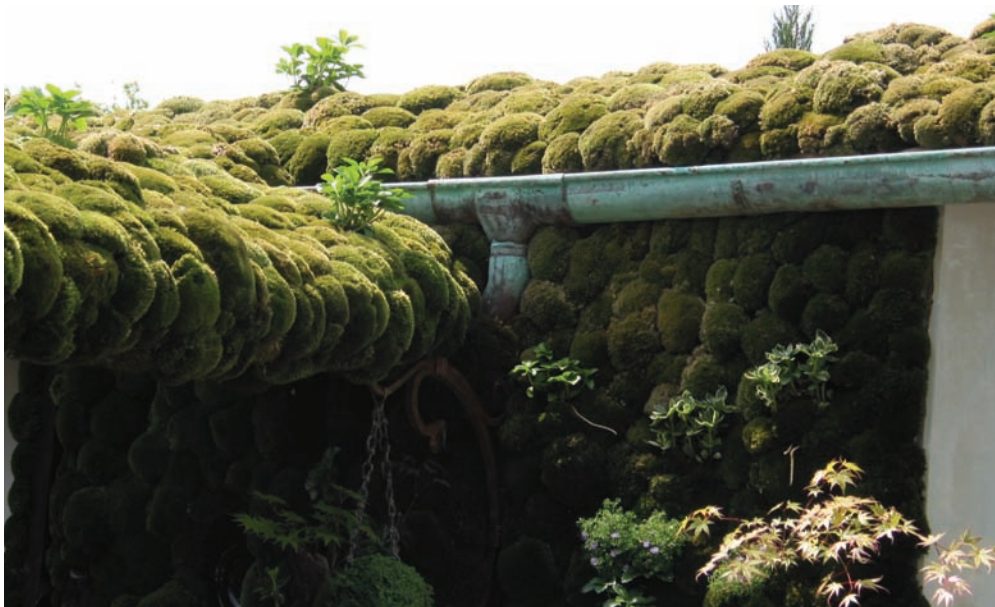
This Japanese-style moss roof will only succeed in wetter climates or in shade. Photo by Wendy Allen
