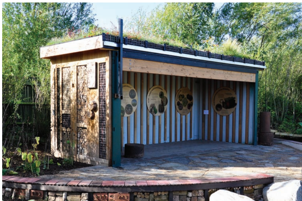
A green-roofed container building in the Rain Garden at The London Wetland Centre. Designed and built by Green Roof Shelters. Photo by Nigel Dunnett
