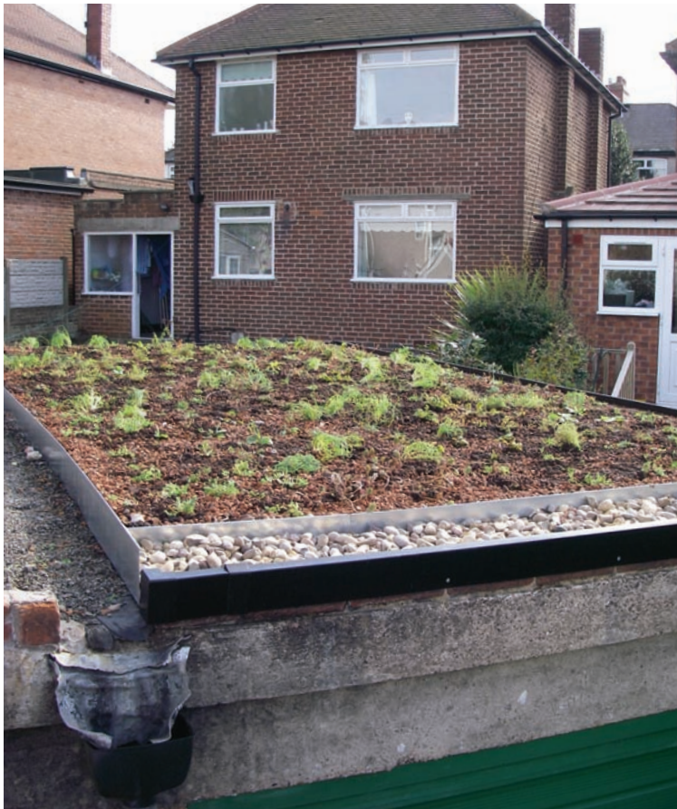
Left: A pebble edge leads to the existing roof drainage point. Photo by Green Estate Ltd.
