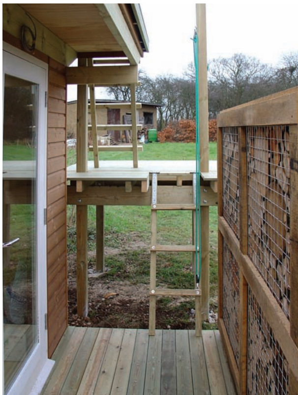
The thin screen to the building contains log sections in wire mesh panels. Photo by Jane Sebire
