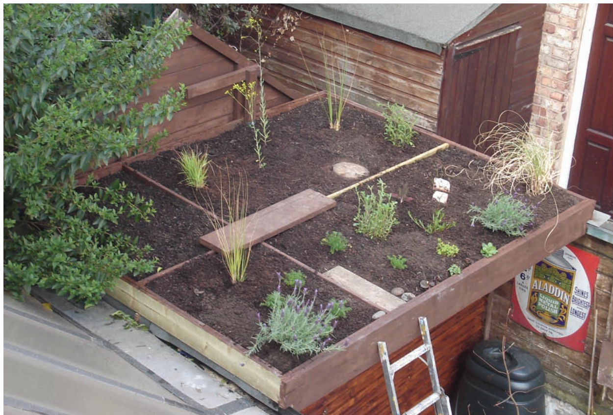
The roof on the shed being planted. Photo by Helene Rudlin
