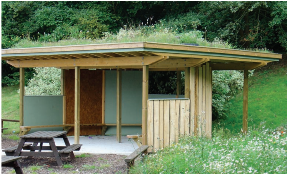
The green roof is a great educational resource and blends well with the building's surroundings. Photo by John Little
