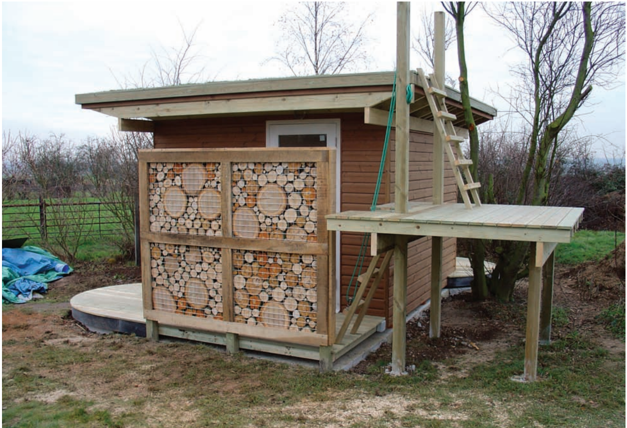
The completed building, with external access and drawbridge to roof level. Photo by John Little
