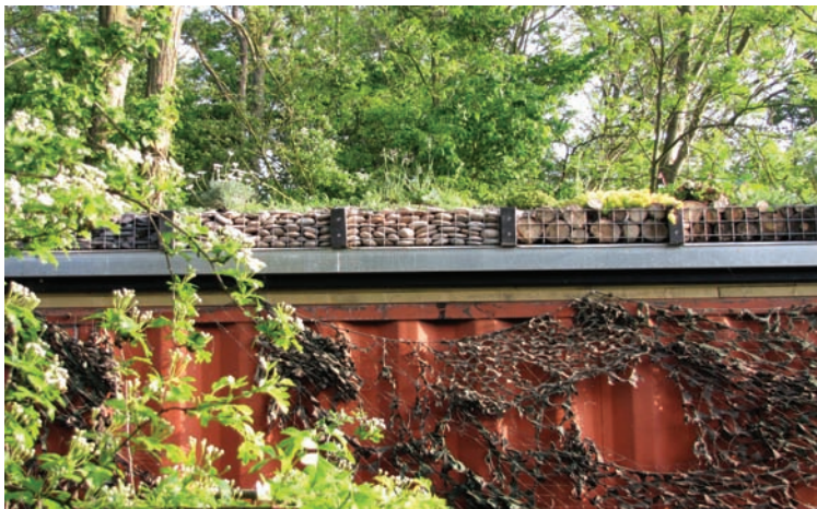
Left: An edging of pebbles and log sections on this green roof on a converted shipping container retains substrate, aids drainage, provides invertebrate habitat, and is an attractive feature in itself. Photo by John Little
