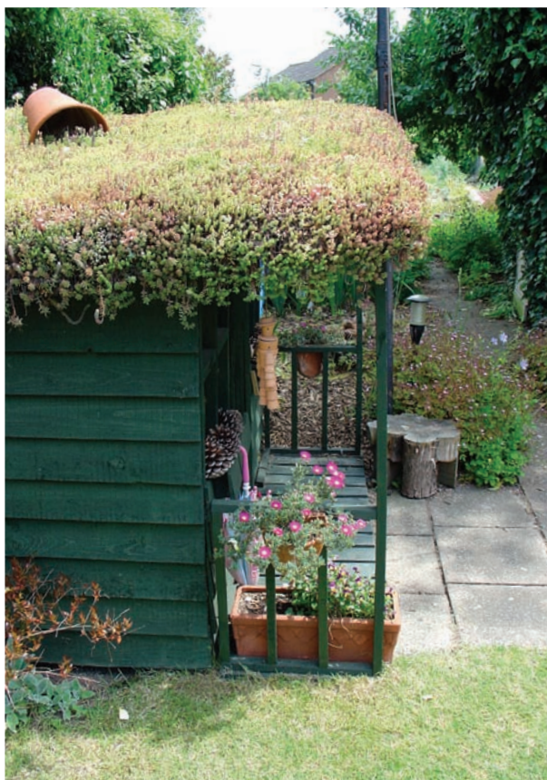
The surplus sedum blanket from the house roof was used to make a green roof on the children's playhouse. Photo by Jane Sebire
