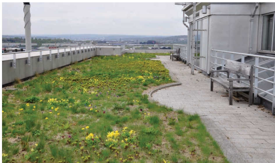
A roof terrace which supports green roof planting, rather than plants in containers or raised beds. Photo by Nigel Dunnett
