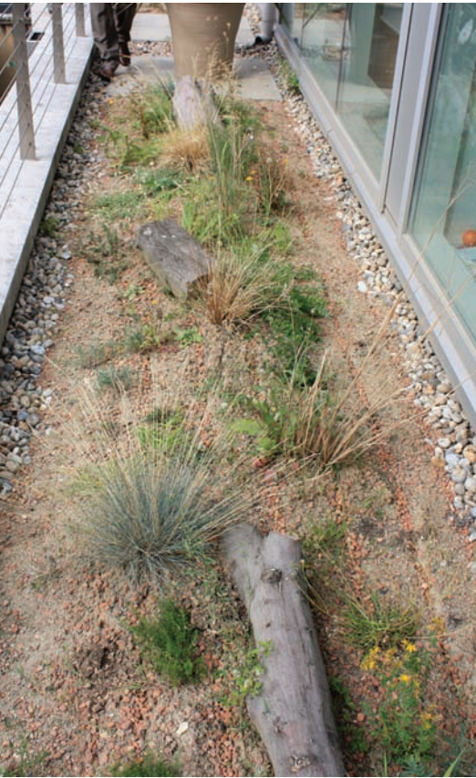
Even the smallest of spaces are suitable for greening. Here a green roof for wildlife is installed on an apartment balcony. Photo by Dusty Gedge
