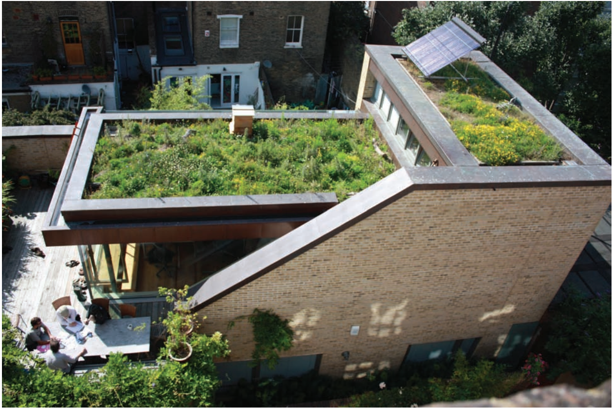
These green roofs are inaccessible and planted to attract wildlife. Photo by Dusty Gedge
