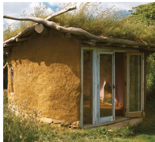
The roof structure on this yoga studio in Cornwall, United Kingdom, consists of oak logs. Local soil and turf was used to make the grass roof. Photos by Katy Bryce
