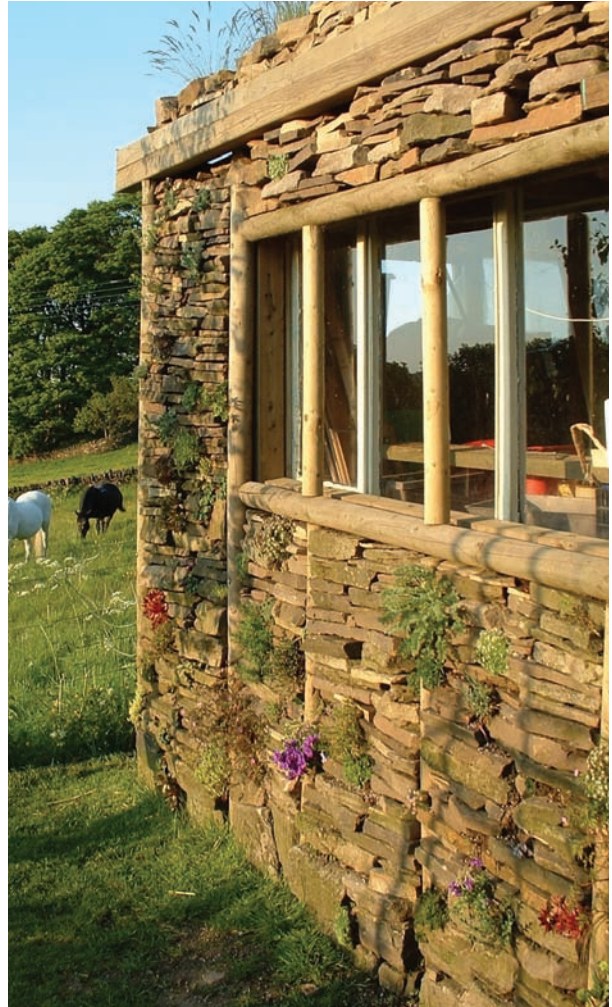
The living wall of Nigel Dunnett's shed contains many alpinas, planted into gaps in the dry stone. Photo by Nigel Dunnett
