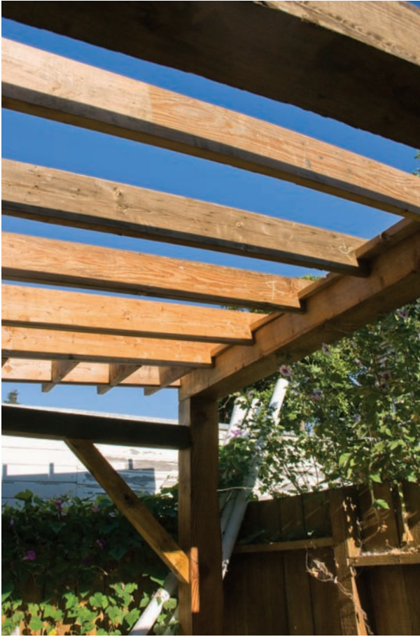
Above: The underlying structure of the roof. Photo by Jennifer Natali
