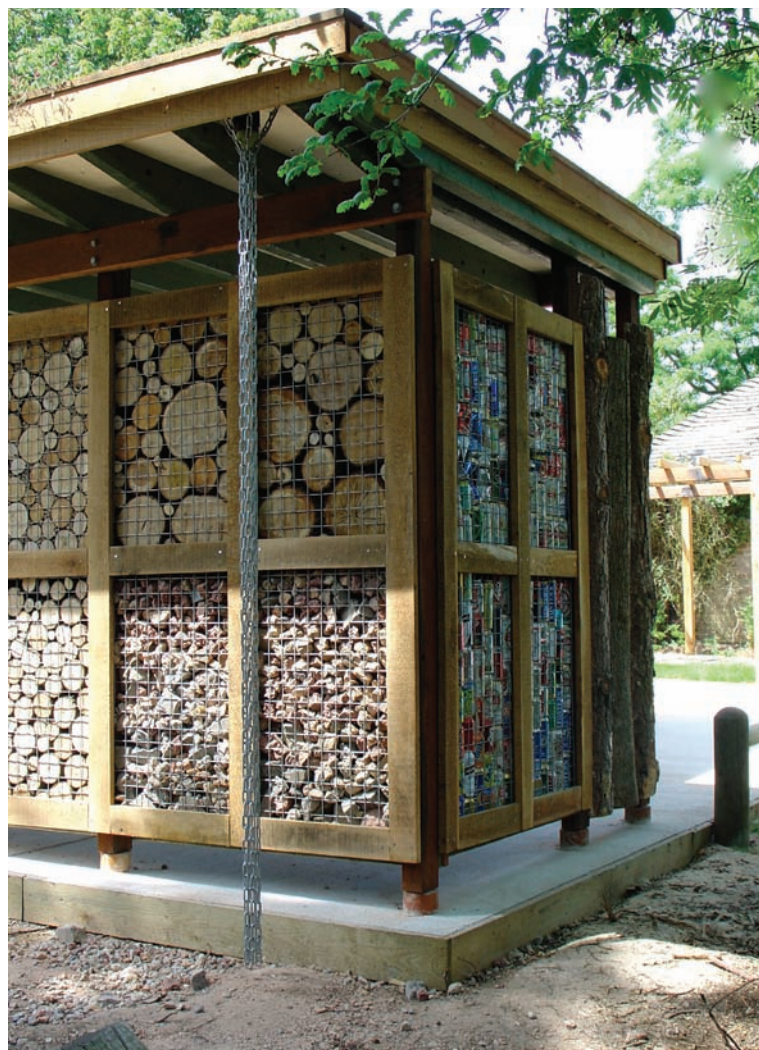
The rain chain directs runoff water to ground level. Photo by John Little
