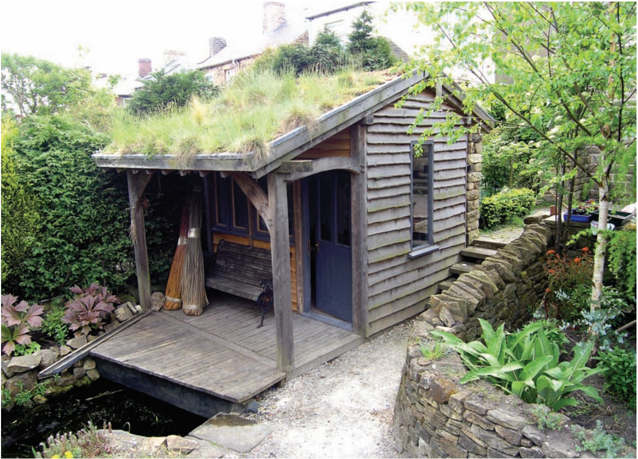
The green roof after seven years. Water drains from the roof into the pond. Photo by Andy Clayden
