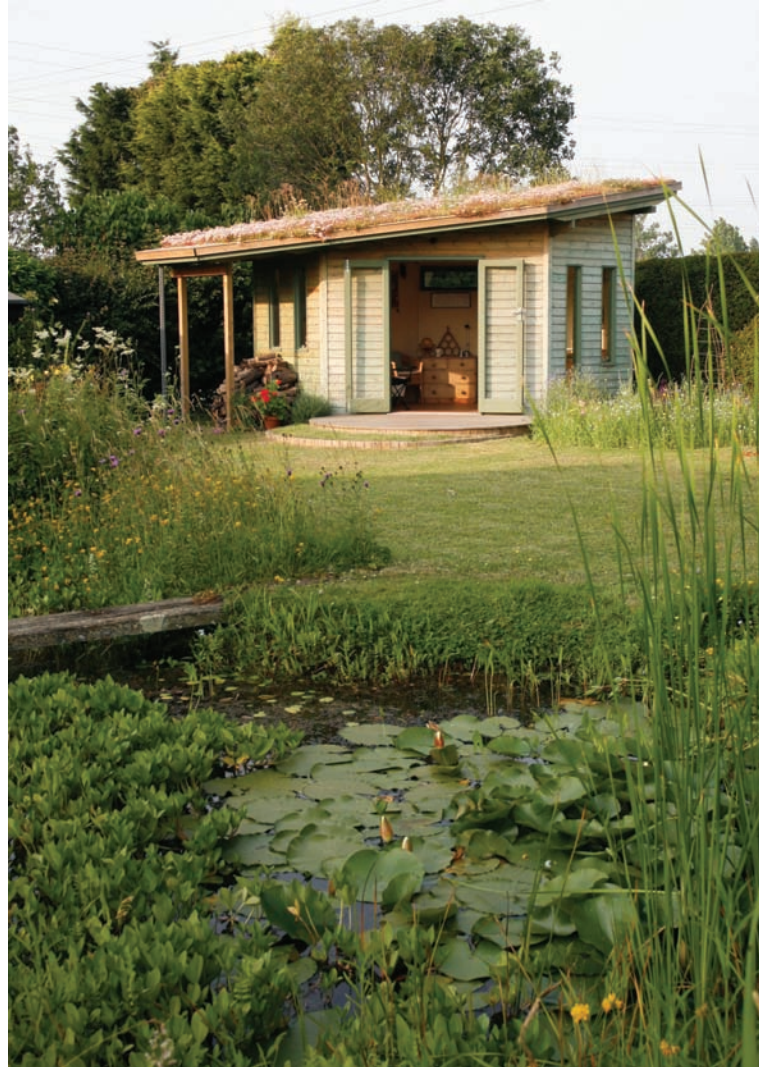
The green roof fits beautifully into the natural garden. Photo by Jane Sebire
