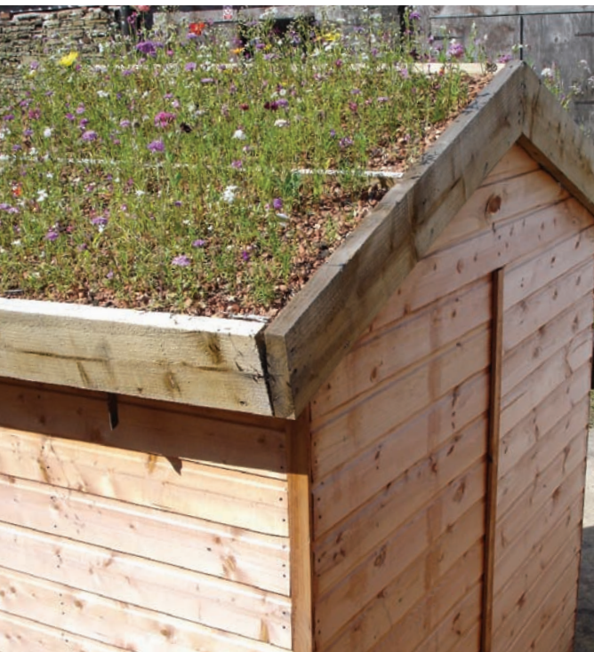
The completed shed, with green roof tray added on top. Photo by Green Estate Ltd.
