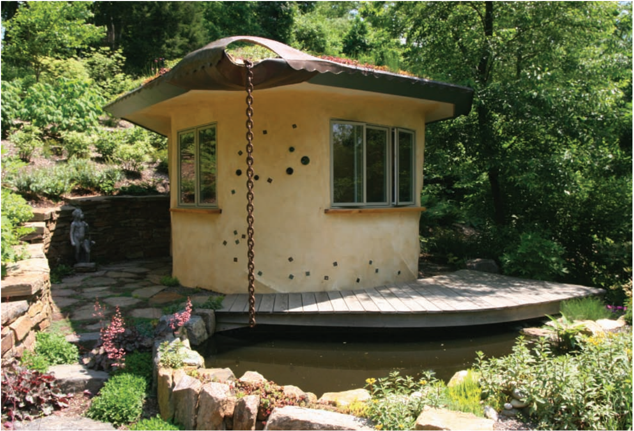
A chain carries runoff water from the roof into a reflecting pool below. Photo by Ed Snodgrass
