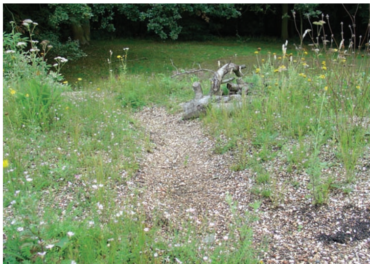
The roof has a varied topography, and old logs add to the wildlife value. Photo by John Little
