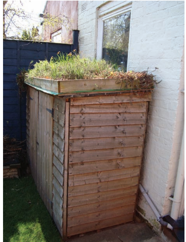
The completed shelter. Photo by Dan Cornwell
