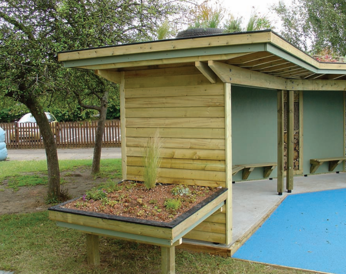
Left: A miniature green roof at children's level shows what is on the classroom roof. Photo by John Little
