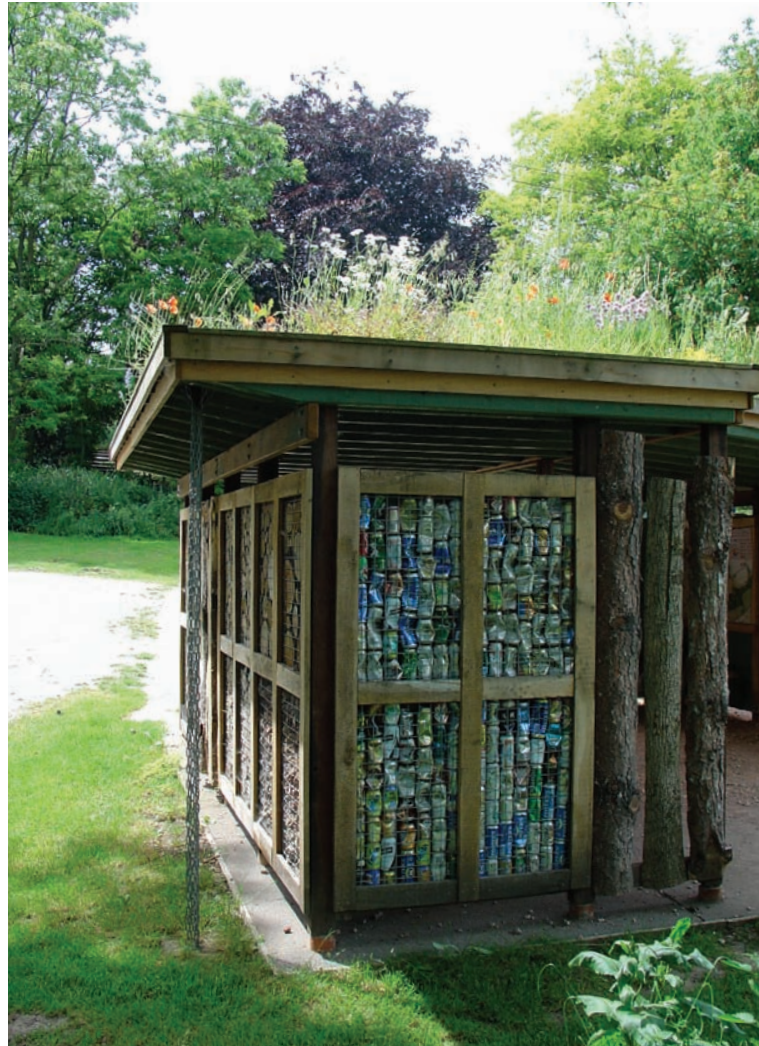
The building houses recycling facilities, and the wall panels contain examples of the items that can be recycled there. Photo by John Little
