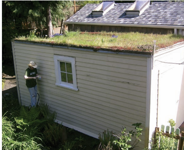
The ecoroof on the garage. Photo by Tom Liptan
