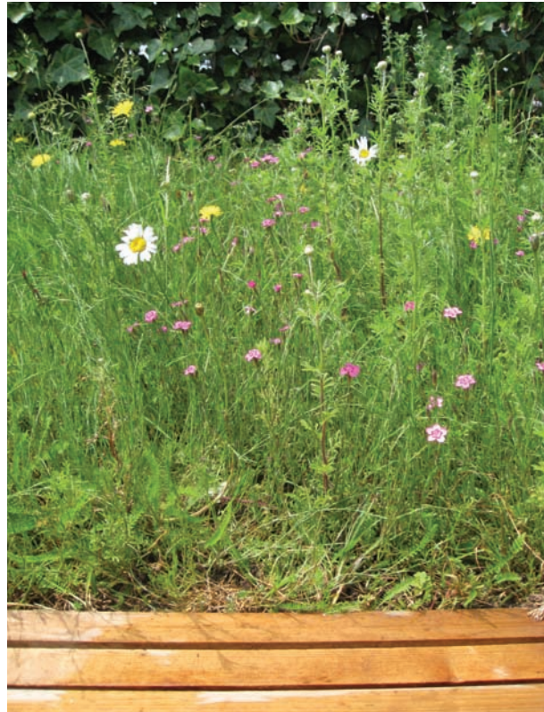
The vegetation was installed using a species-rich green roof mat produced by Lindum Turf. Photo by Wendy Allen
