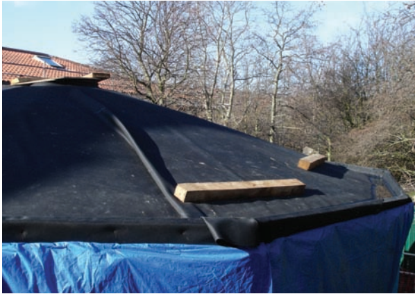
Above: Waterproofing a round conical roof with a flexible liner on a building at a school in Sheffield, United Kingdom. Photo by Green Estate Ltd.
