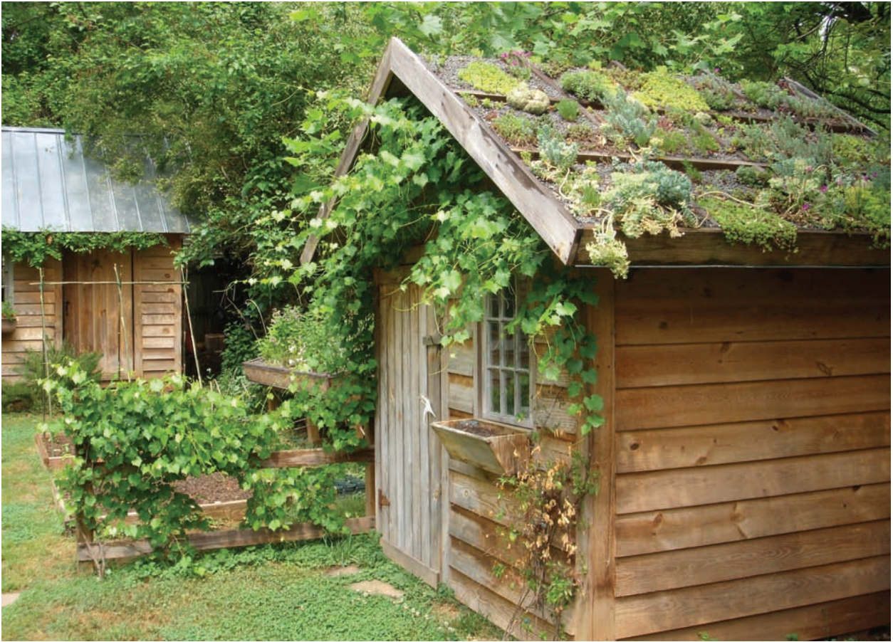
The completed shed. Photo by Emilio Ancaya, Living Roofs, Inc.
