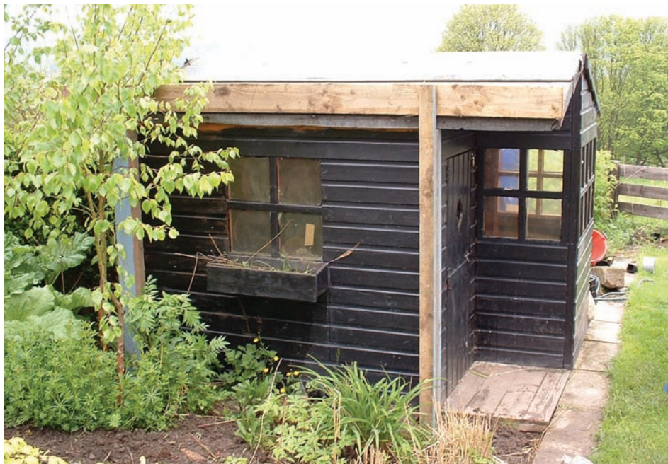
Left: A timber edge is held in place with external supports. Photo by Nigel Dunnett
