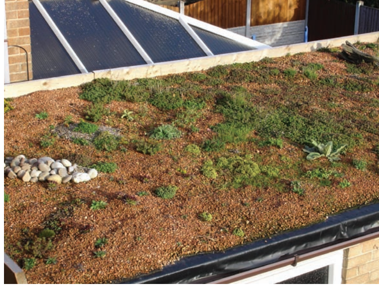
After plant establishment, the deeper areas can easily be seen as they have far better vegetation growth. Photo by Jeff Sorrill
