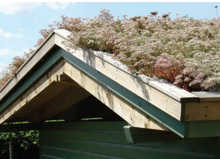
Sedum album flowering on the bicycle shelter roof. Photo by John Little
