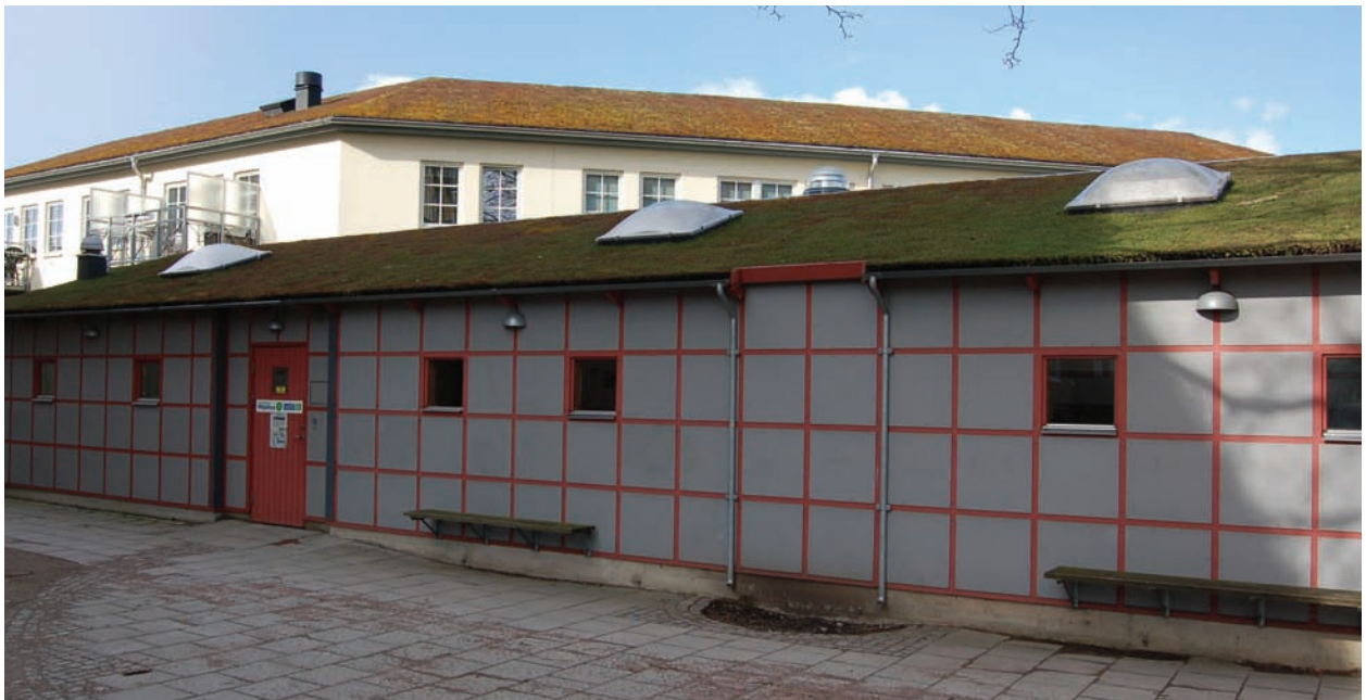
Green roofs on houses and storage sheds created with a pregrown sedum mat. Photo by Nigel Dunnett
