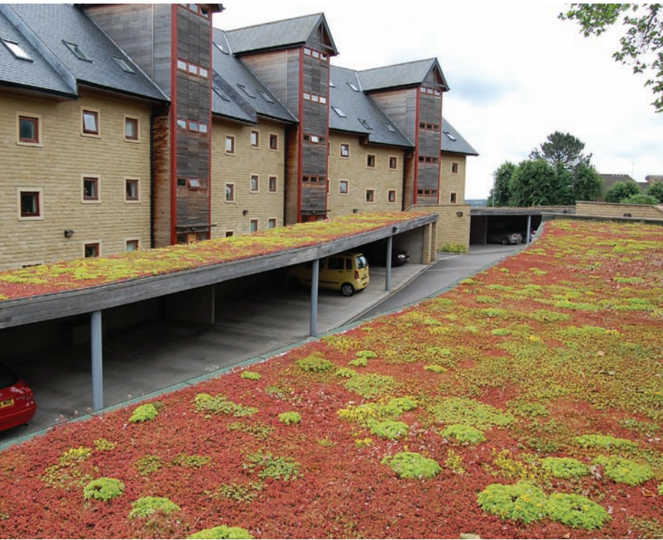
Left: Green-roofed garages for an apartment block in Sheffield, United Kingdom. Photo by Nigel Dunnett
