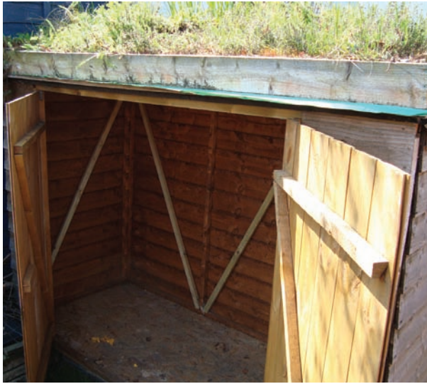
The shed is internally strengthened with batons. Photo by Dan Cornwell
