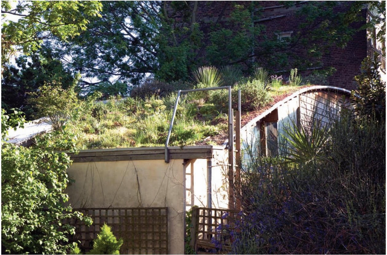
The green roof is on a curved sloping roof, which creates a range of moisture regimes from top to bottom. Photo by Jane Sebire
