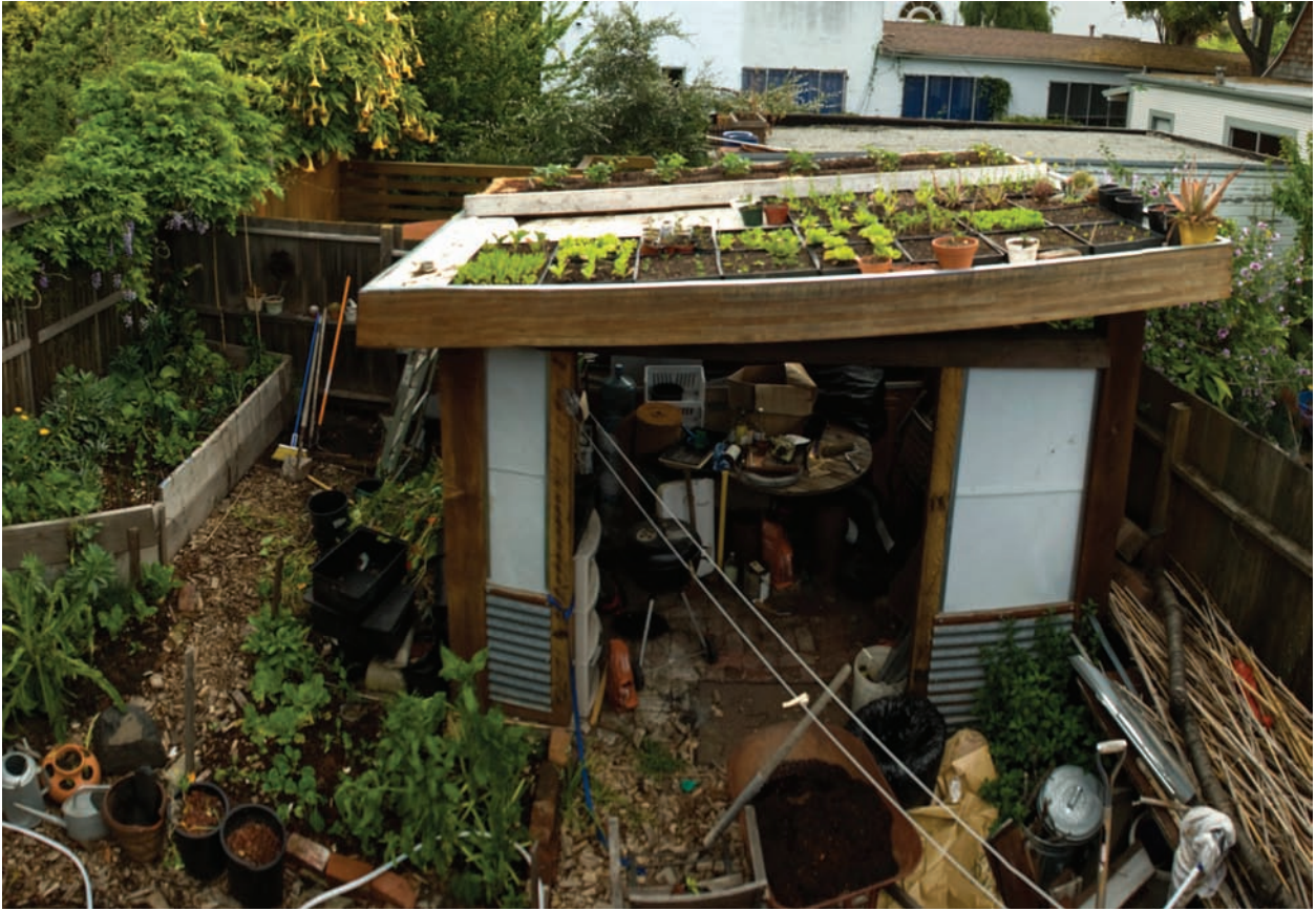
The first trays were placed on drainage material, and later trays went directly onto the roof. Photo by Jennifer Natali
