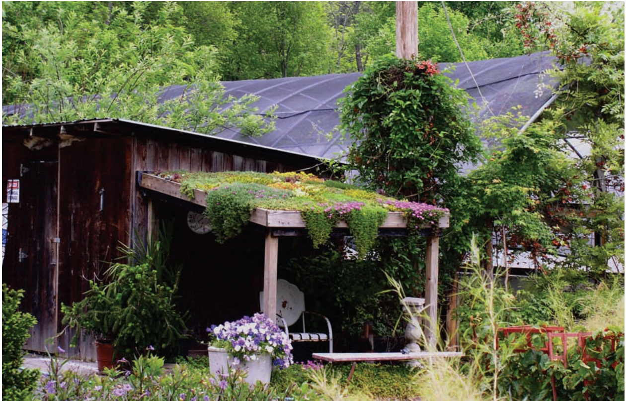
The green roof is on a simple lean-to structure fixed to an existing building. Photo by Ed Snodgrass
