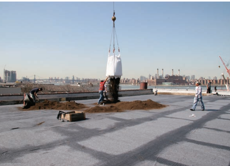
Substrate being lifted to the prepared roof. Photo by Annie Novak
