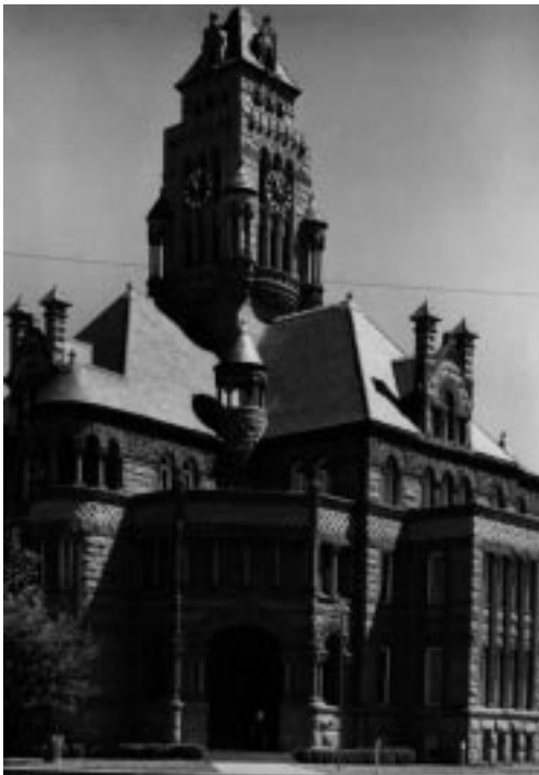
ELLIS COUNTY COURT HOUSE (1894–97) Main Street (US 287) Waxahachie, Texas
