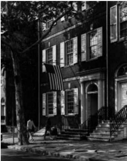
POWEL HOUSE (1765–69) 244 South 3rd Street Philadelphia, Pennsylvania
