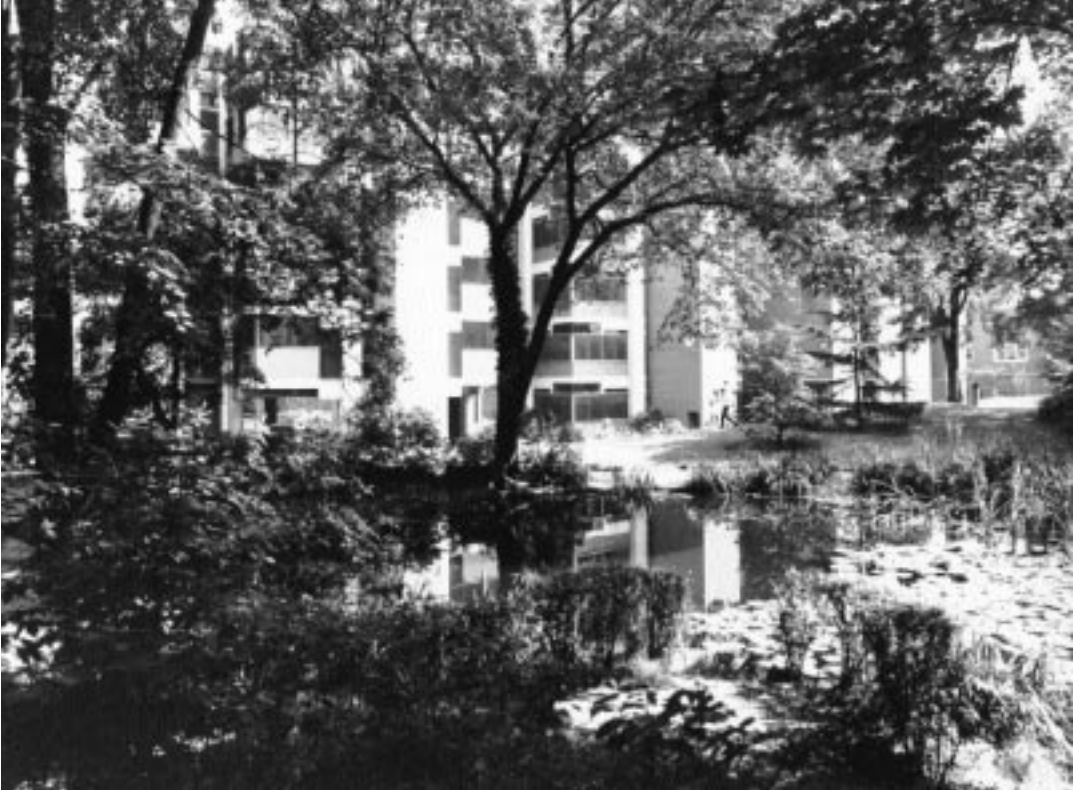
ALFRED NEWTON RICHARDS MEDICAL RESEARCH BUILDING (1957–61) GODDARD BIOLOGY LABORATORY (1962–64) University of Pennsylvania 3700 Hamilton Walk, next to Medical School Philadelphia, Pennsylvania
