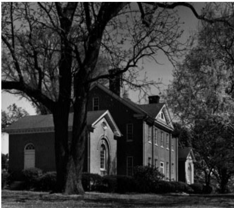
MOUNT CLARE (c. 1763/1906) 1500 Washington Boulevard at Monroe Street (US 1) Carroll Park Baltimore, Maryland
