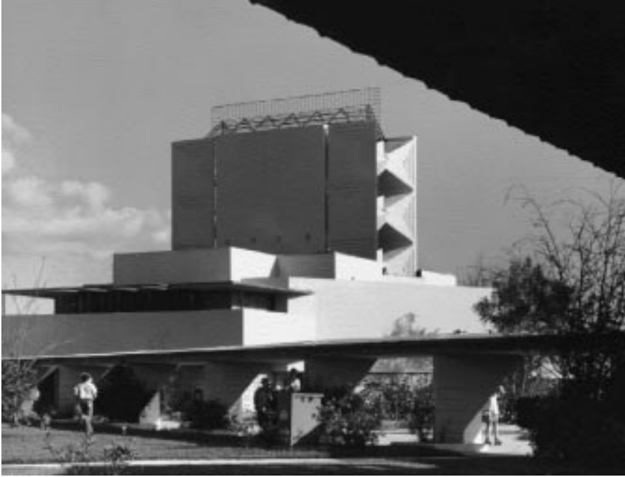
FLORIDA SOUTHERN COLLEGE (1938–58) Johnson Avenue and McDonald Street Lakeland, Florida
