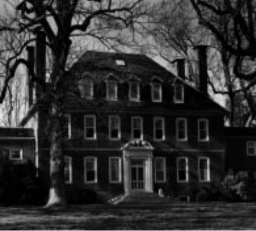
WESTOVER (c. 1730–34) 7000 Westover Road Charles City, Virginia
