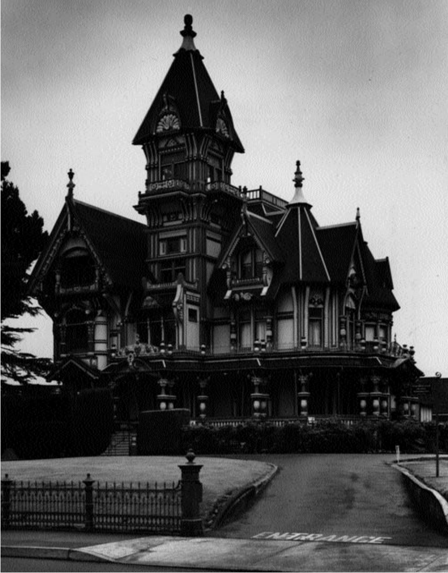
CARSON MANSION (1884–86) 143 M Street at 2nd Street Eureka, California
