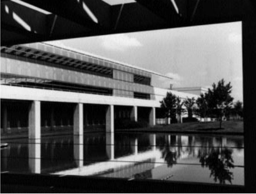
CONOCO HEADQUARTERS (1984–86) 600 North Dairy Road Houston, Texas
