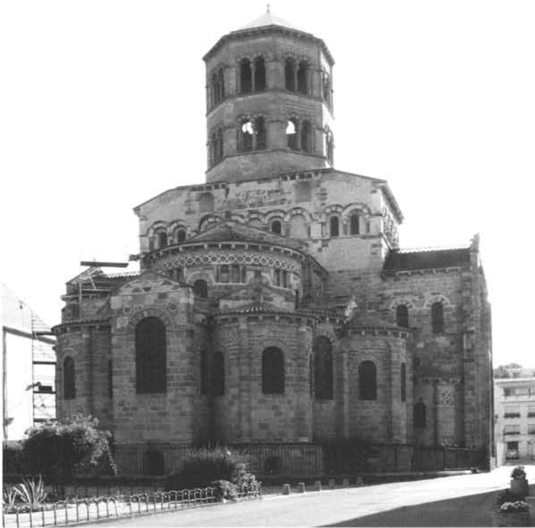
St. Austremoine in Issoire, probably built around 1130–1150, is an example of the unique architectural tradition of the Auvergne, a region on France's central plateau.
