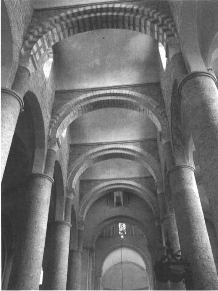
Saint Philibert at Tournus in Burgundy (late 900s through early 1100s) is nearly unique in its use of transverse barrel vaults, making it much lighter than most Romanesque churches. Photo by Randy Seitsinger.
